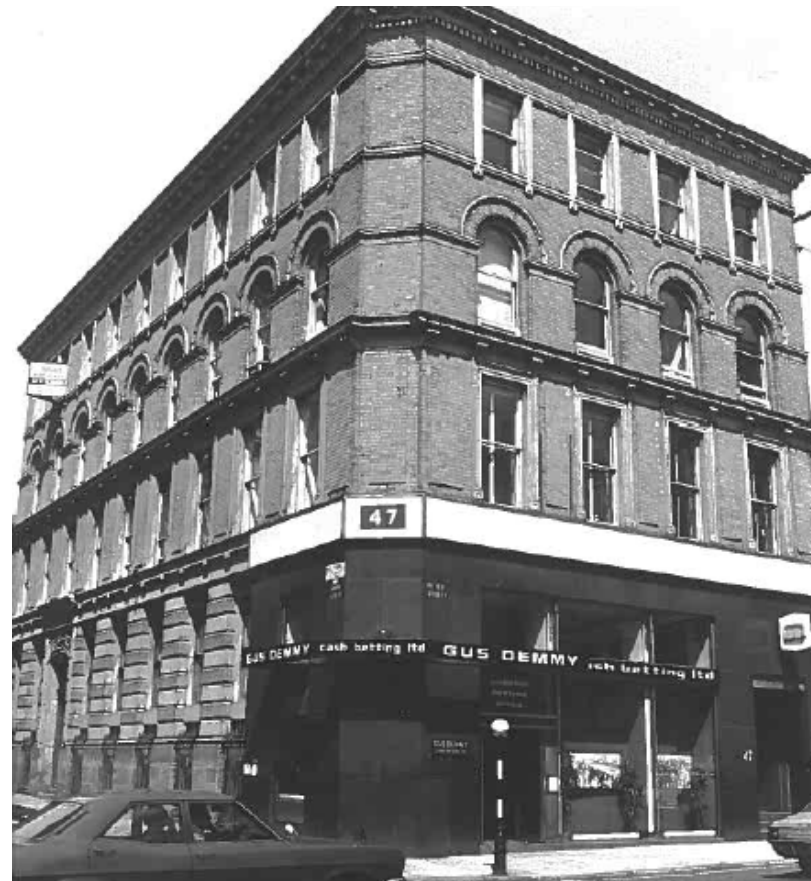
3. 1976 - GRANITE OVERCLADDING TO GROUND FLOOR ELEVATION
