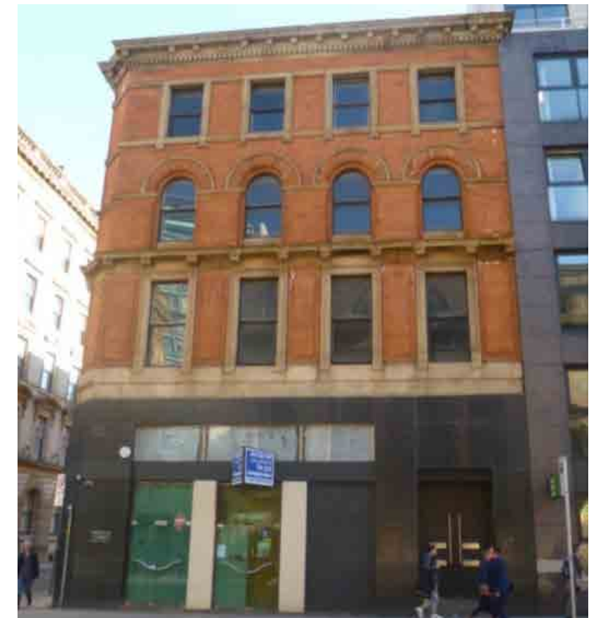
4. 2014 - ELEVATIONAL ALTERATIONS FOLLOWING A FIRE IN 2012
