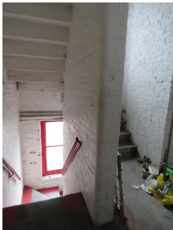
Figure 21 – The stone staircase, accessed originally from the eastern entrance on Addington Street only.
