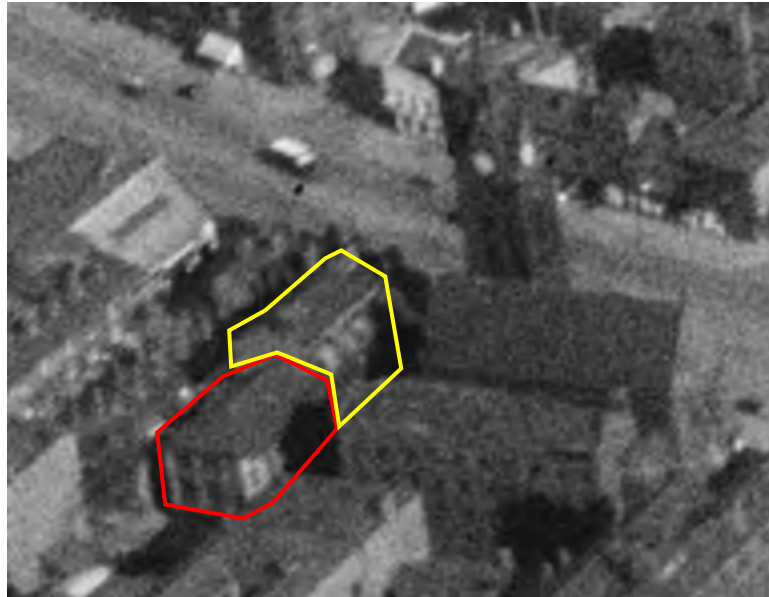
Figure 16 – An aerial view of the Site in 1937, showing No. 14 (left) 3 years before the building was substantially damaged by a German bombing raid. This is the only known photograph showing the original two-storeys of No. 14 Addington Street (outlined red). To the right can be seen No. 4 (outlined yellow).
