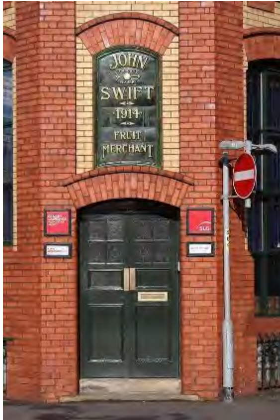
Figure 14 - No. 19 Mason Street
