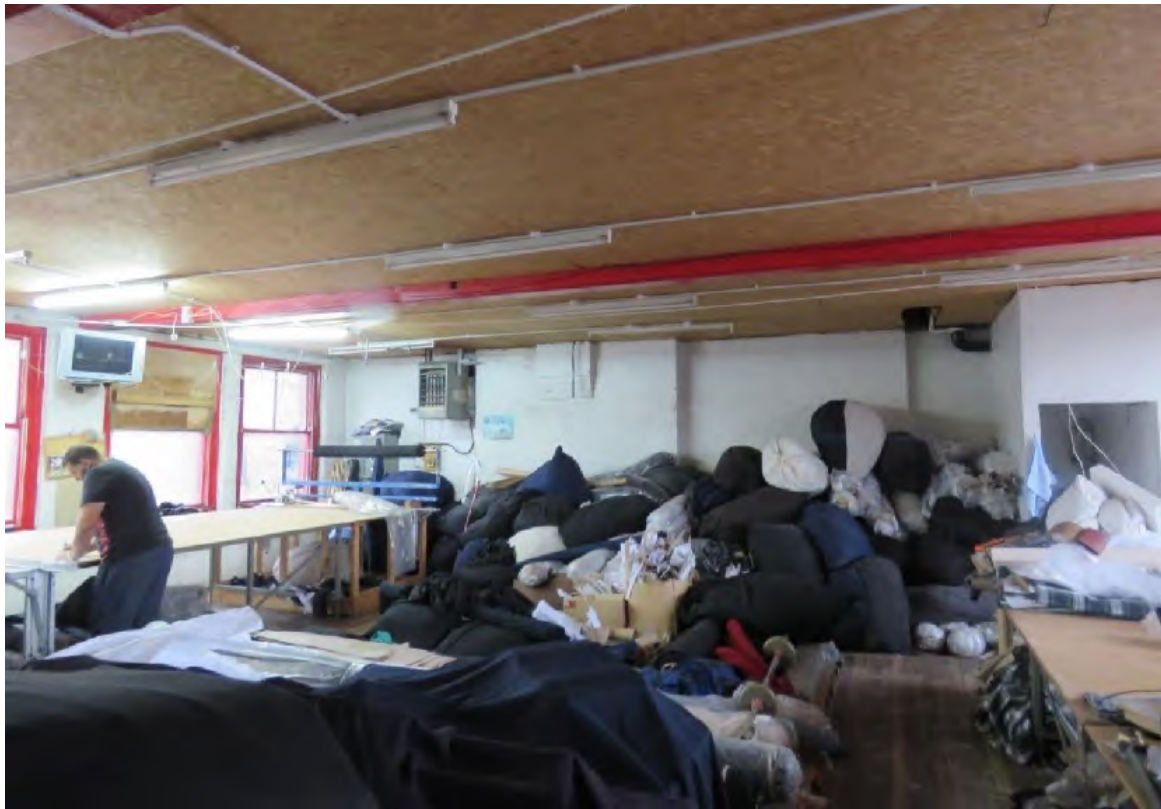
Figure 18 – Looking west across the second floor level.
