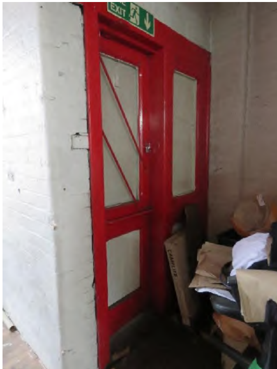
Figure 19 – The original timber teagles doors on the second floor
