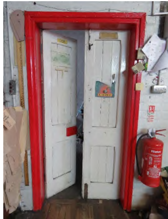
Figure 20 – The original doors leading into the second floor from the separate stone staircase to the eastern end of the building.
