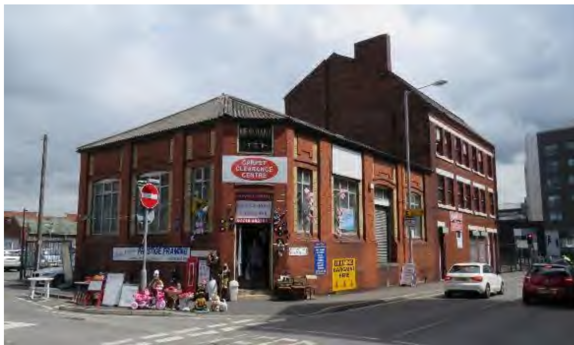
Figure 13 – No. 14 Addington Street (left) and No. 4 Addington Street (right)
