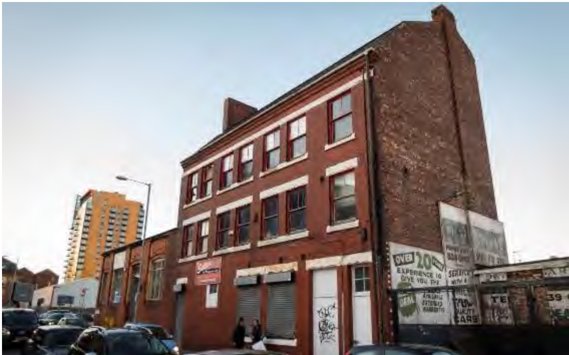
Figure 7 – No. 4 Addington Street
