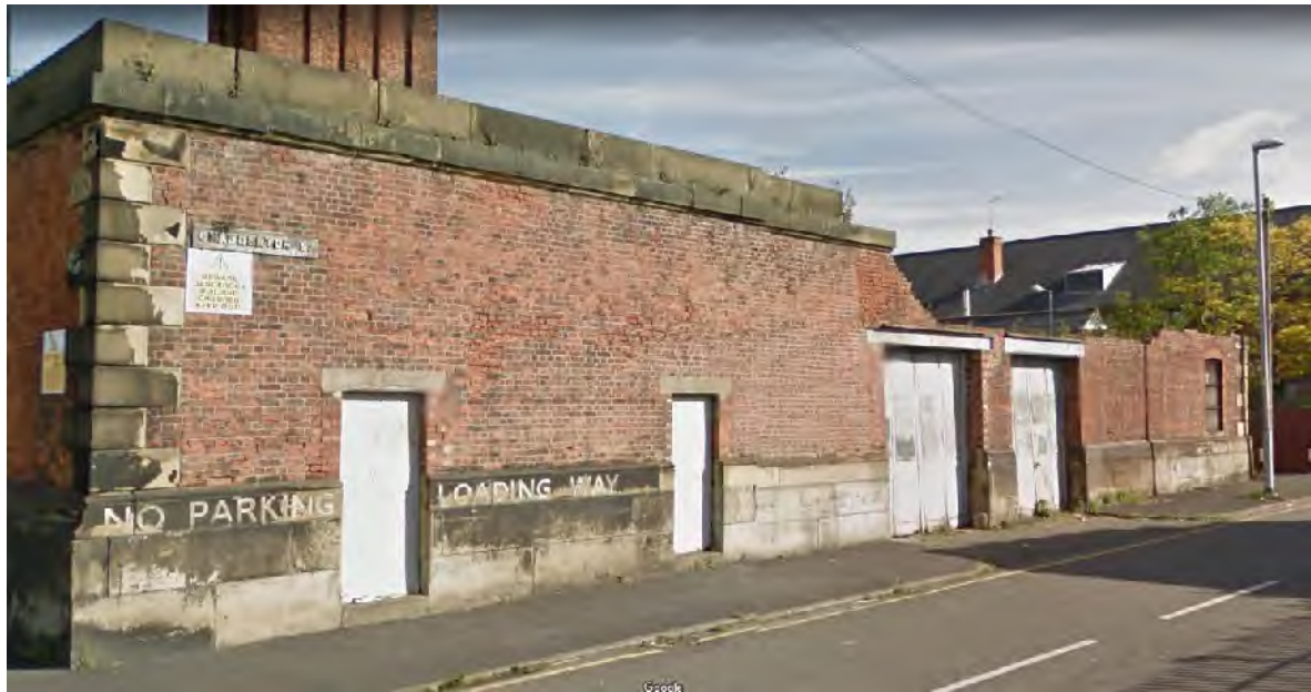
Figure 47 – The Chadderton Street elevation as viewed from Goulden Street.
