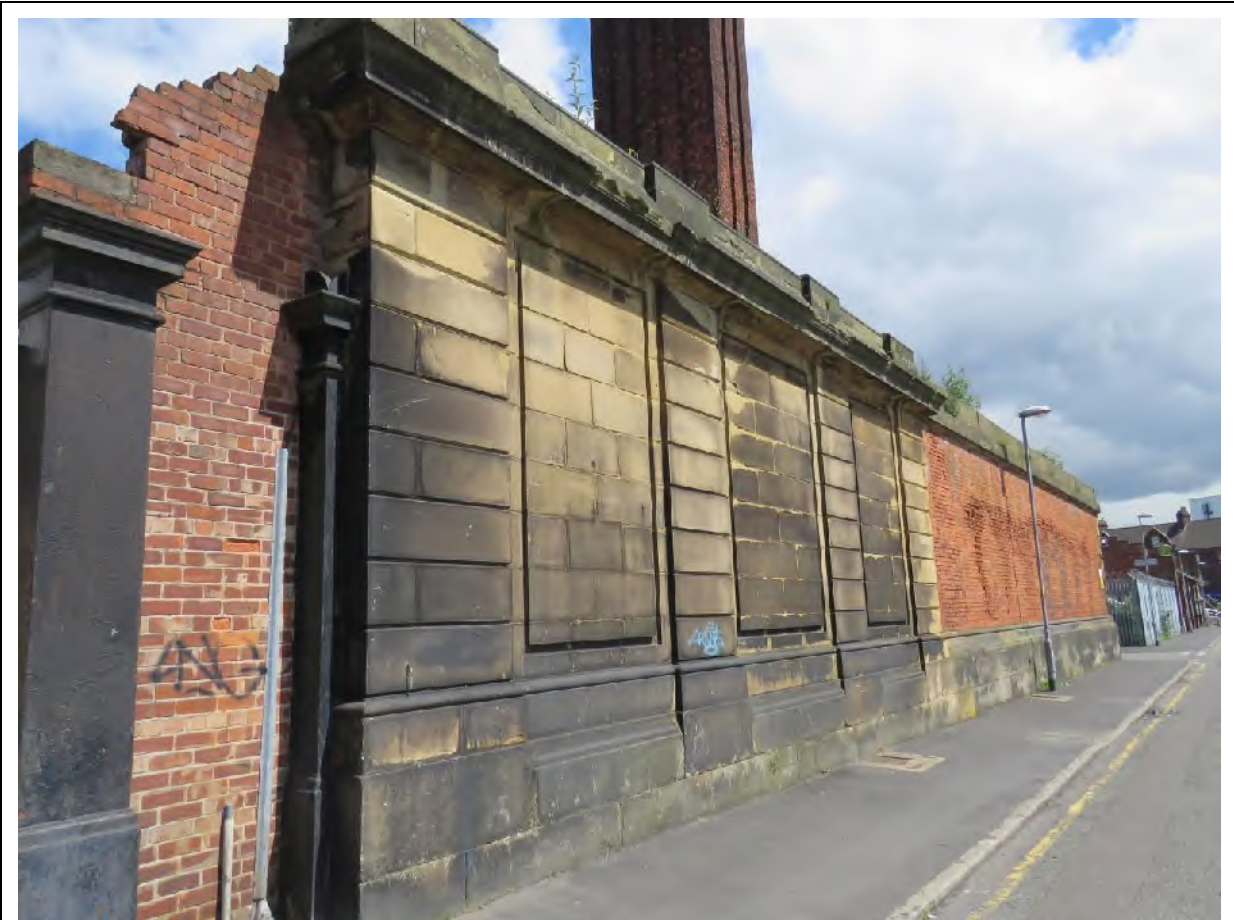
Figure 44 – The rusticated ground floor elevation of the former police station. Note the original pedestrian gate into the yard to the left.
