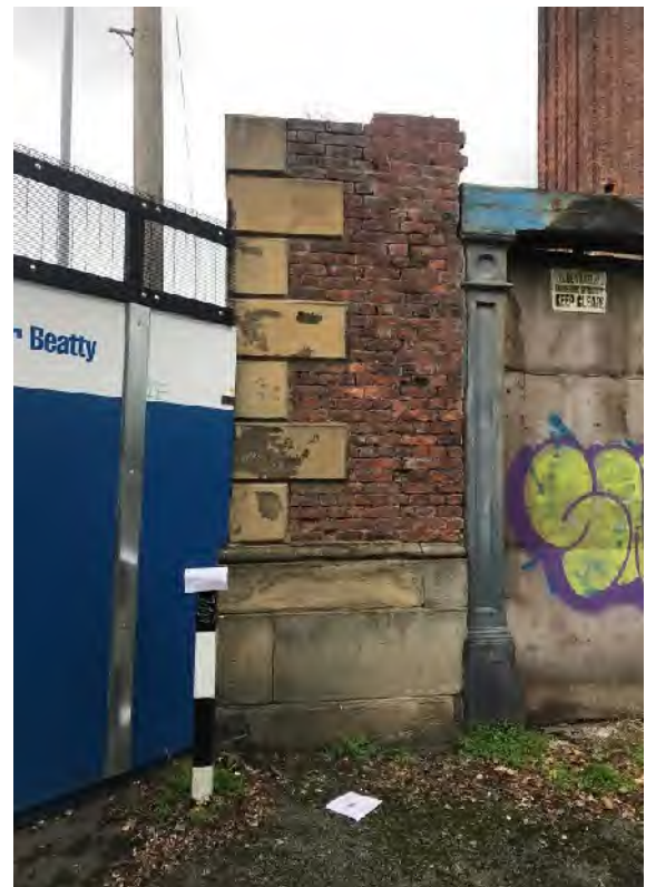
Figure 53 – The original 1870 corner stone quins and brickwork at the junction of Bendix Street (right) and Chadderton Street (left).
