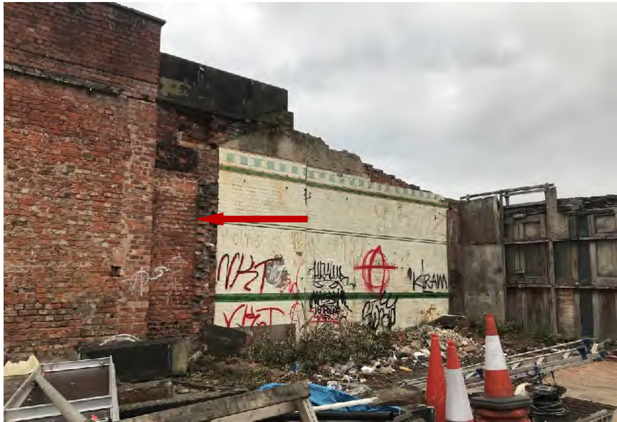
Figure 56 – The remaining 1916 tiled internal wall of the former ambulance station, showing its extended line across the original location of the engine shed and stable (red arrow).
