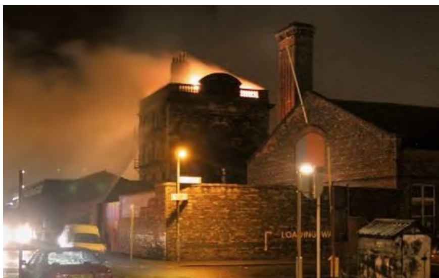
Figure 38 – A view of the police station building on the night it was destroyed by fire in November 2002.
