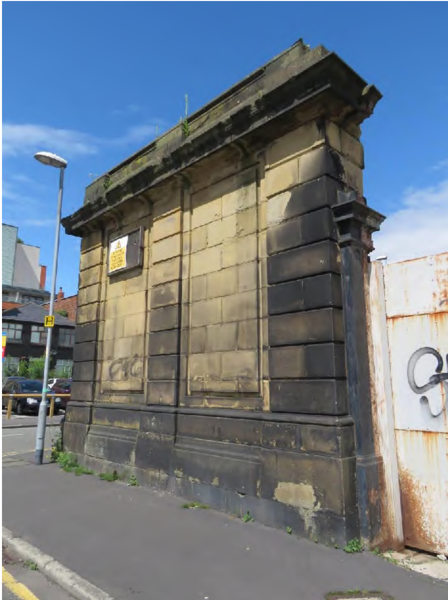
Figure 45 – The rusticated stone ground floor elevation of the former fire station, showing one of two original cast iron gate pilasters.
