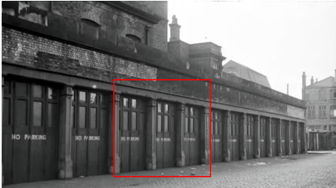
Figure 20 – 1977 photograph of the Bennett Street elevation showing the original three openings (outlined), with the additional 8 openings inserted to the right in 1916, and 2 out of the 3 openings inserted to the left in 1926.
