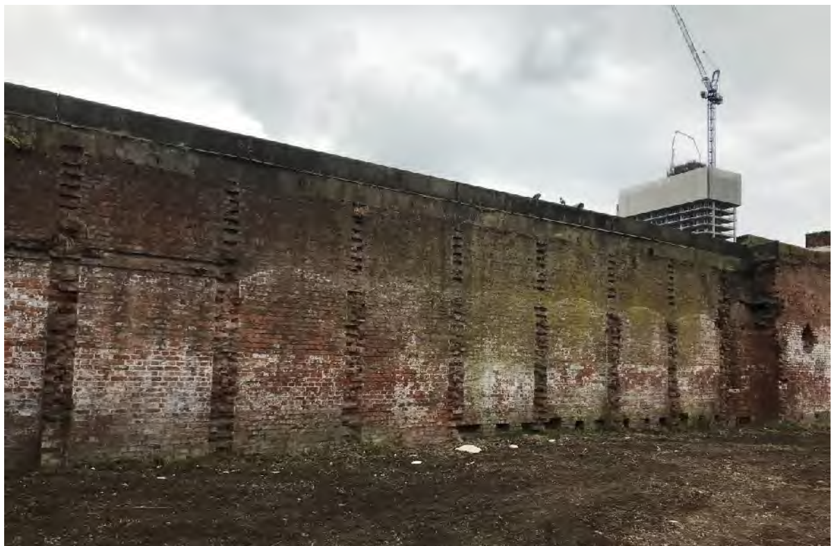
Figure 55 – The internal face of the former police cells on Goulden Street. Note the original location of the barrel-vaulted brick ceilings.
