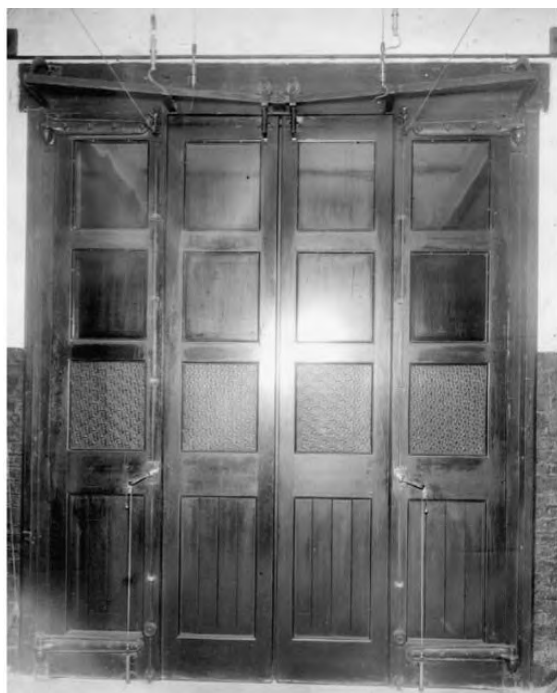
Figure 26 – Internal view of one of the three new fast-release gates of ambulance station facing Chadderton Street in 1902.
