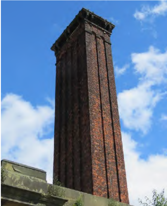
Figure 58 – The ventilation shaft viewed from Goulden Street
