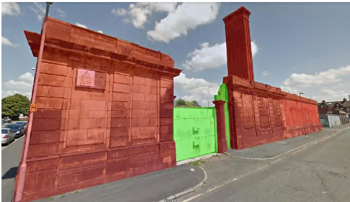
Figure 65 - South-west elevation (Goulden Street)
