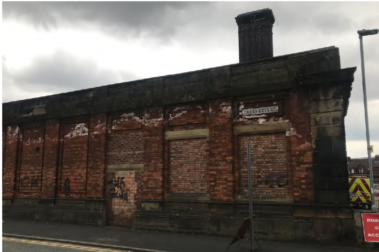
Figure 49 – The western end of the Cross Keys Street elevation. The two window openings to the left were inserted in 1901, whilst the doorway was inserted in 1952 to access the ground floor flat.
