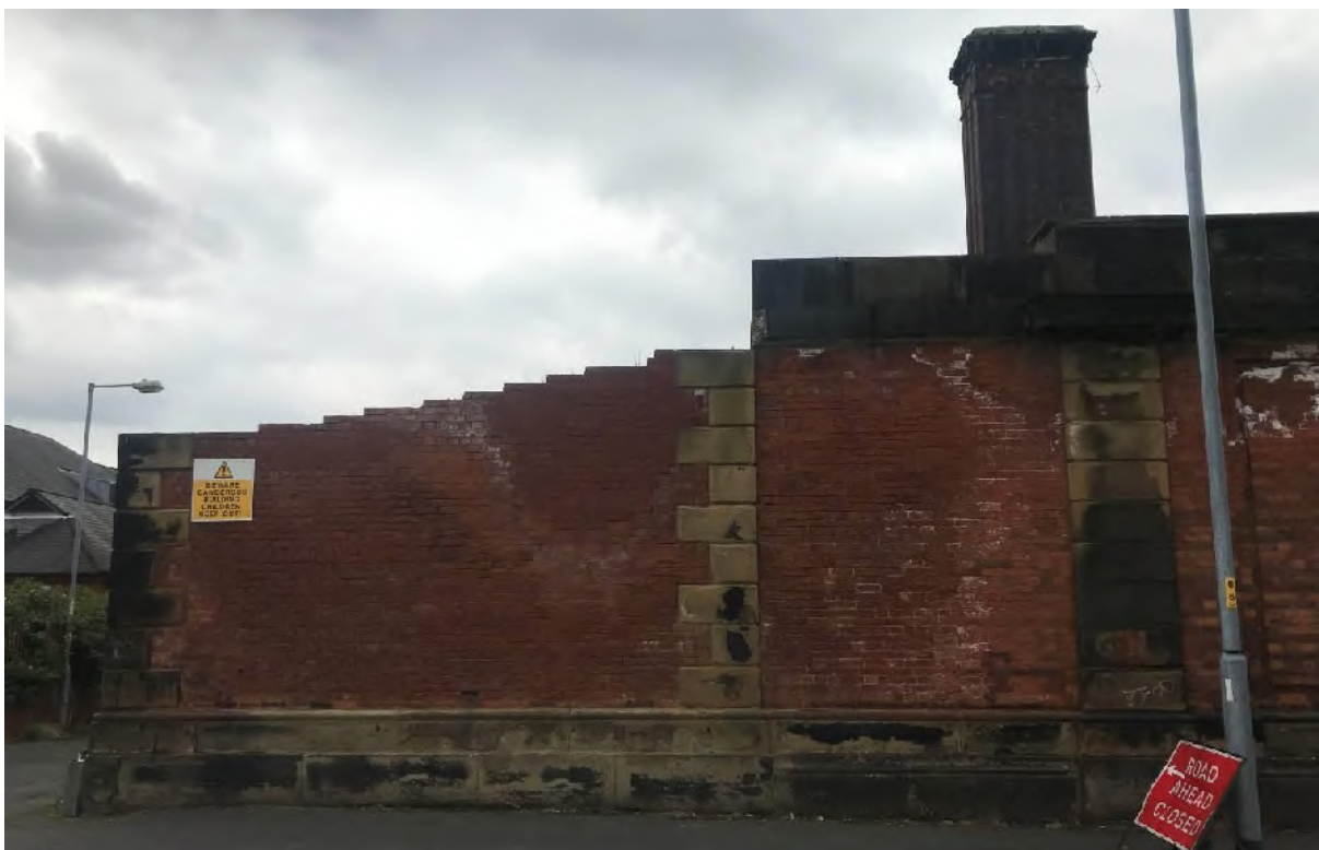
Figure 50 – The corner of Cross Keys Street (right) as it turns into Bendix Street to the left. This elevation illustrates the original stables and engine house use to the left, that was altered in 1916 to form a large new ambulance station.
