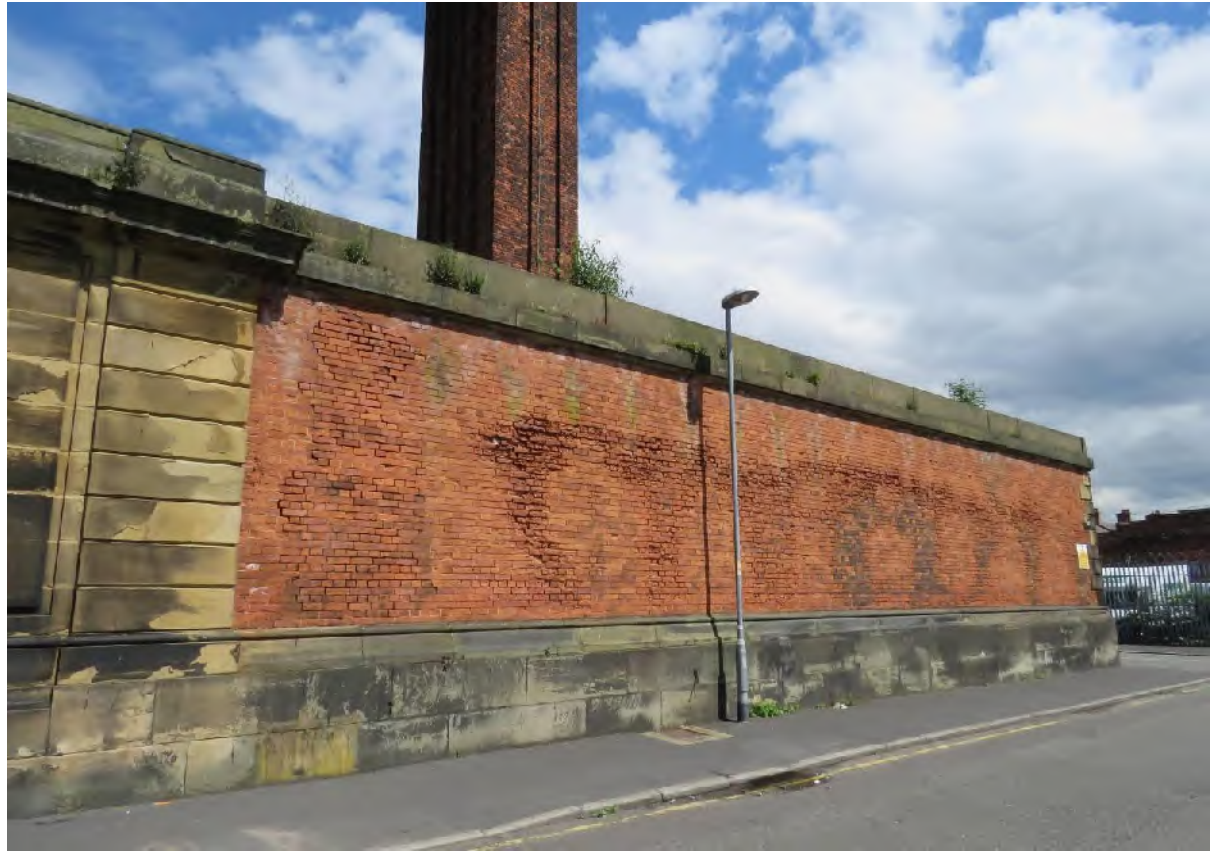
Figure 46 – The external wall of the former single-storey police cells at the southern end of the Goulden Street elevation. Note the weathered marks denoting where each dividing cell wall and ceiling was.
