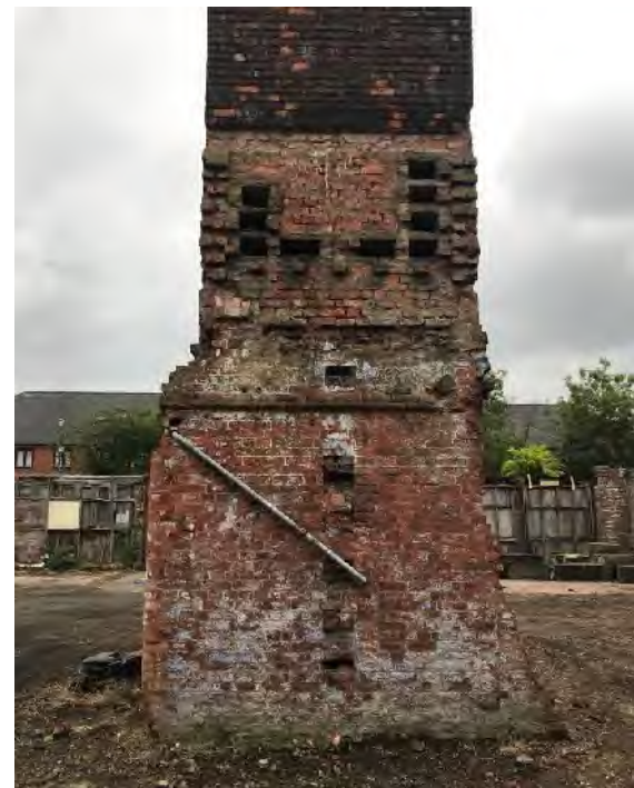
Figure 61 – The base of the shaft looking north.
