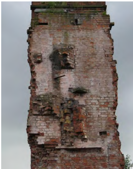
Figure 60 – The upper floor level of the northern side of the shaft, showing its original connections into the police station.
