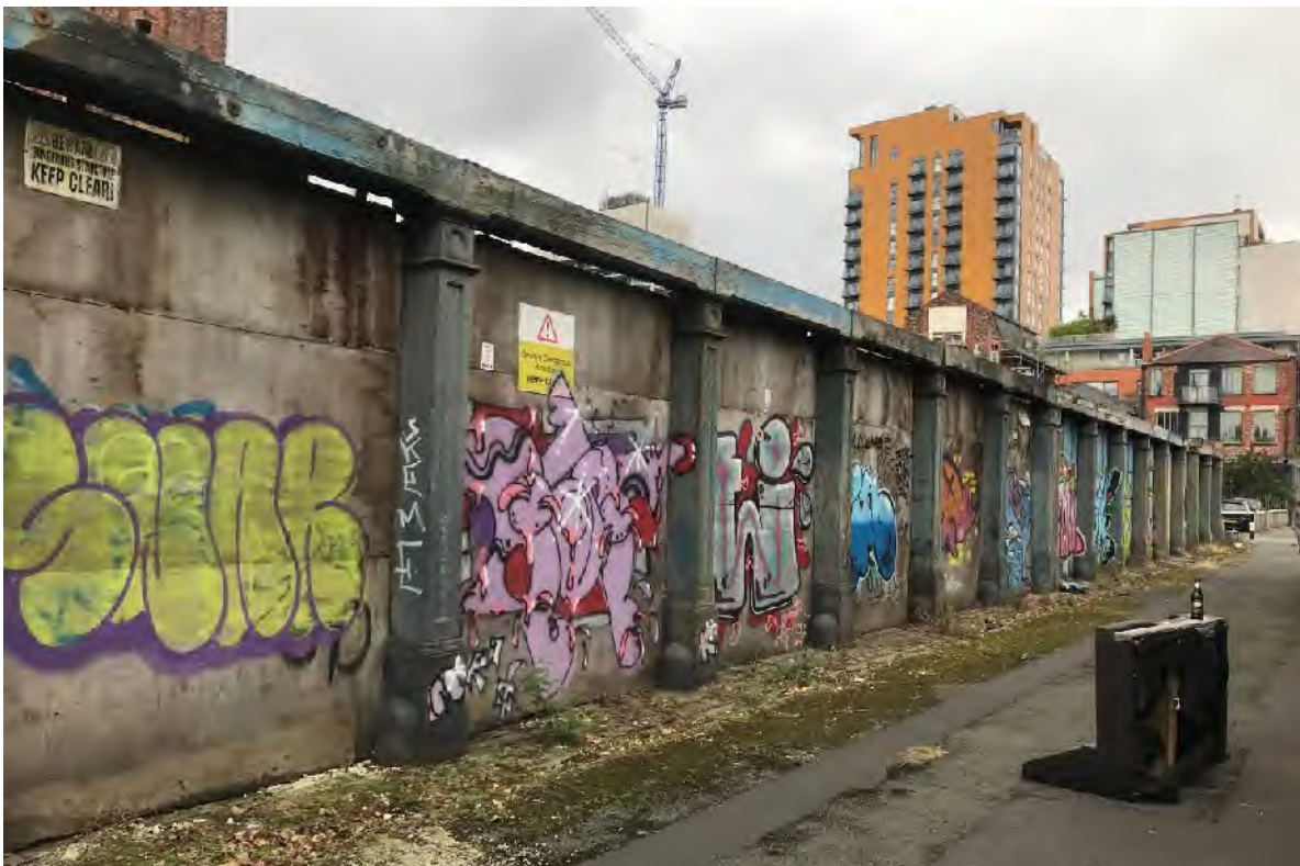
Figure 51 – Looking north-west along Bendix Street showing the three phases of ambulance station gateway openings.
