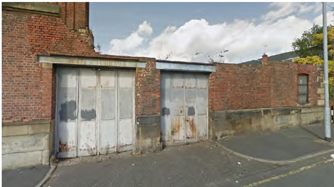
Figure 48 – Two out of the three horse-ambulance openings inserted in 1900 on the Chadderton Street elevation. The third opening, can be seen now blocked to the right.
