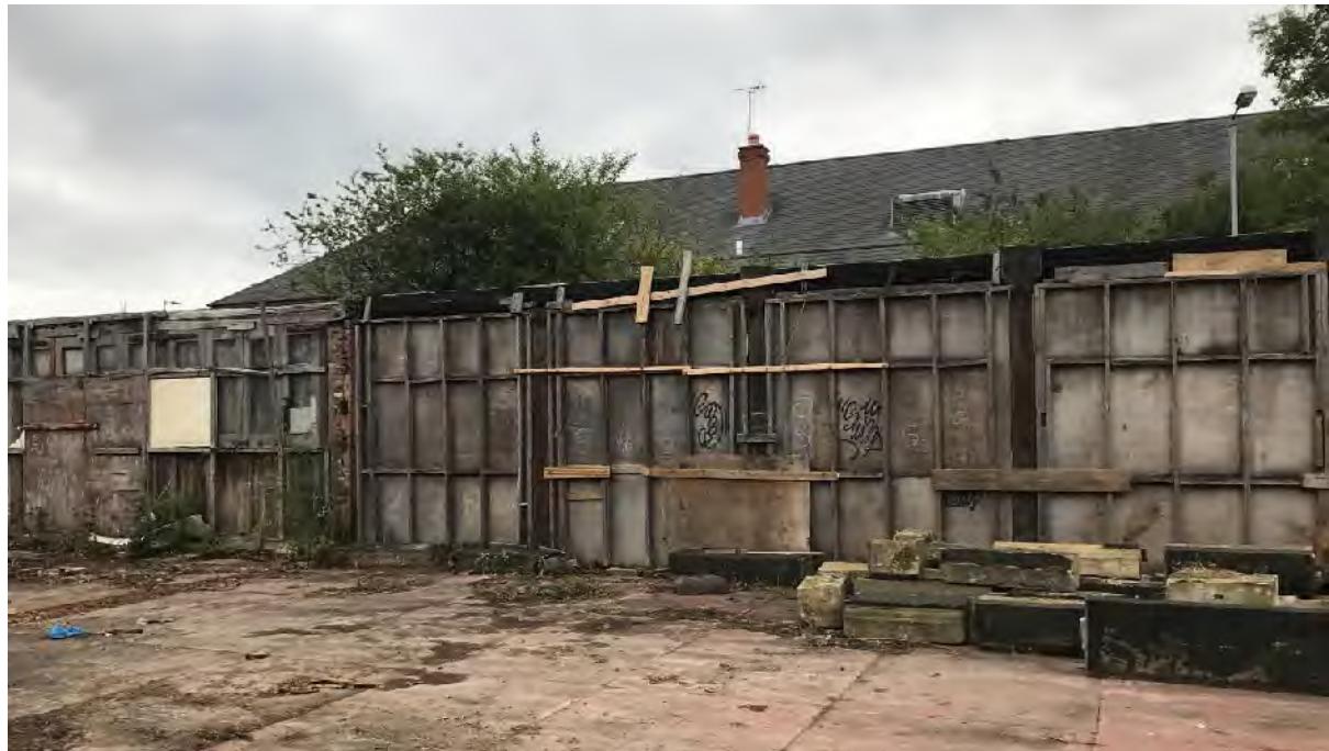
Figure 54 – The internal face of the 1916 ambulance station openings onto Bendix Street.
