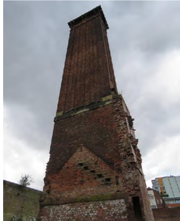
Figure 59 – The ventilation shaft viewed from inside the site, showing the many ventilation duct openings.
