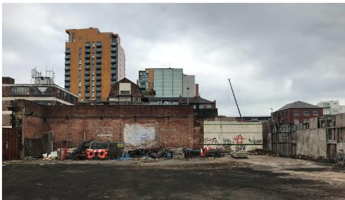
Figure 57 – Looking north towards the internal face of the Cross Keys elevation.
