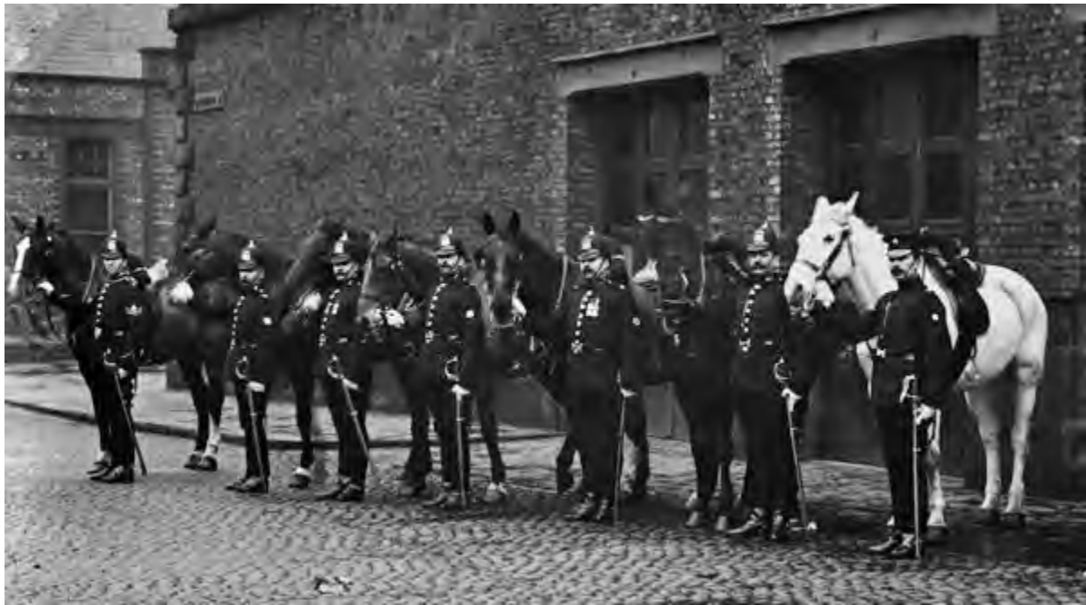
Figure 22 – Circa Early 1900s view showing the original horse-ambulance openings formed in the Chadderton Street elevation, inserted in c1901.
