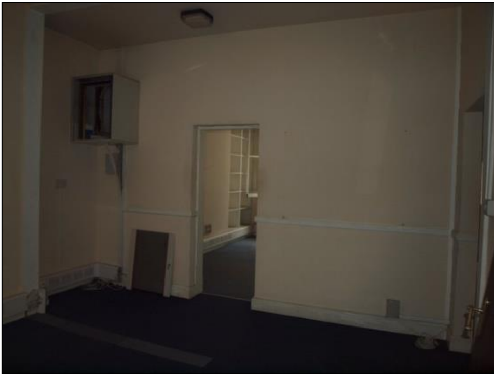
Plate 38: Northern room showing doorway to southern room
