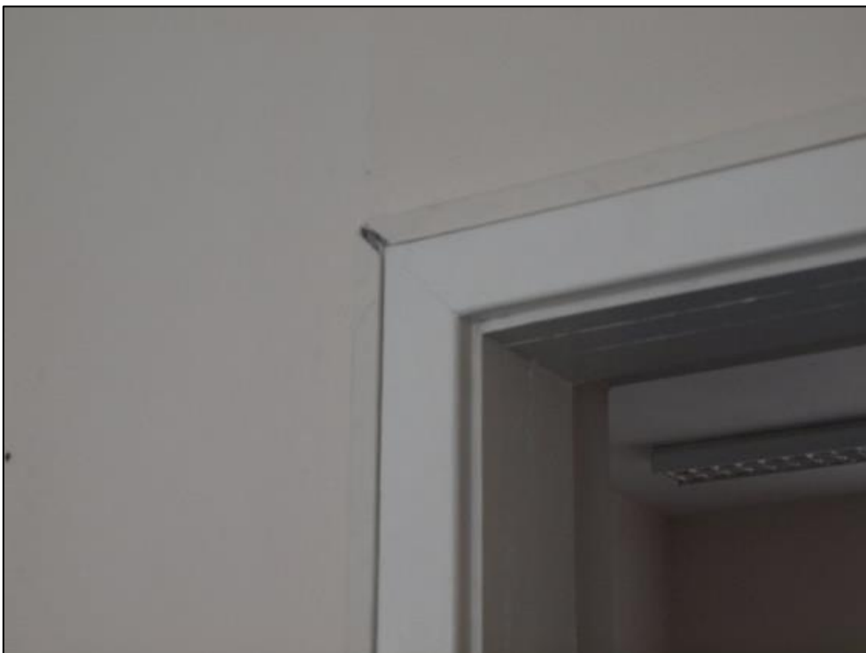
Plate 43: Detail of simple timber moulding around doorway
