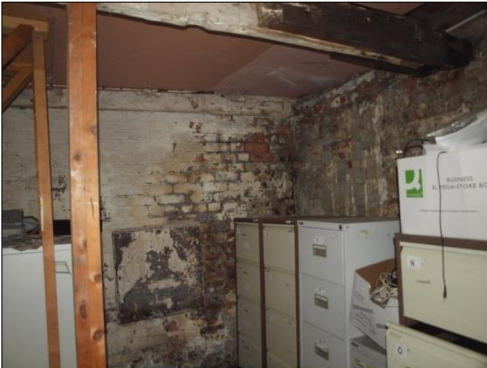
Plate 74: Northern room of basement
