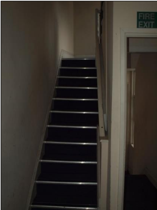
Plate 44: Staircase to second floor
