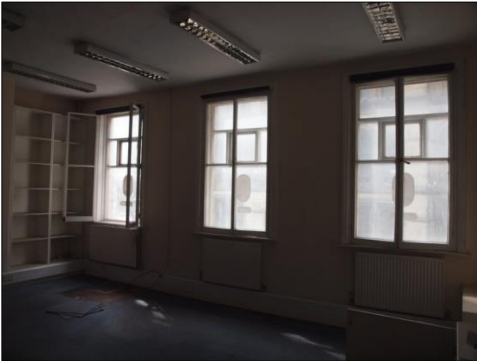
Plate 40: Southern room showing windows
