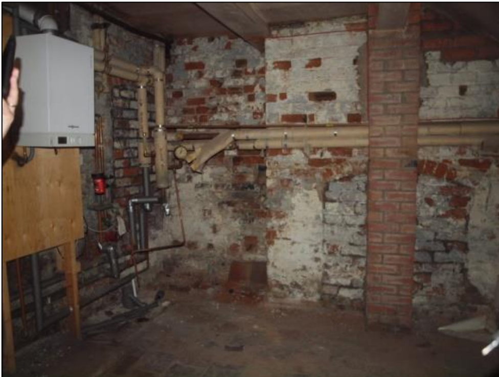
Plate 80: Eastern room of basement showing blocked fireplace
