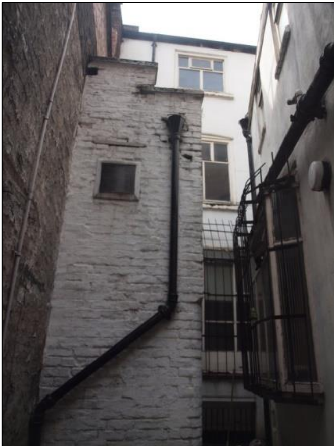
Plate 13: View showing upper floors of rear elevation
