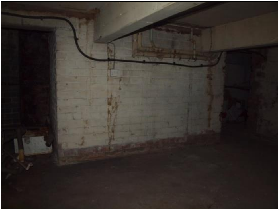
Plate 79: Southern room of basement
