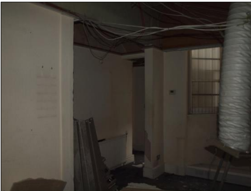
Plate 23: Northern end of ground floor showing passage to northwest extension
