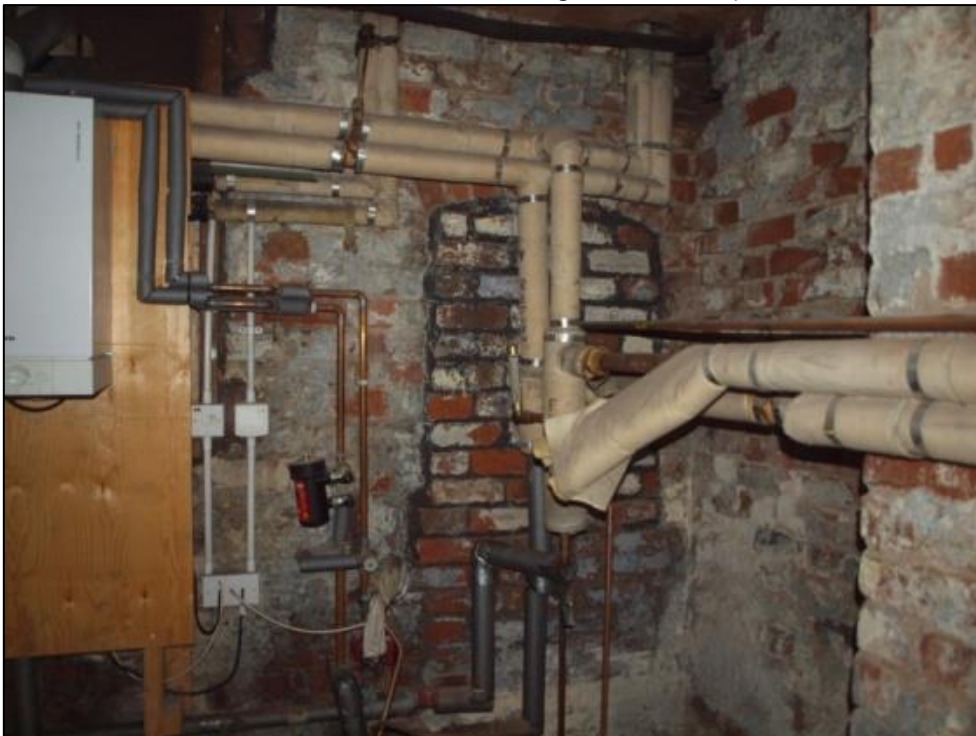
Plate 81: Eastern room of basement showing blocked opening
