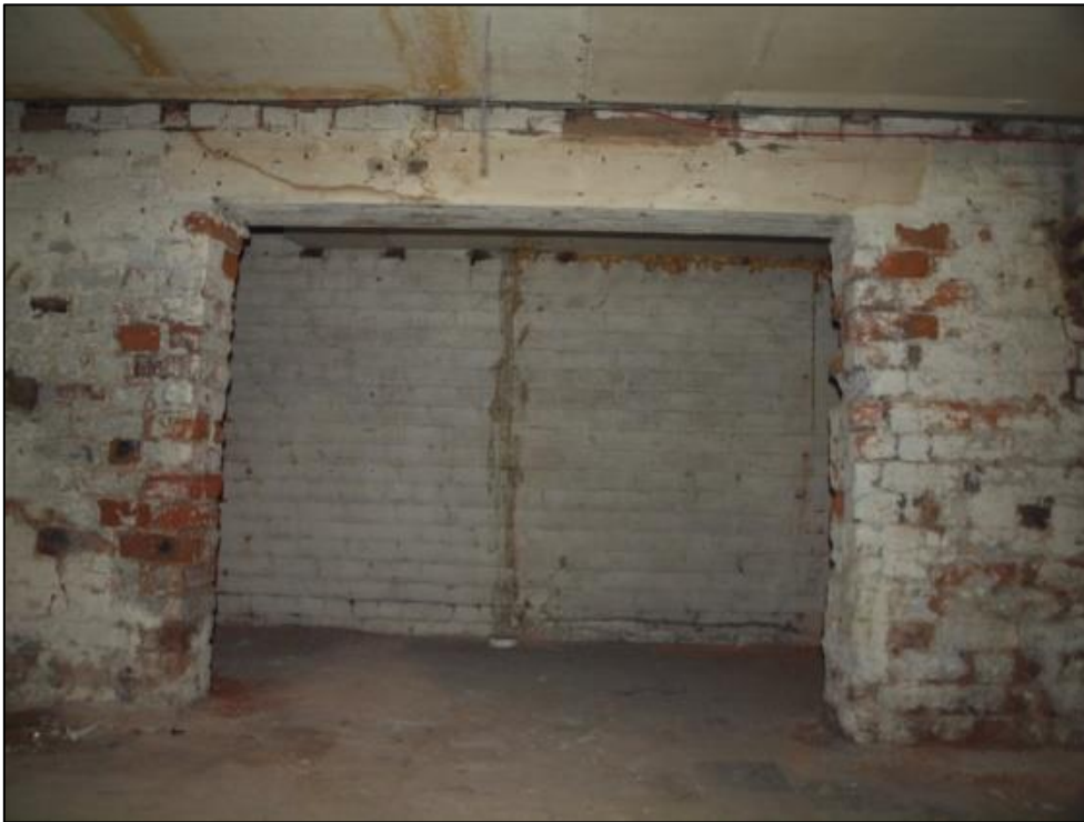
Plate 78: Inserted opening in basement wall to eastern room
