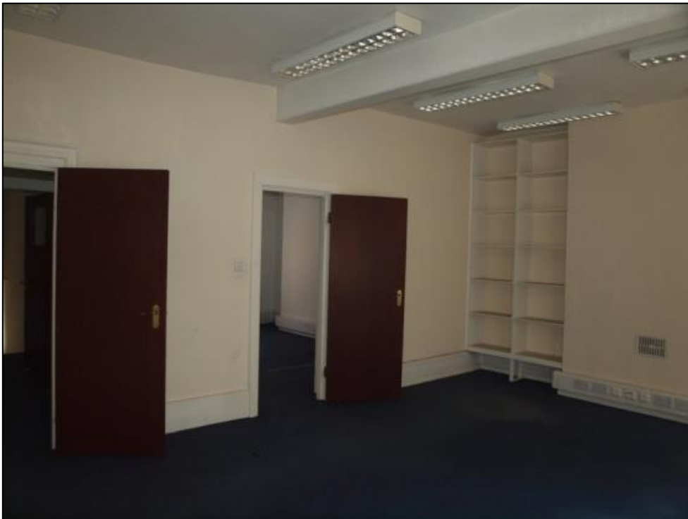
Plate 69: North wall of south room showing modern doors
