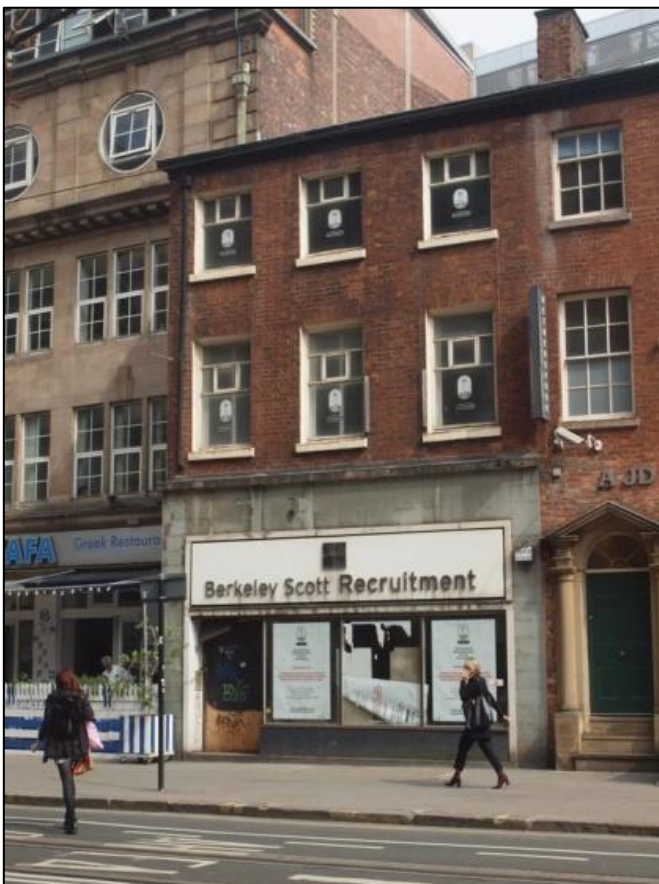
Plate 2: Detail of 65 Princess Street
