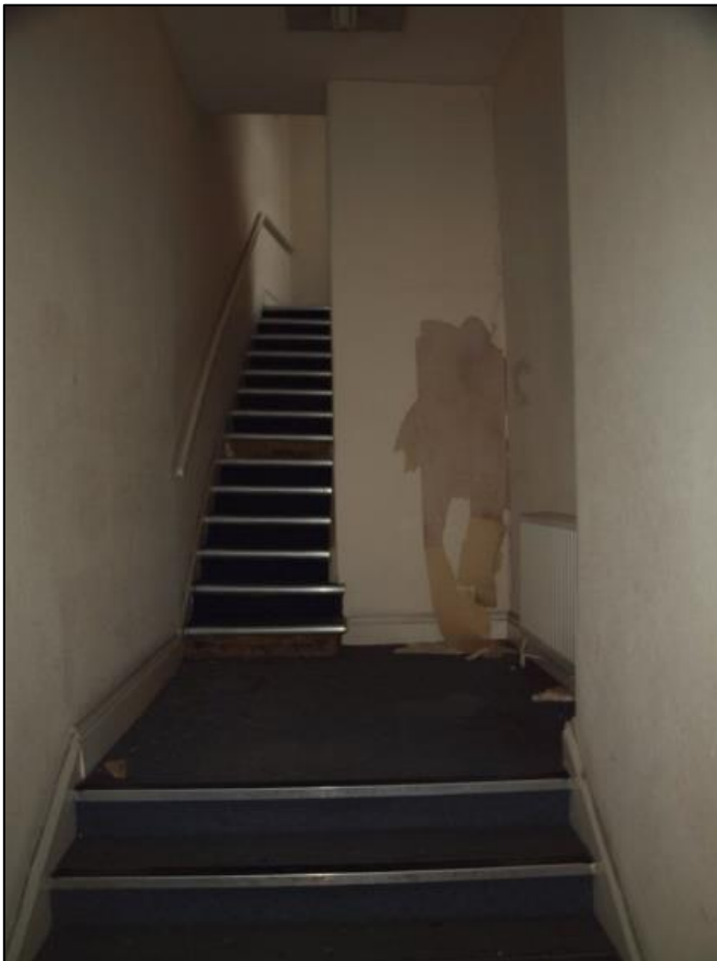
Plate 27: Staircase to first floor
