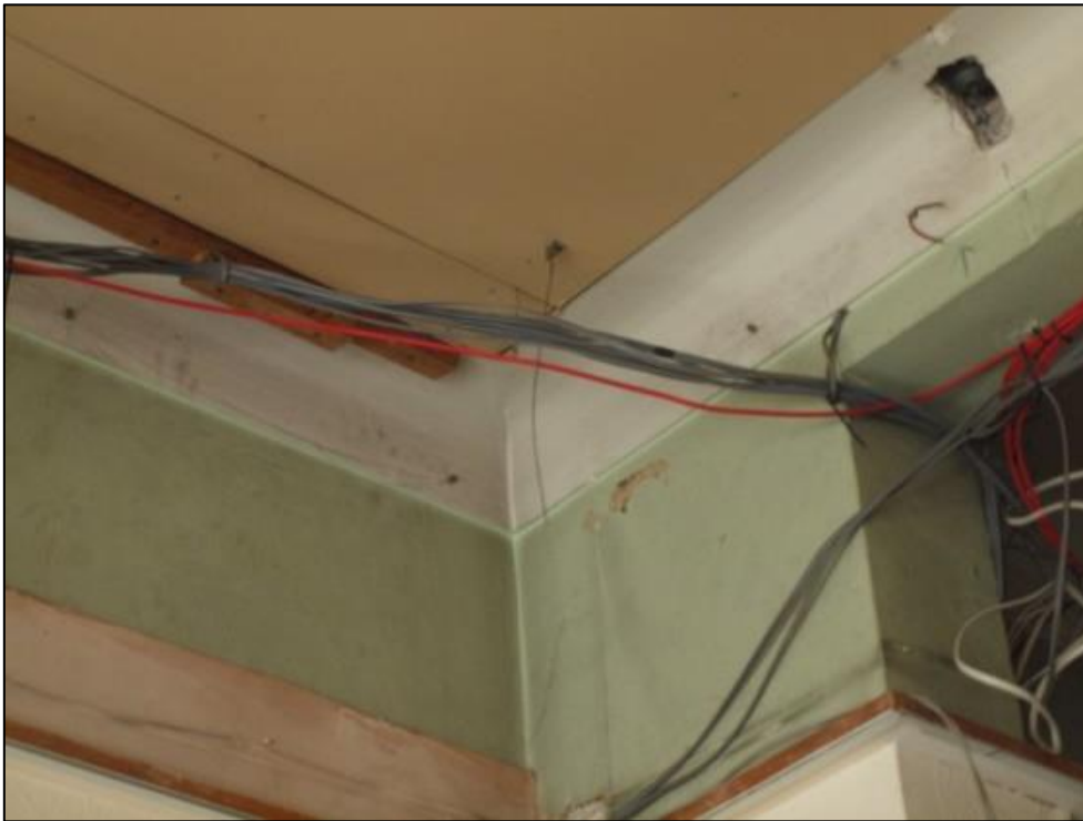
Plate 18: Modern cornice on modern plasterboard ceiling
