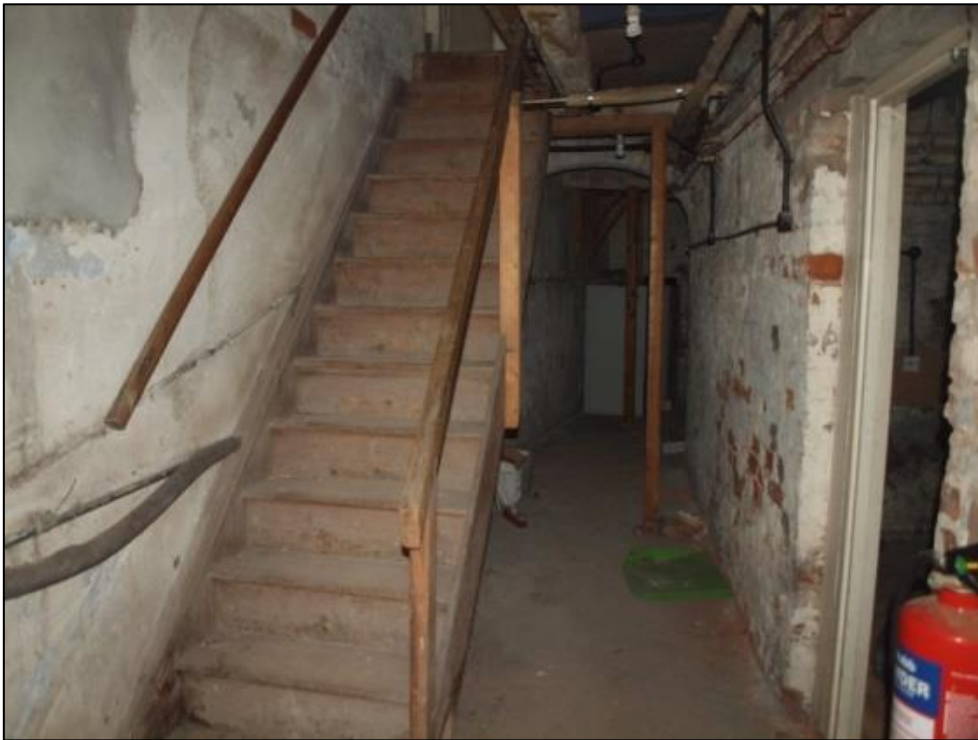
Plate 72: Modern staircase to basement
