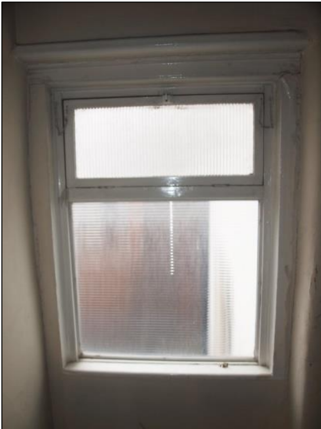
Plate 50: Modern timber framed casement window on landing
