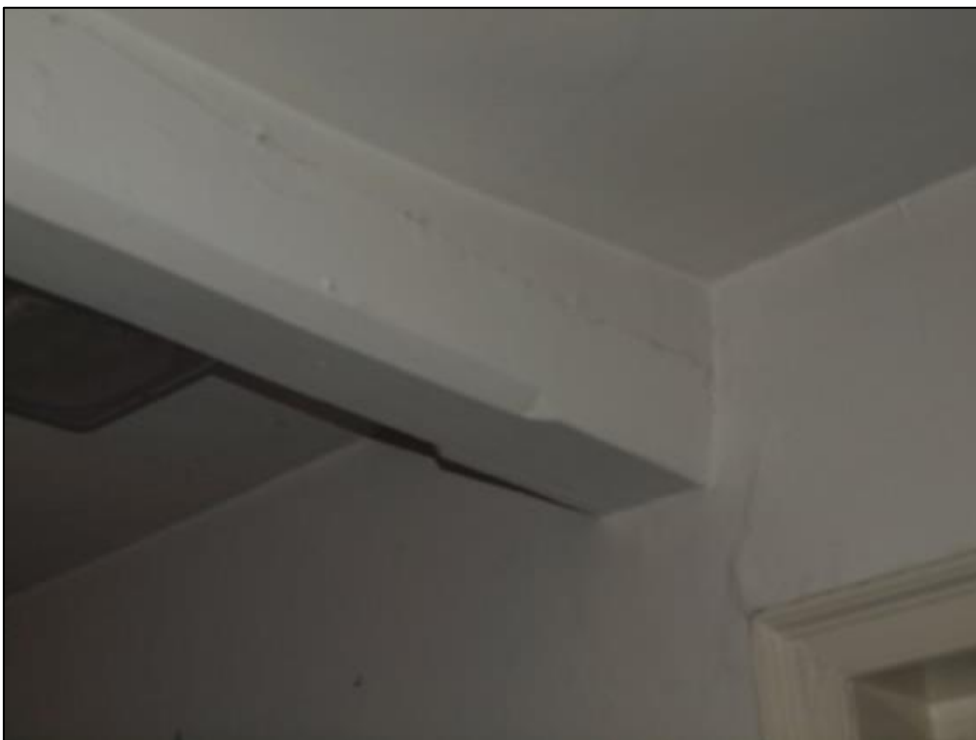
Plate 65: Chamfered and stopped timber beam in north room
