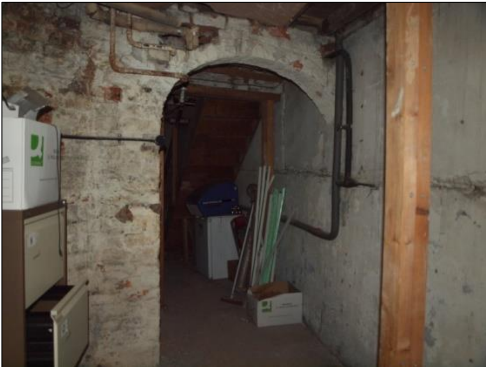
Plate 75: Northern room of basement looking south
