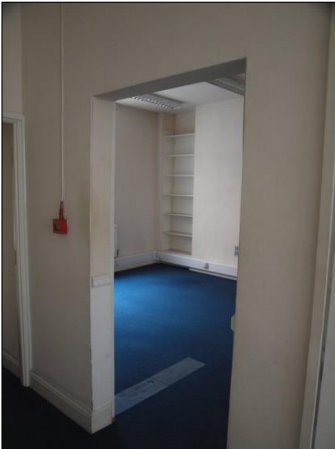
Plate 36: Doorway to northern room of first floor
