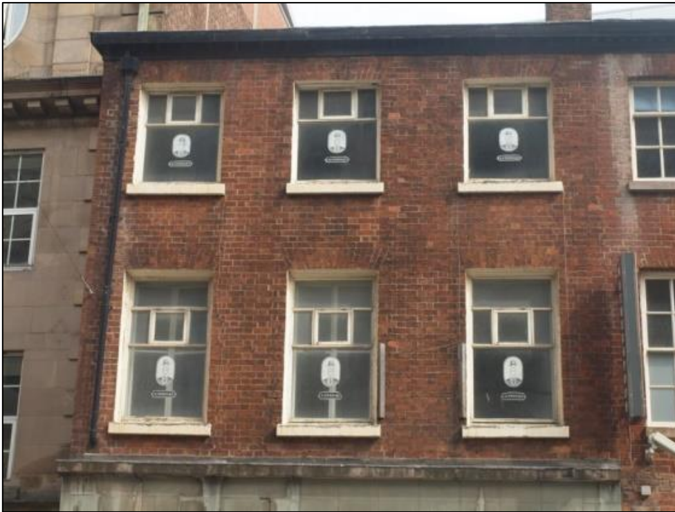
Plate 5: First and second floor windows
