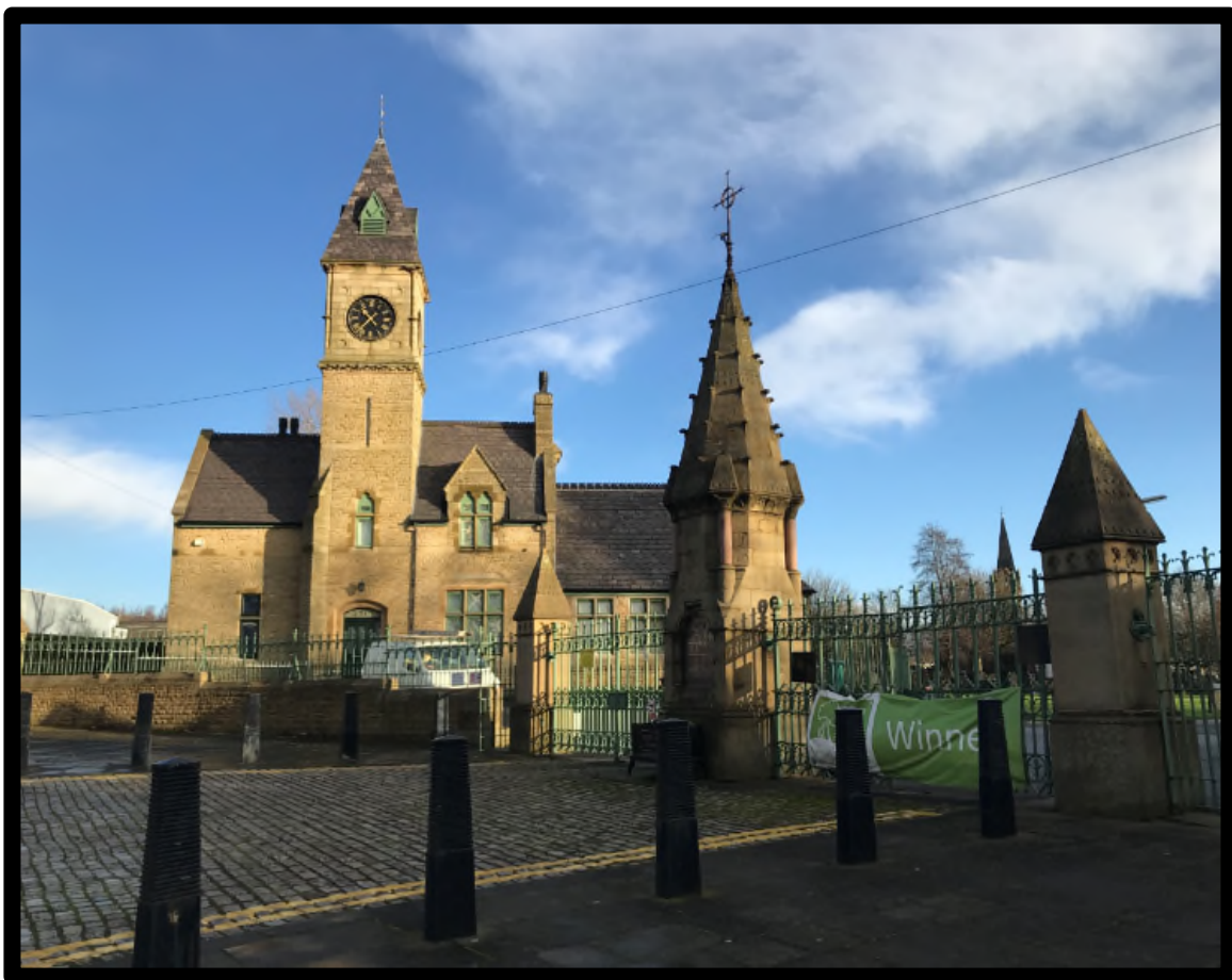
Figure 4.4: Cemetery Office at Phillips Park Cemetery Principal Facade (Source: Author's Own, December 2019)
