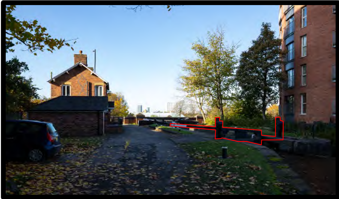
Figure 5.8: Ashton Canal Lock Number 7 with Roving Bridge Immediately East of Mill Street Bridge (Source, Planit.i.e. November 2019)
