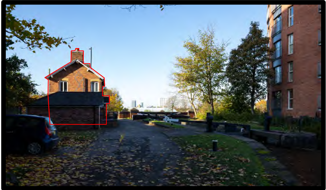
Figure 6.12: Lock Keepers Cottage (original)(Source: Planit.i.e, November 2019)
