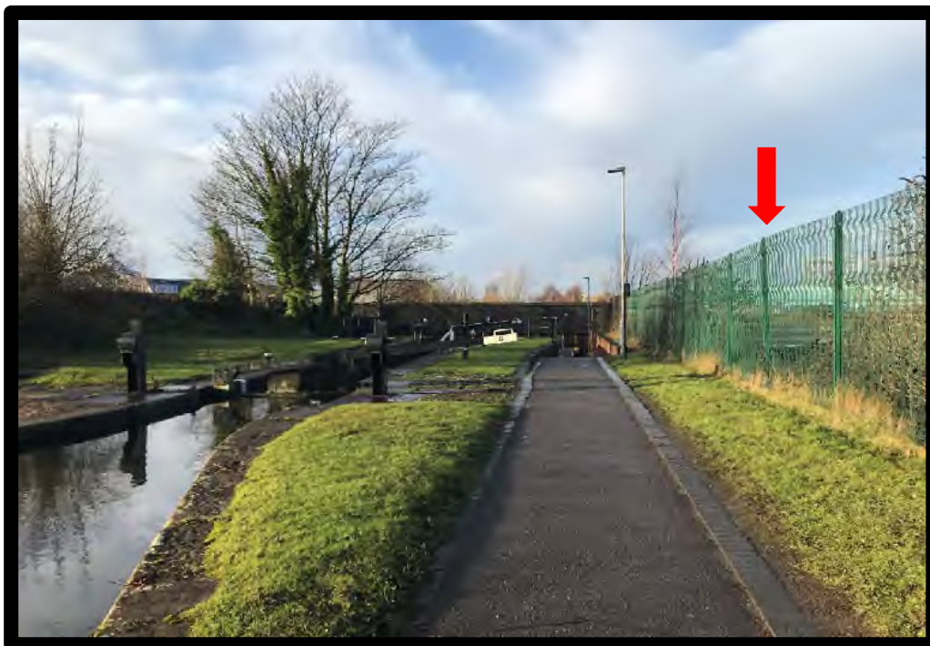
Figure 6.7: View of Lock 6 with location of Proposed Development indicated by the red arrow
