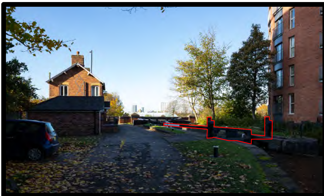
Figure 6.10: Lock 7 (original) (Source: Planit.i.e, November 2019)
