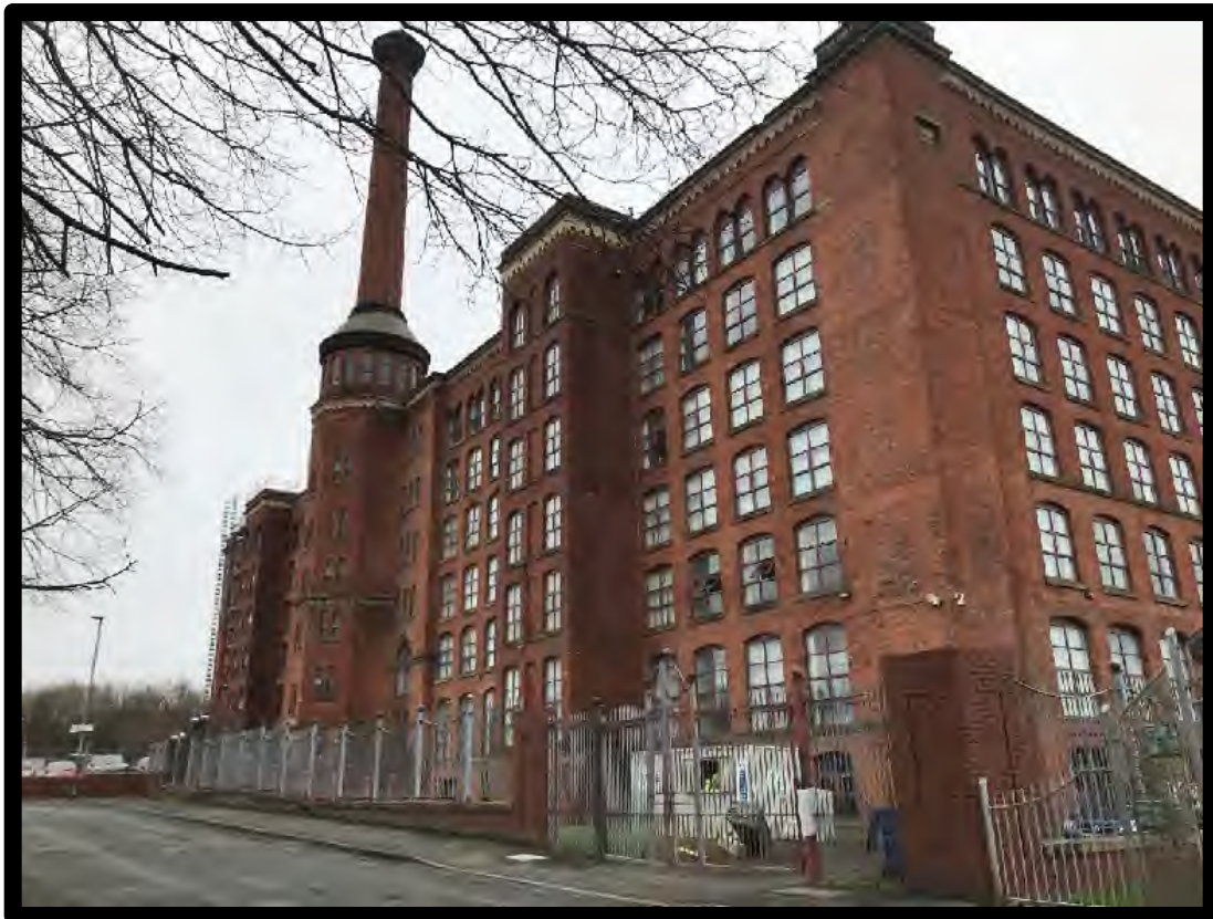
Figure 5.12: Victoria Mill's Principal Facade (Source: Author's Own, 2020)
