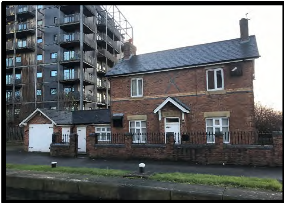
Figure 5.11: Principle Facade of the Lock Keepers Cottage (Source: Author's Own, 2019)
