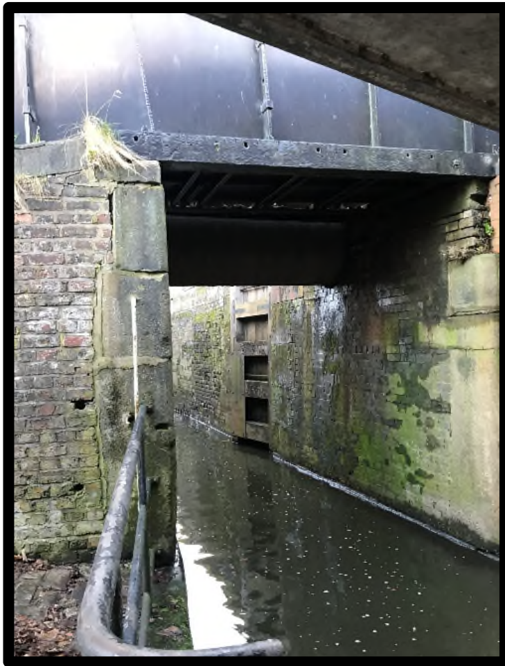
Figure 4.8: Mill Street Bridge (Source: Author's Own, December 2019)
