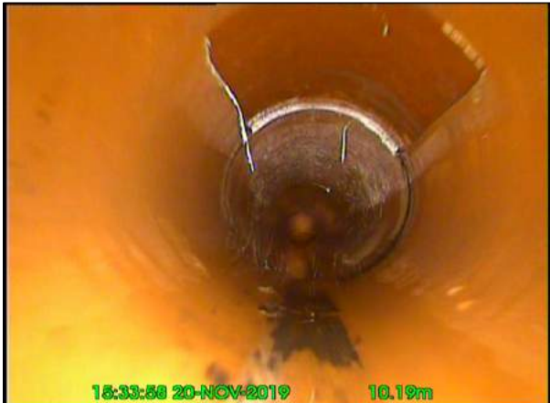
Photo: 6_7A 10.4m, Point repair, hole repaired, from 11 to 1 o'clock, Start
