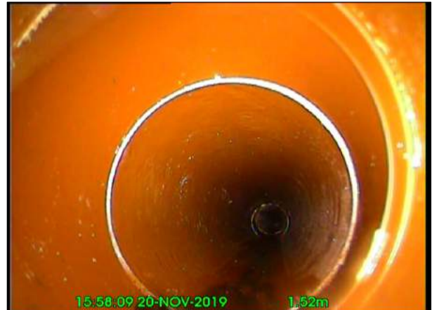
Photo: 10_3A 1.6m, Line deviates right
