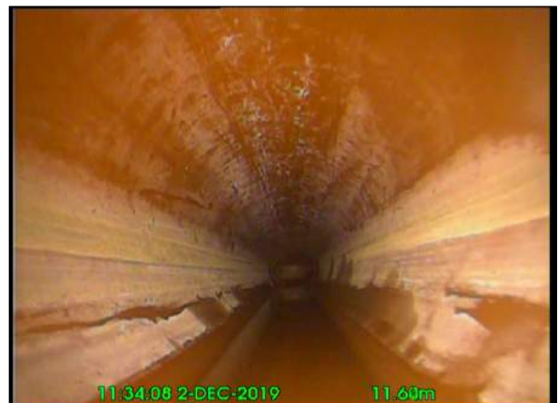
Photo: 22_5A 11.6m, Clear water level, 10% of the vertical dimension
