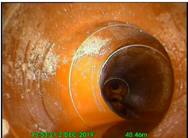
Photo: 24_20A 40.46m, Point repair, hole repaired, from 10 to 2 o'clock, End
