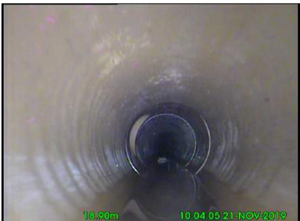
Photo: 15_9A 18.9m, Turbid water level, 10% of the vertical dimension
