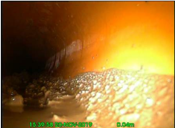
Photo: 7_2A 0m, Turbid water level, 5% of the vertical dimension
