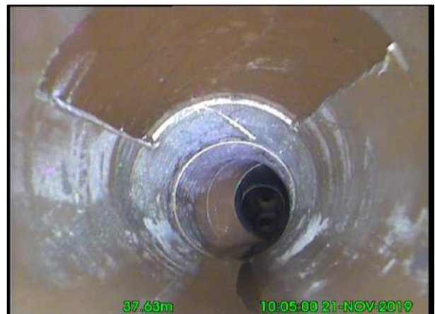
Photo: 15_19A 37.7m, Point repair, hole repaired, from 10 to 2 o'clock, Start
