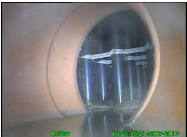
Photo: 18_4A 1.3m, Line deviates right
