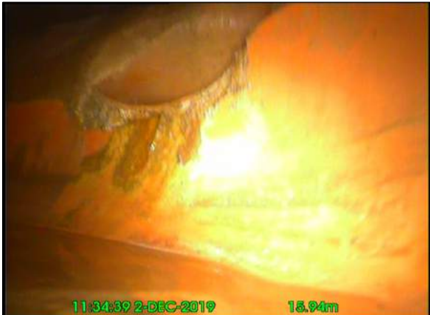
Photo: 22_10A 16m, Finish node type, manhole reference number: S07
