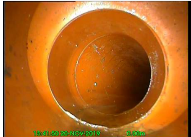
Photo: 8_3A 0.3m, Shape changes to circular, 100mm high
