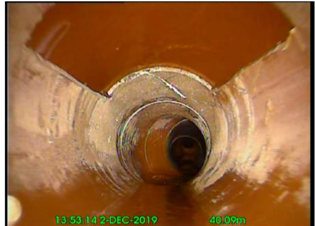
Photo: 24_19A 40.2m, Point repair, hole repaired, from 10 to 2 o'clock, Start
