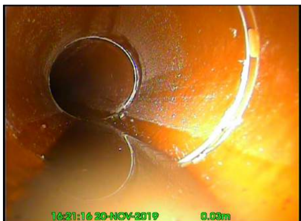
Photo: 3_2A 0m, Clear water level, 10% of the vertical dimension
