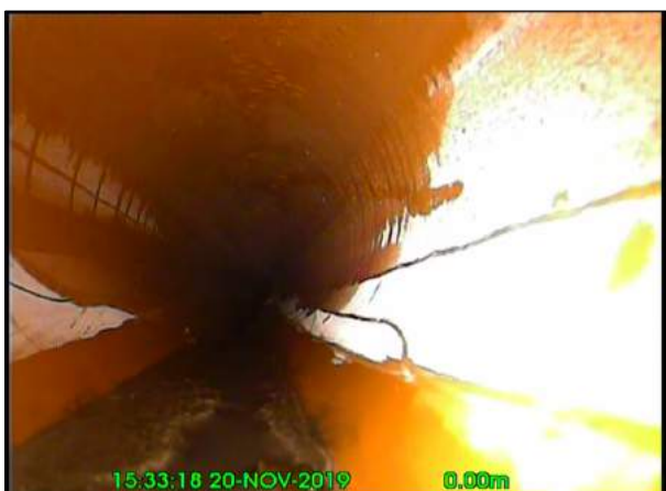
Photo: 6_2A 0m, Turbid water level, 10% of the vertical dimension
