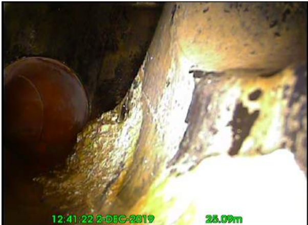
Photo: 20_14A 25.1m, Finish node type, manhole reference number: S05
