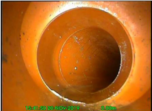
Photo: 8_2A 0m, Clear water level, 5% of the vertical dimension
