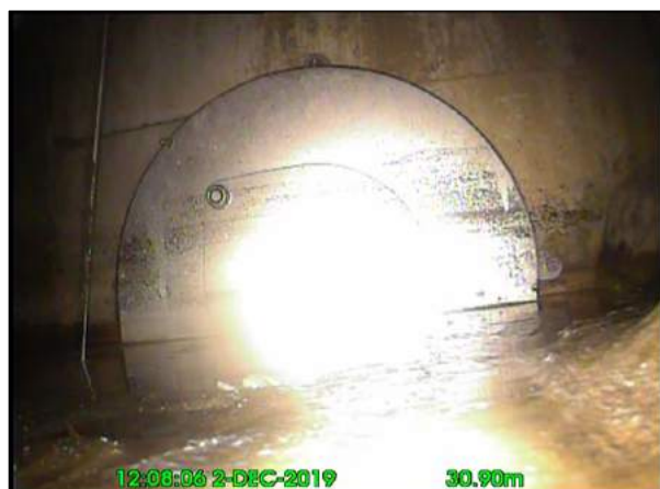
Photo: 25_3A 30.9m, Finish node type, manhole reference number: S08
