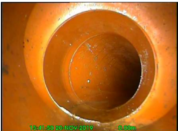
Photo: 8_4A 0.3m, Line deviates right
