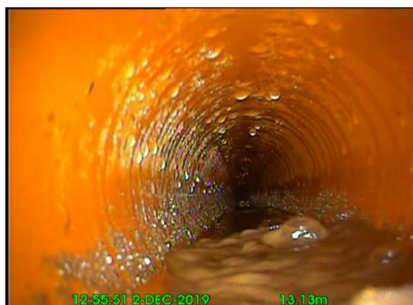
Photo: 21_8A 13.2m, Settled deposits, fine, 10% cross-sectional area loss
