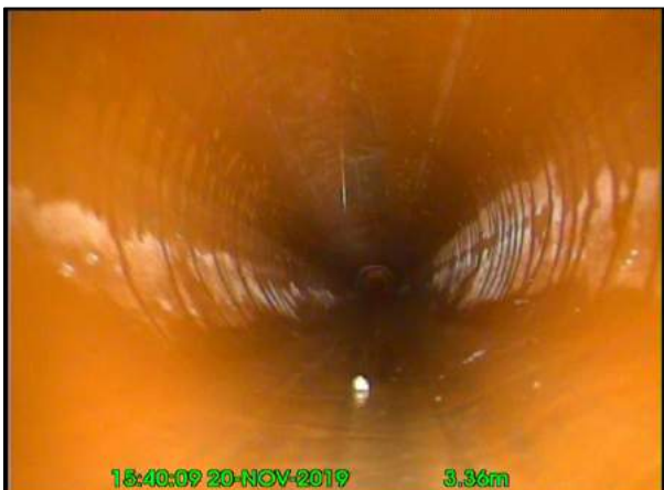
Photo: 7_5A 3.36m, Water level, 0% of the vertical dimension
