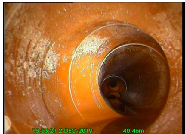
Photo: 24_21A 40.6m, Line deviates right
