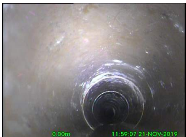
Photo: 11_2A 0m, Turbid water level, 15% of the vertical dimension
