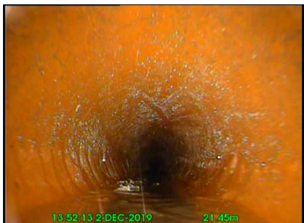
Photo: 24_12A 21.45m, Clear water level, 20% of the vertical dimension
