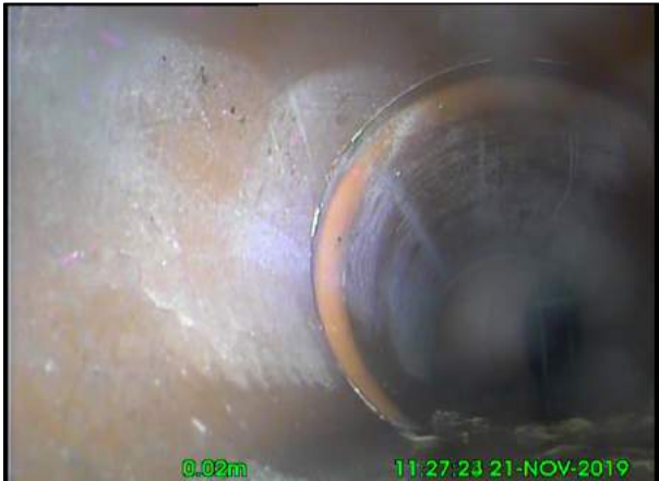
Photo: 18_2A 0m, Clear water level, 10% of the vertical dimension
