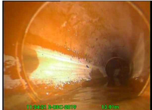
Photo: 22_7A 13.9m, Line deviates right
