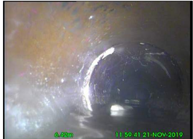
Photo: 11_7A 6.45m, Clear water level, 20% of the vertical dimension
