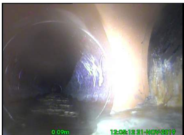
Photo: 12_2A 0m, Clear water level, 15% of the vertical dimension
