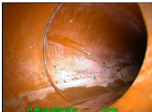
Photo: 23_3A 0.2m, Line deviates right
