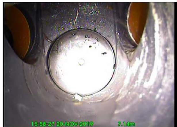
Photo: 10_5A 7.2m, Finish node type, manhole reference number: S14
