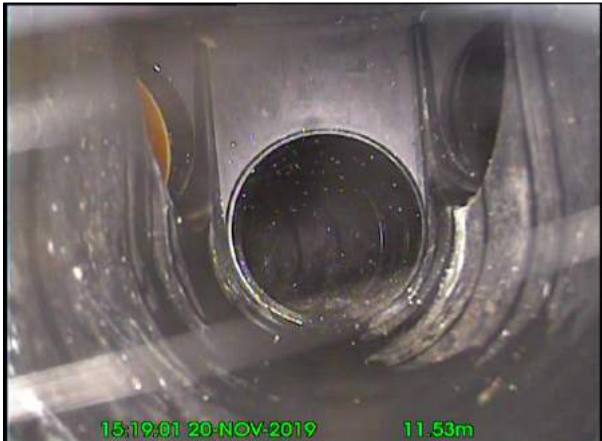
Photo: 5_6A 11.4m, Finish node type, manhole reference number: S15
