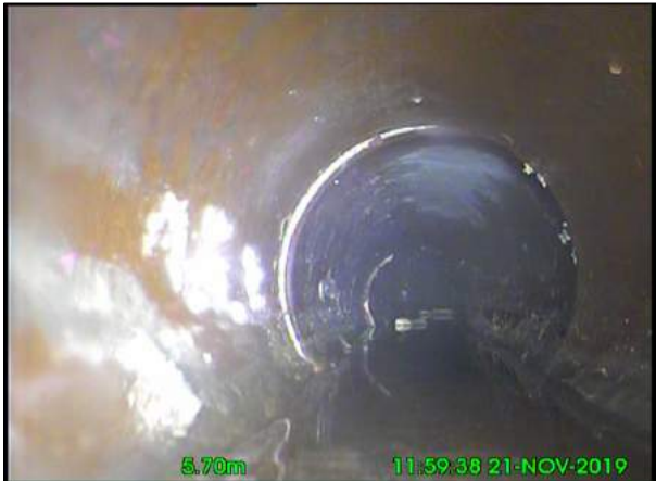
Photo: 11_6A 5.7m, Clear water level, 15% of the vertical dimension
