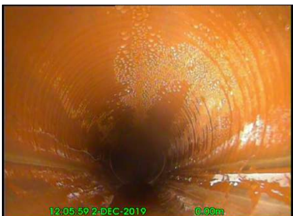
Photo: 25_2A 0m, Clear water level, 5% of the vertical dimension
