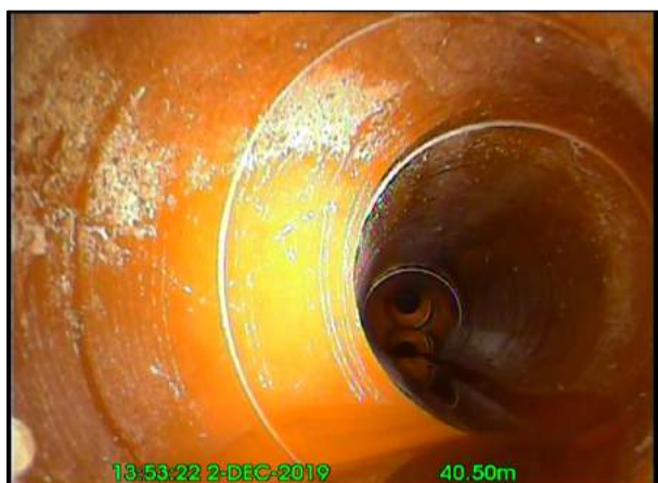
Photo: 24_22A 40.7m, Shape changes to circular, 100mm high
