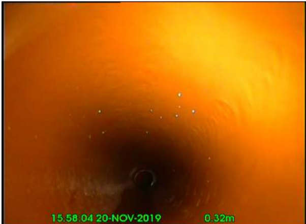
Photo: 10_2A 0m, Clear water level, 5% of the vertical dimension
