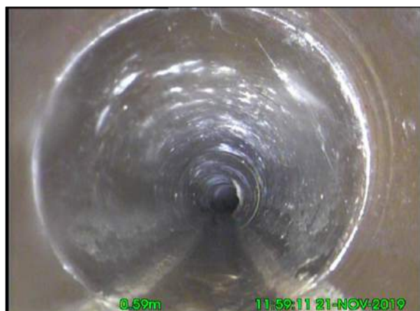
Photo: 11_3A 0.6m, Clear water level, 10% of the vertical dimension
