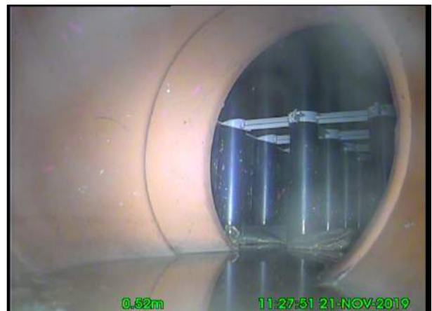
Photo: 18_6A 1.9m, Finish node type, other special chamber reference number: Tank Remarks: Tank
