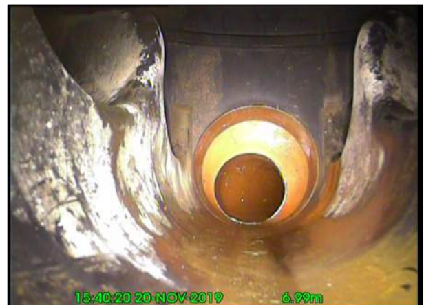
Photo: 7_6A 6.99m, Finish node type, manhole reference number: S11
