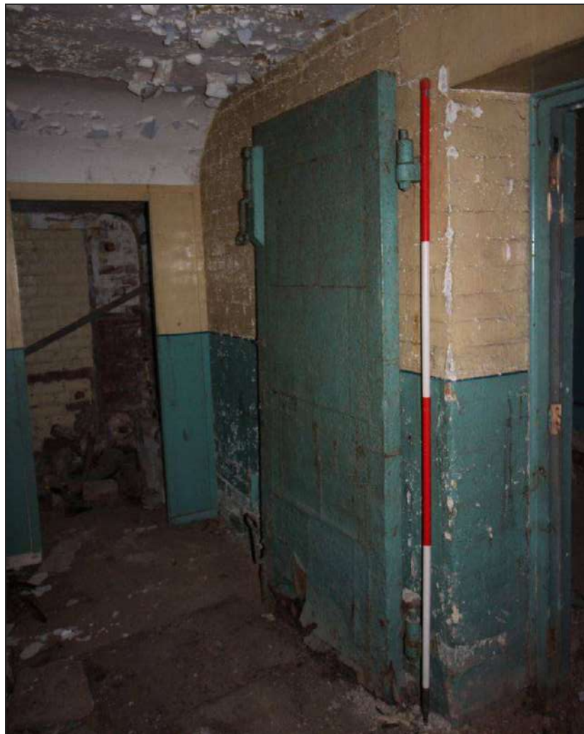
Plate 38: Vestibule at base of north-west stair tower with door into basement and room
