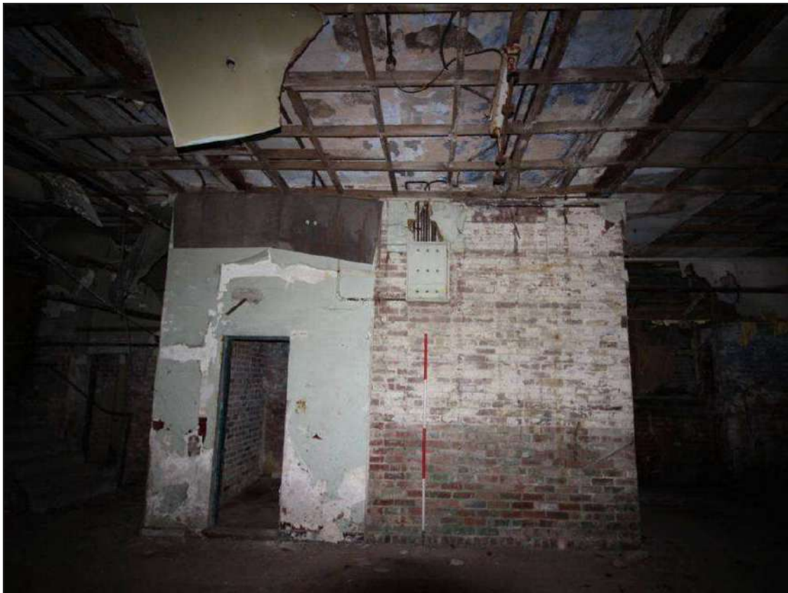
Plate 53: The small vestibule leading into the boiler room within the basement
