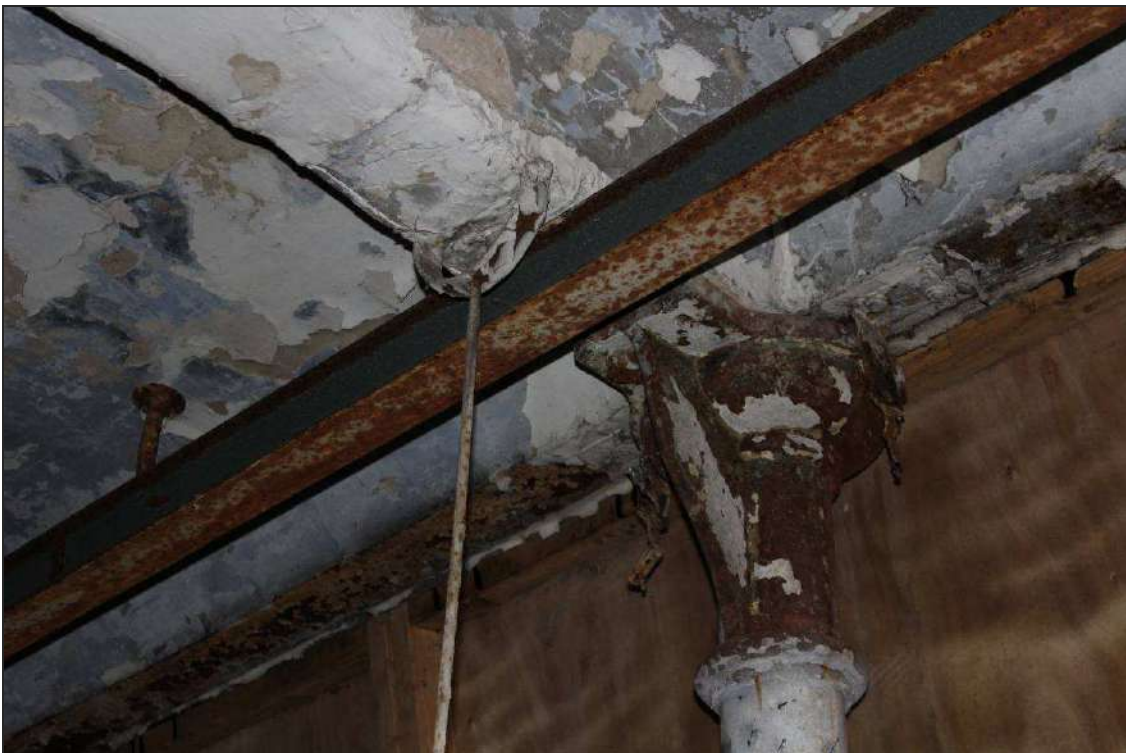
Plate 88: Detail of column capital and beam jointing by north wall of upper floor
