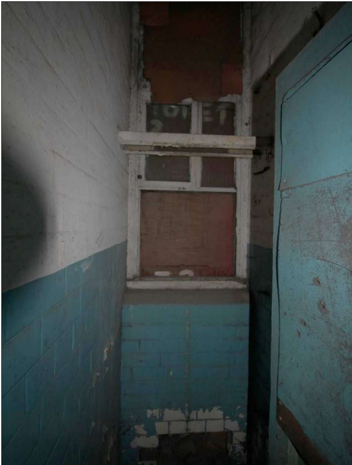
Plate 69: The blocked window and cistern rails within the northern privy tower on the first floor
