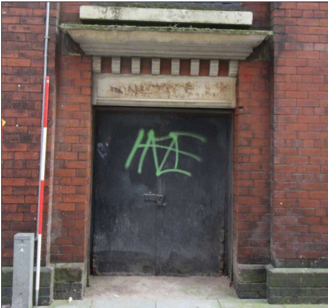
Plate 22: Detail of the doorway at basement level of the stair tower
