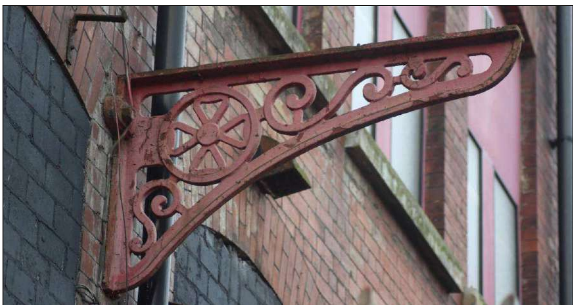
Plate 30: Detail of the cast-iron brackets of the fire escape
