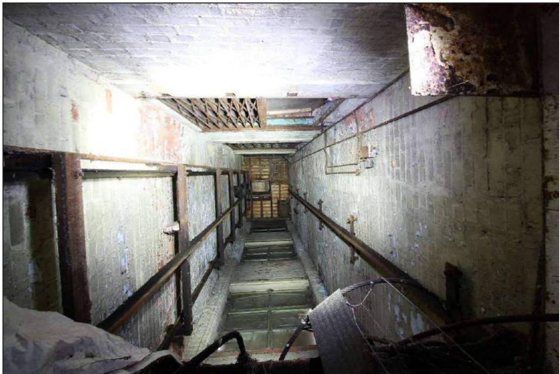
Plate 37: Internal view of the hoist tower
