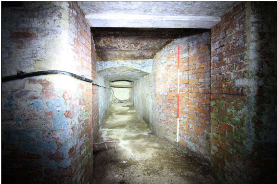
Plate 39: Original tunnel from Little Mill to New Mill within basement
