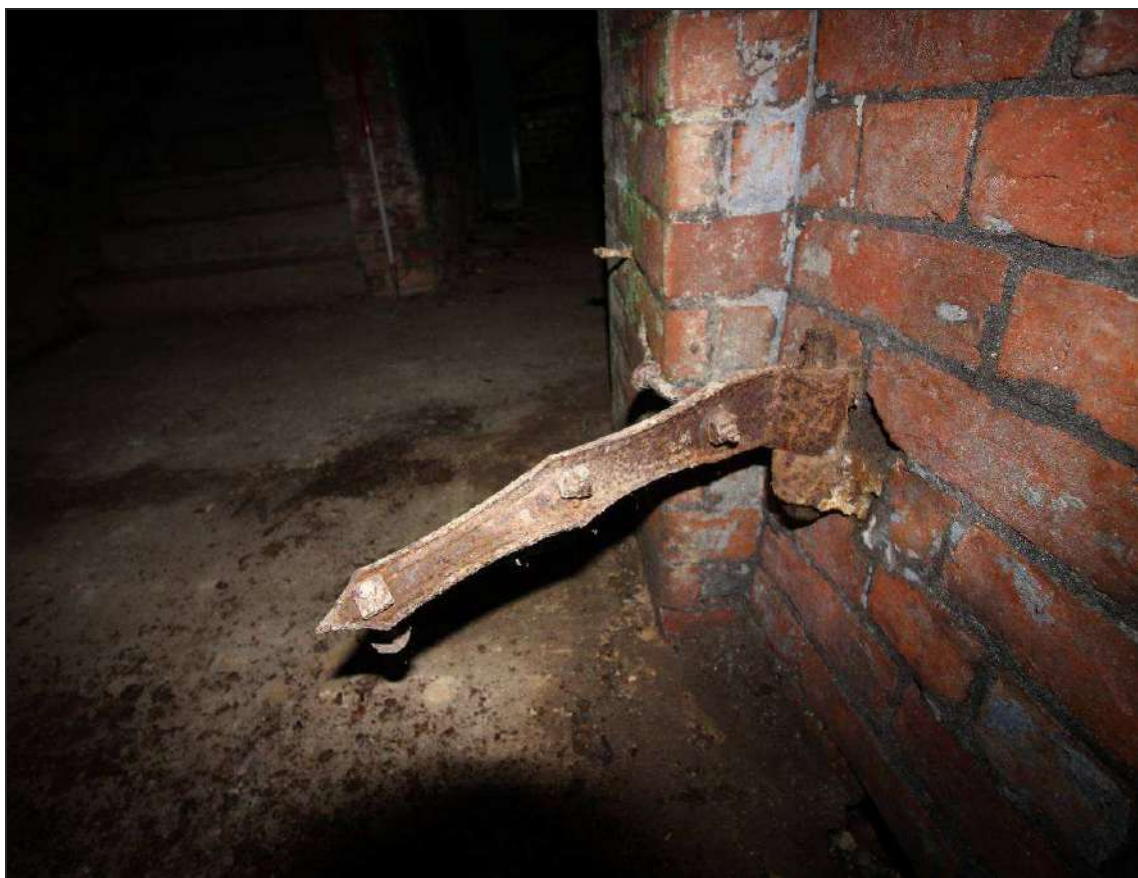
Plate 40: Detail of the remains of the hinge for the door of the north-west tunnel
