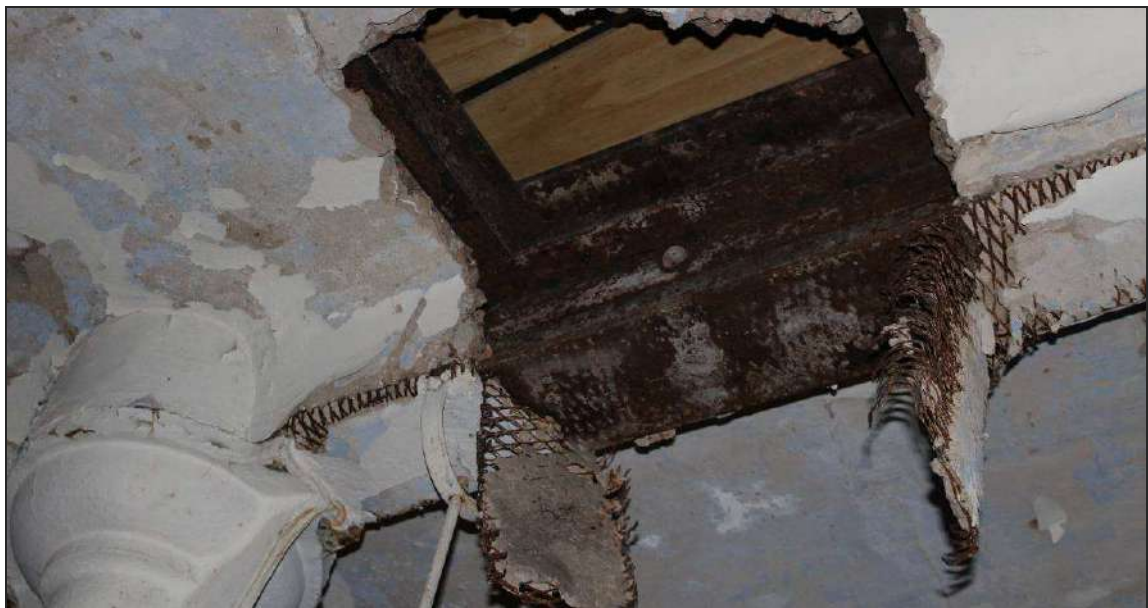
Plate 77: Detail of concrete and I-beam ceiling construction
