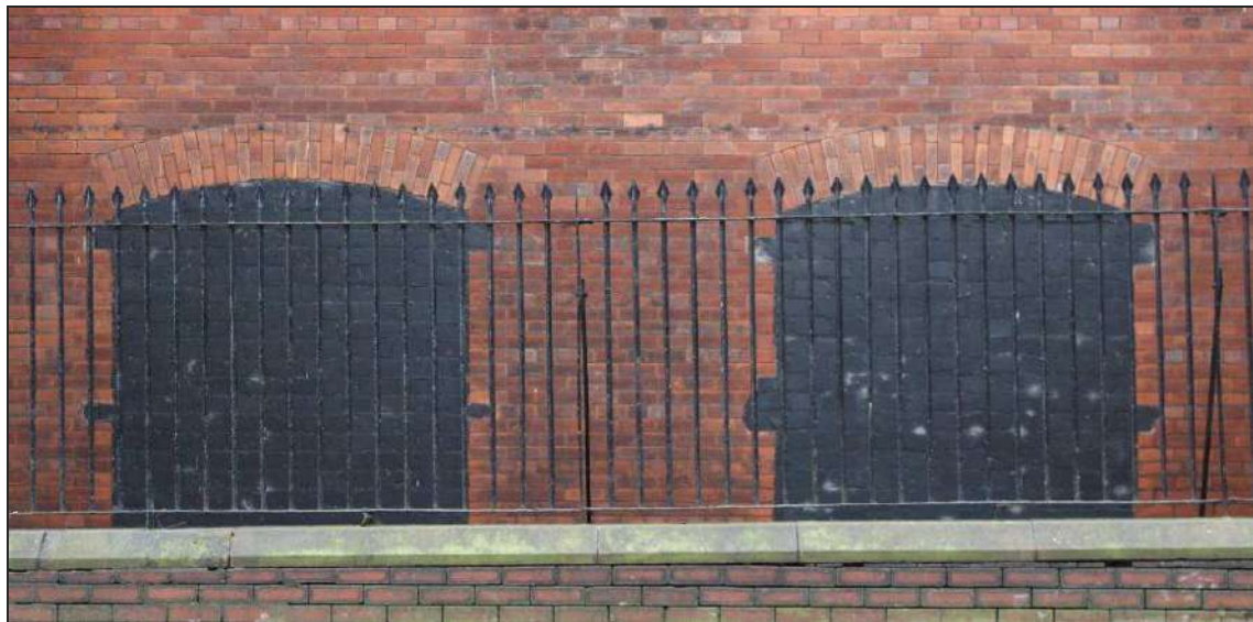
Plate 16: Detail of the blocked windows of the lower ground floor
