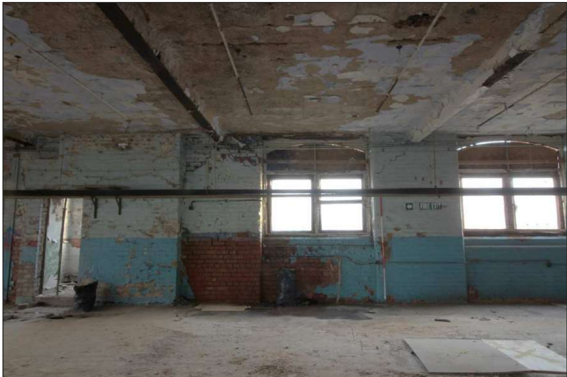
Plate 86: Windows on the third-floor, and remodelled entrance into later privies
