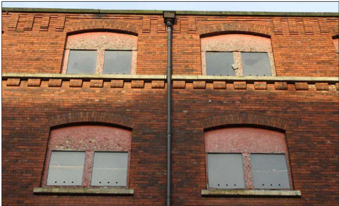
Plate 25: Detail of the upper-floor window apertures and parapet
