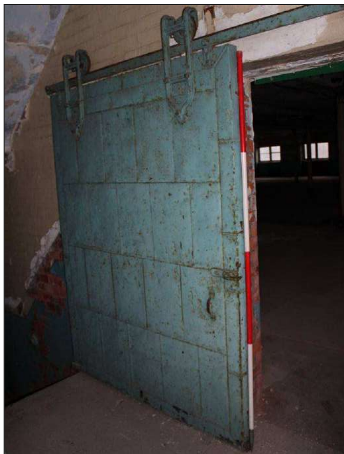
Plate 63: Detail of fireproof sliding door
