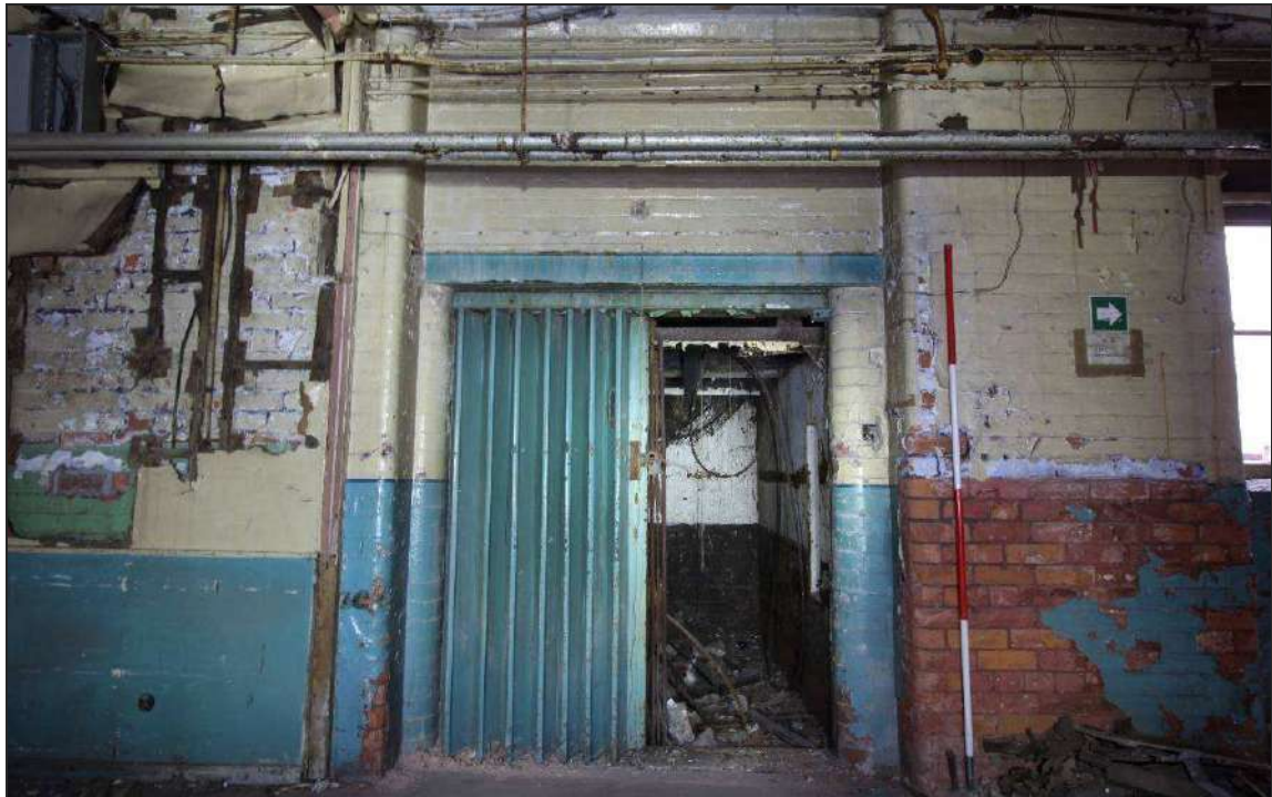
Plate 36: The doorway of the former motor tower at upper ground floor level
