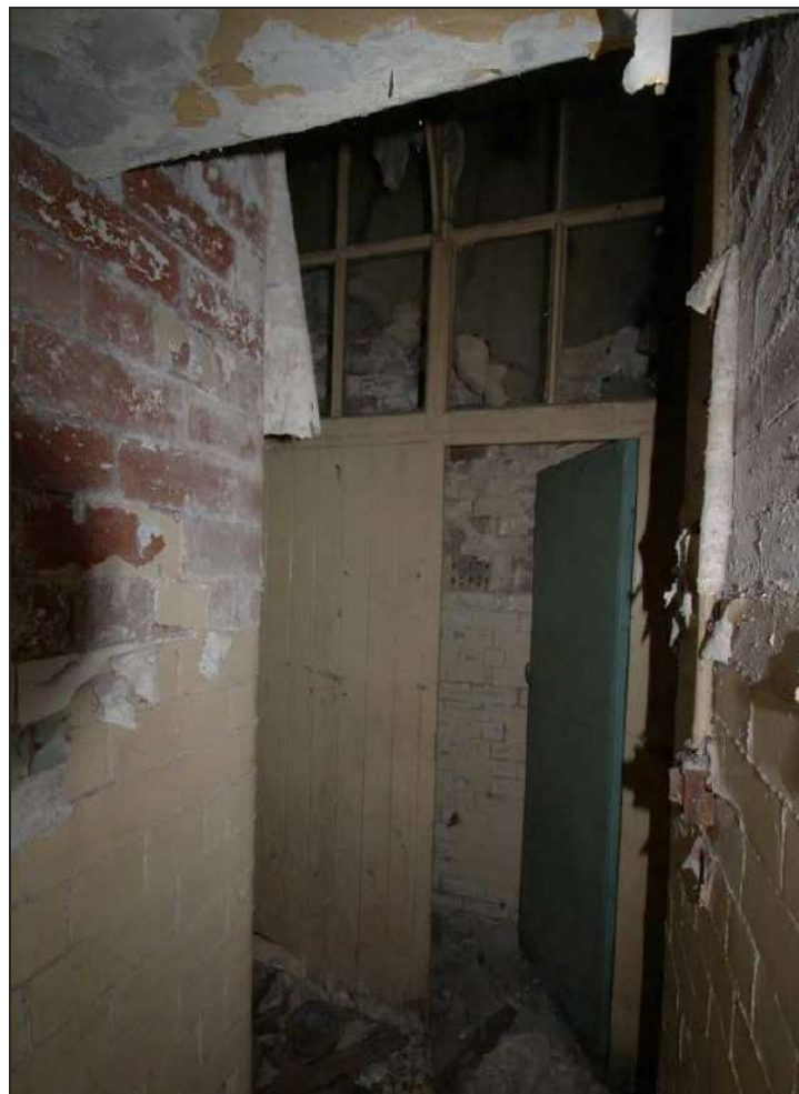
Plate 52: Timber partition within basement privy
