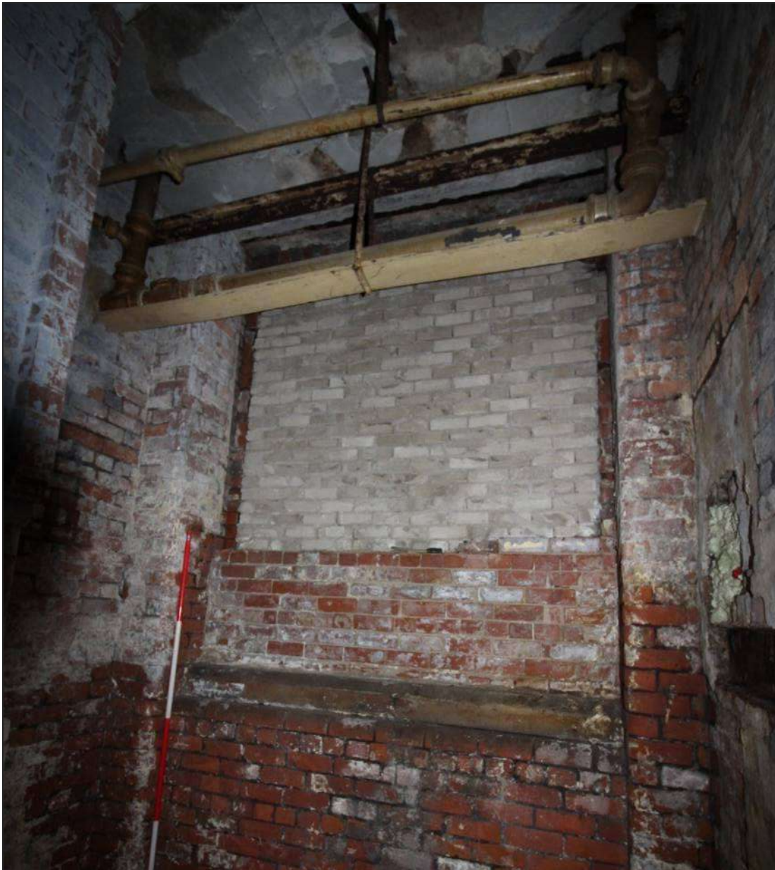
Plate 56: Blocked window in the south wall of the secondary tower
