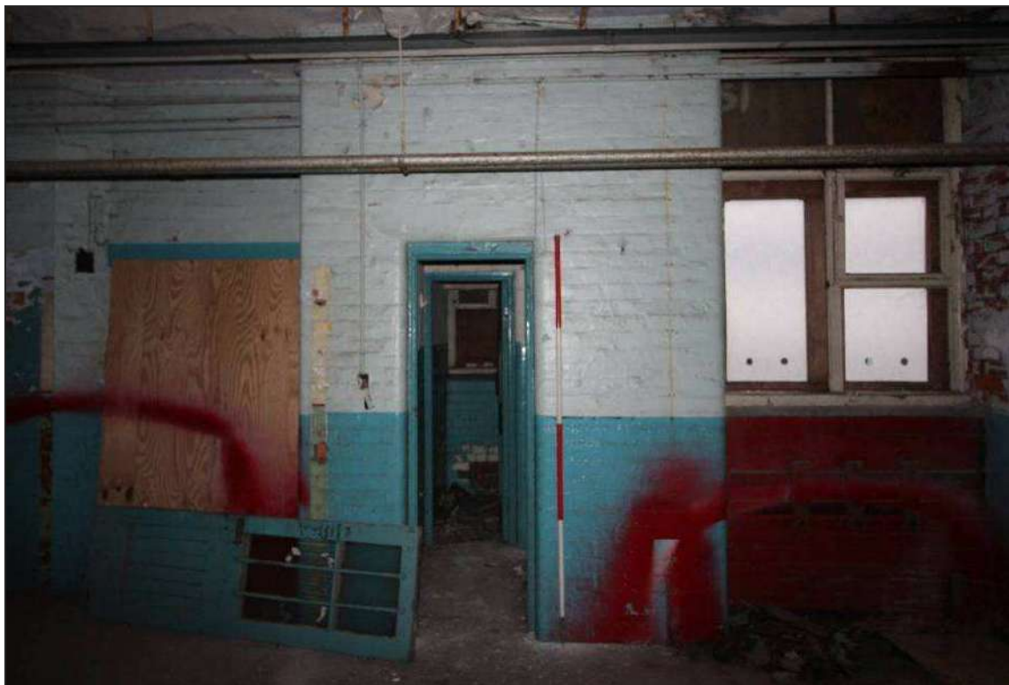
Plate 68: Doorway into original privy tower with blocked hoist to left
