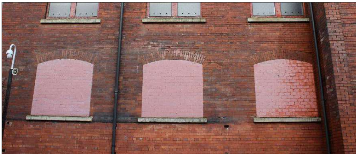
Plate 24: Detail of blocked windows to the ground floor
