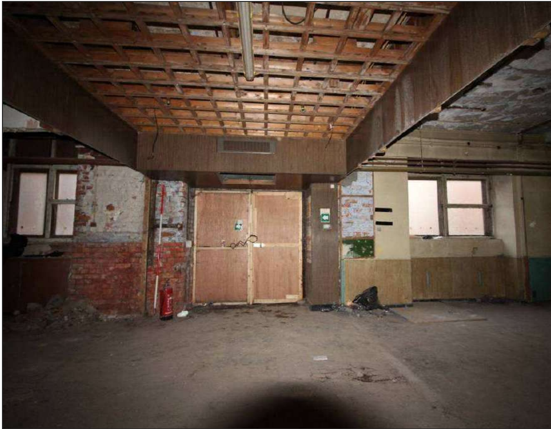
Plate 34: Principal doorway into the mill in the northern wall, with ceiling of vestibule
