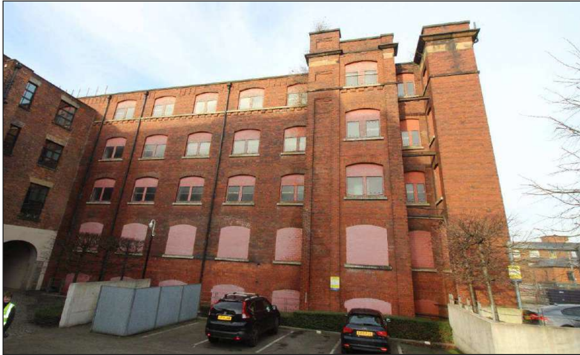
Plate 23: General view of the southern façade
