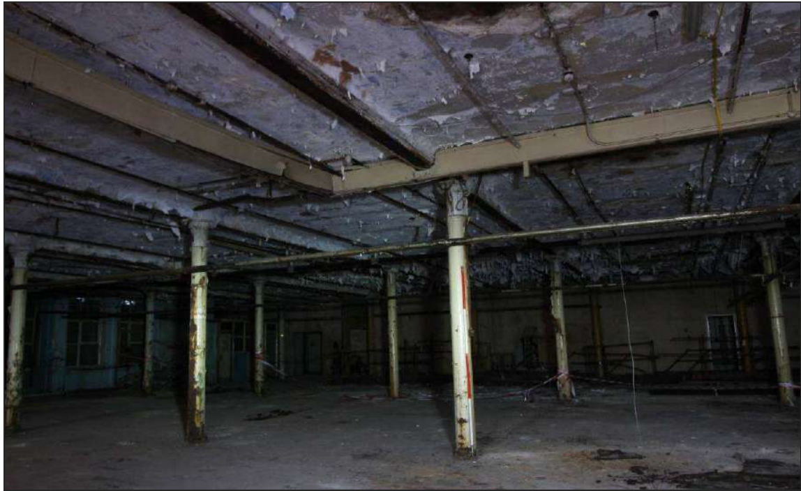
Plate 32: General view of the ground floor, detailing the cast-iron column arrangement
