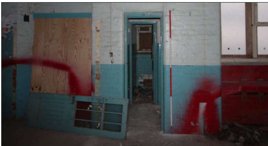
Plate 79: Northern privy and blocked hoist tower, with original doorway lying nearby
