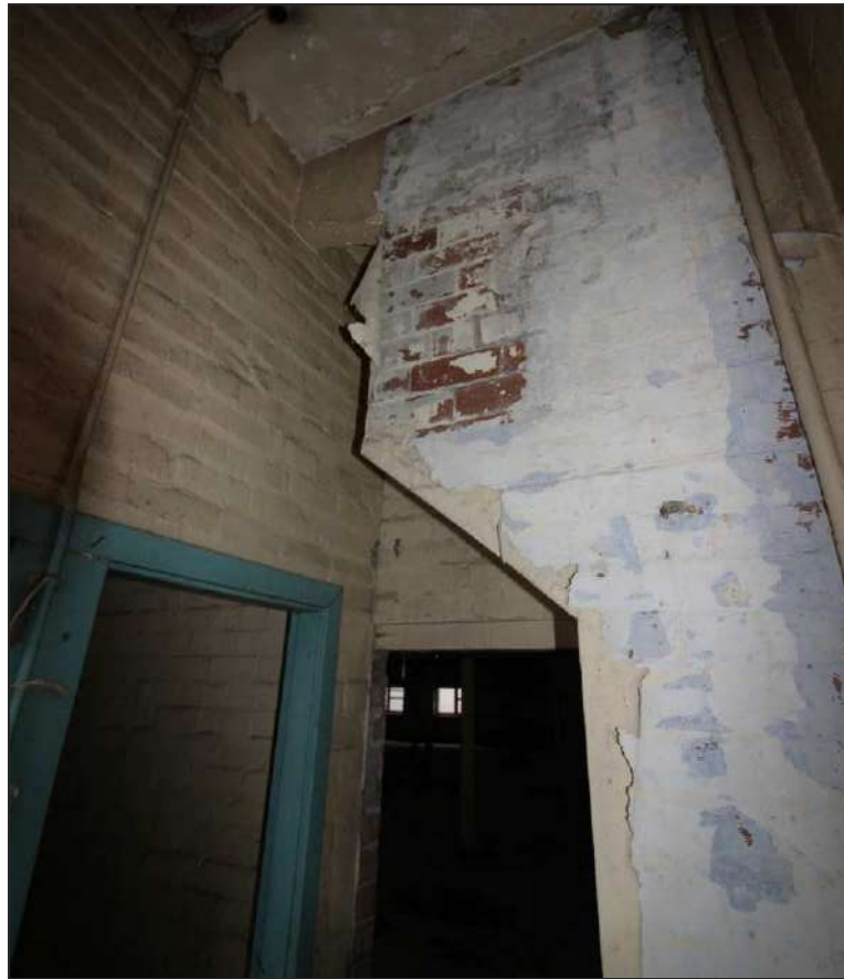
Plate 71: Cutaway east jamb of original window with cubicle wall respecting original lintel arch
