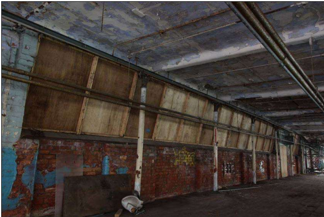
Plate 87: Glazing band within the north wall of the third-floor, with columns at each bay division
