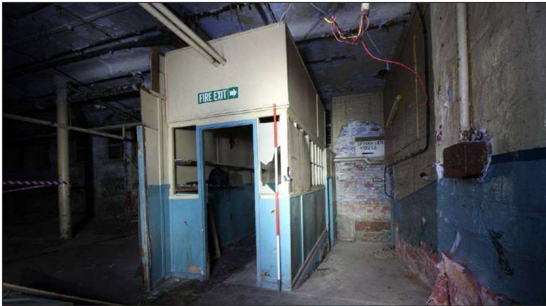
Plate 48: Timber-partitioned office with sprinkler system valve room to the rear
