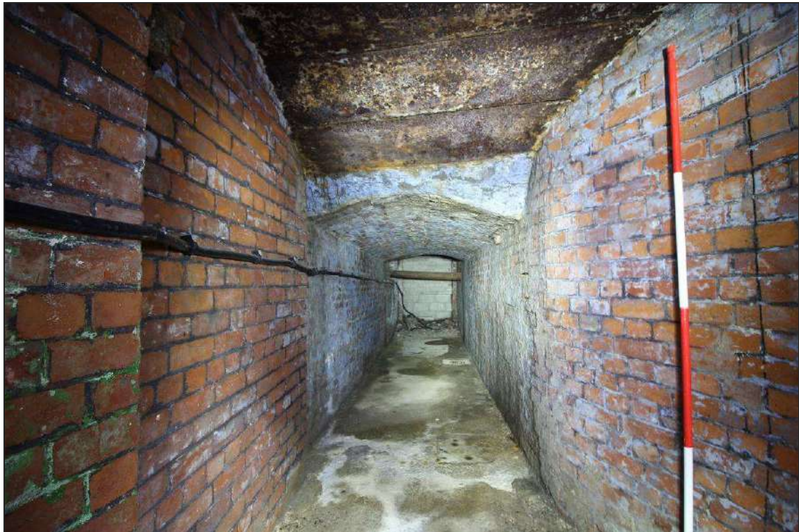
Plate 41: Detail of the phasing within the northern tunnel
