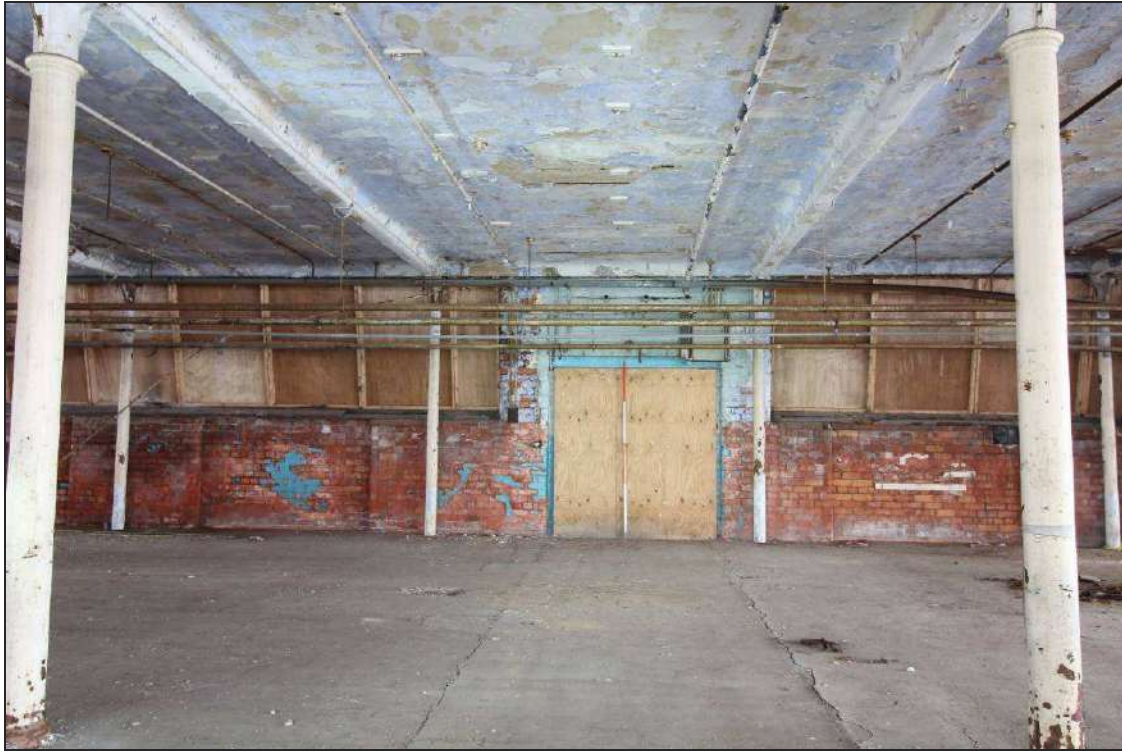
Plate 91: Blocked doorway of the motor tower, with scars for possible power transfer brackets in the ceiling
