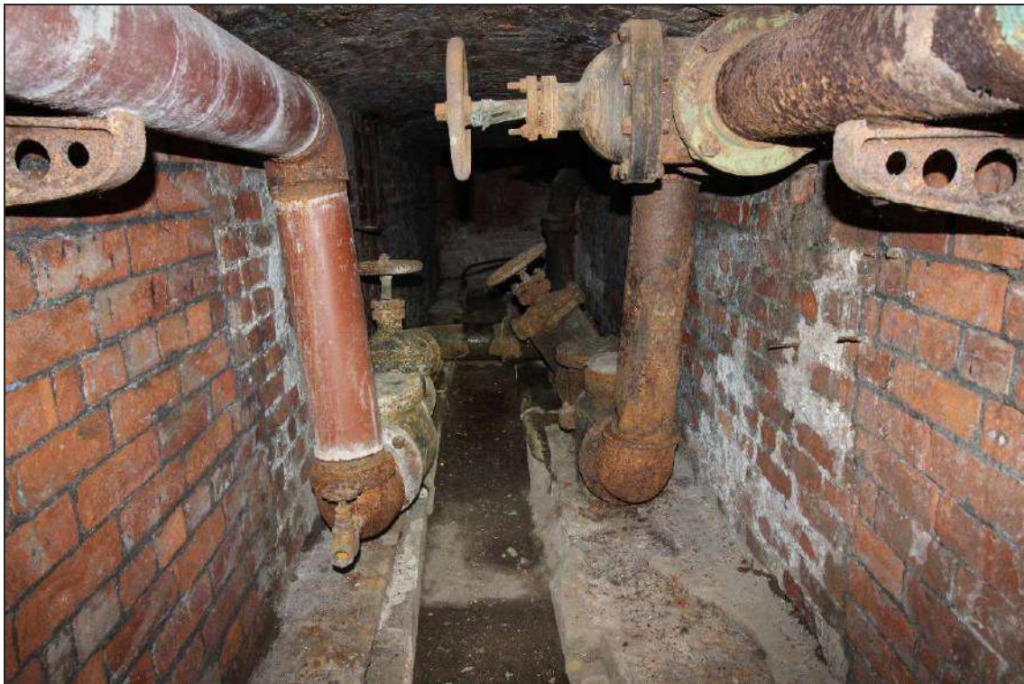
Plate 45: General view of the service tunnel, detailing the channel within the floor
