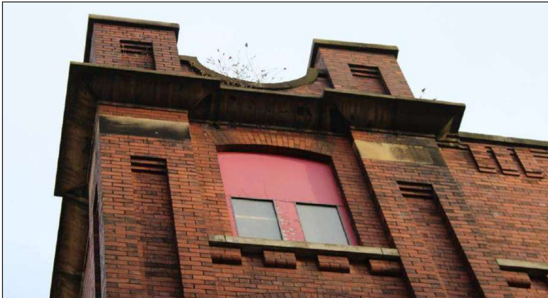
Plate 21: Detail of the parapet wall of the stair tower, and corbels to the parapet to the south
