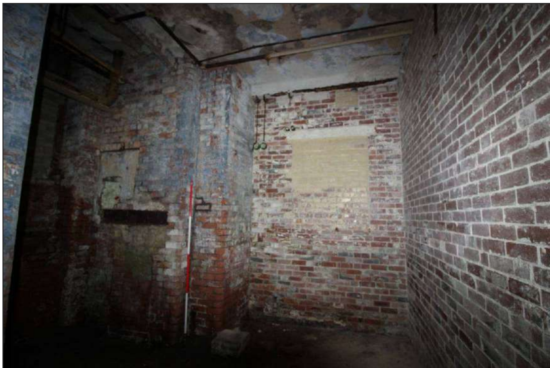
Plate 54: Detail of the blocked window within the south-west wall of the inserted room
