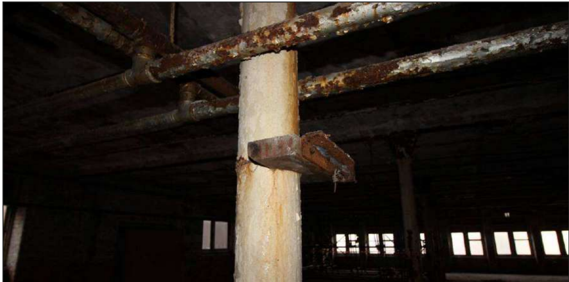
Plate 78: Detail of an attached bracket to the north-west column
