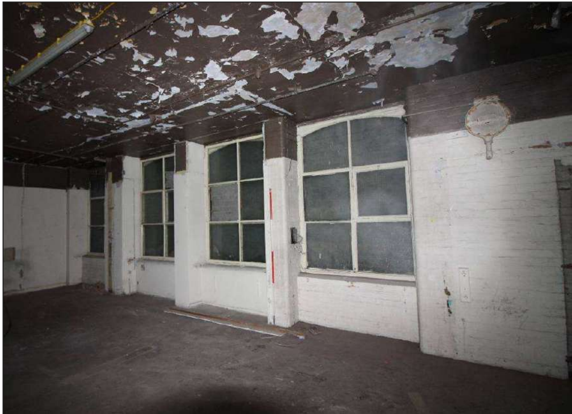
Plate 35: Recessed windows in end wall of upper ground floor, with original timber window frames, late partition wall (left) and fire alarm valve (right)
