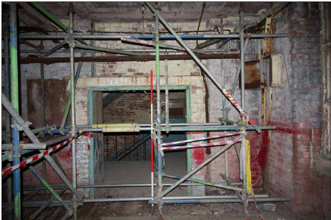
Plate 74: Doorway into the late stair tower at first-floor level
