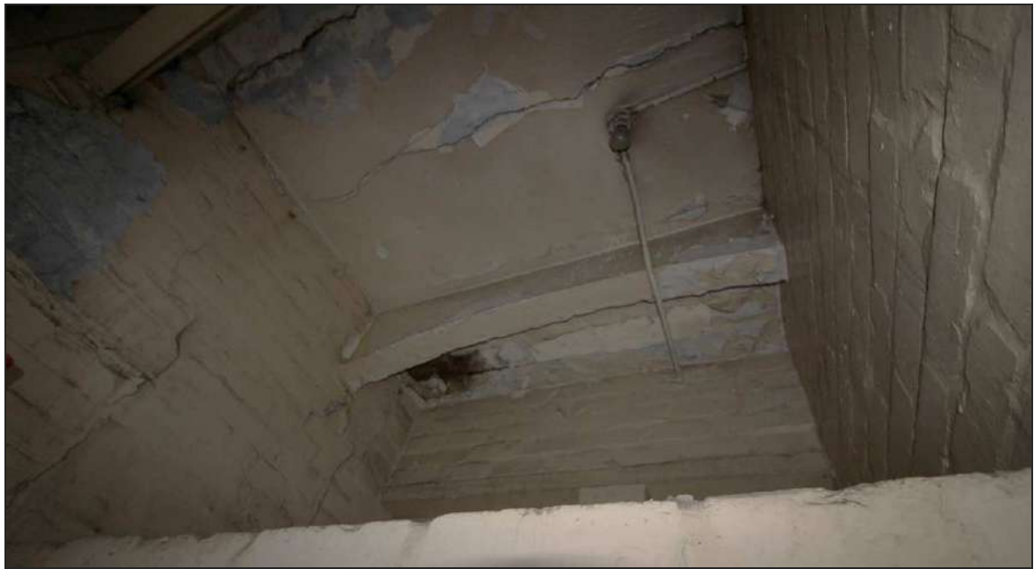
Plate 73: Detail of retained arched head of original window, with inserted cubicle wall on right
