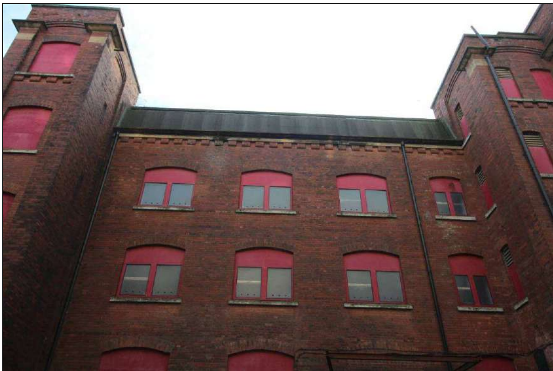
Plate 15: Detail of the windows on the upper-floors and roof structure
