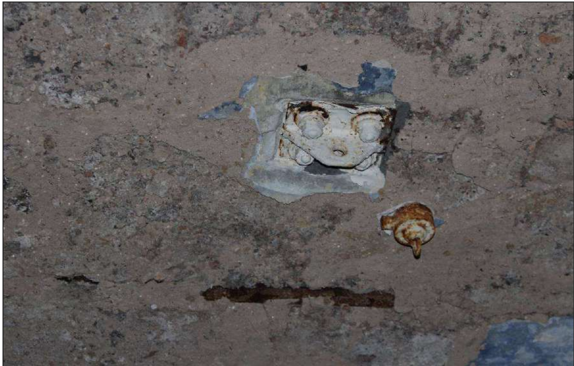
Plate 67: Detail of a cast-iron eye-bracket bolted into the ceiling of the first-floor
