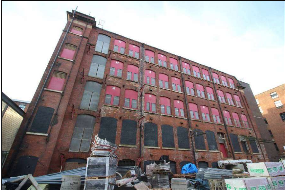
Plate 28: General view of the north-east façade
