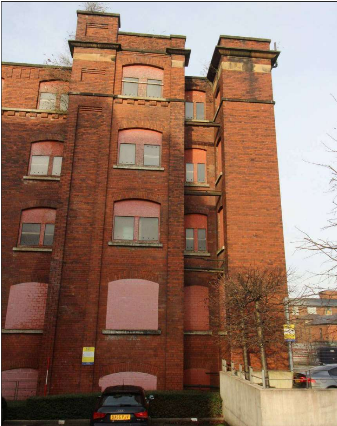
Plate 27: General view of privy tower and later ventilation and humidification tower
