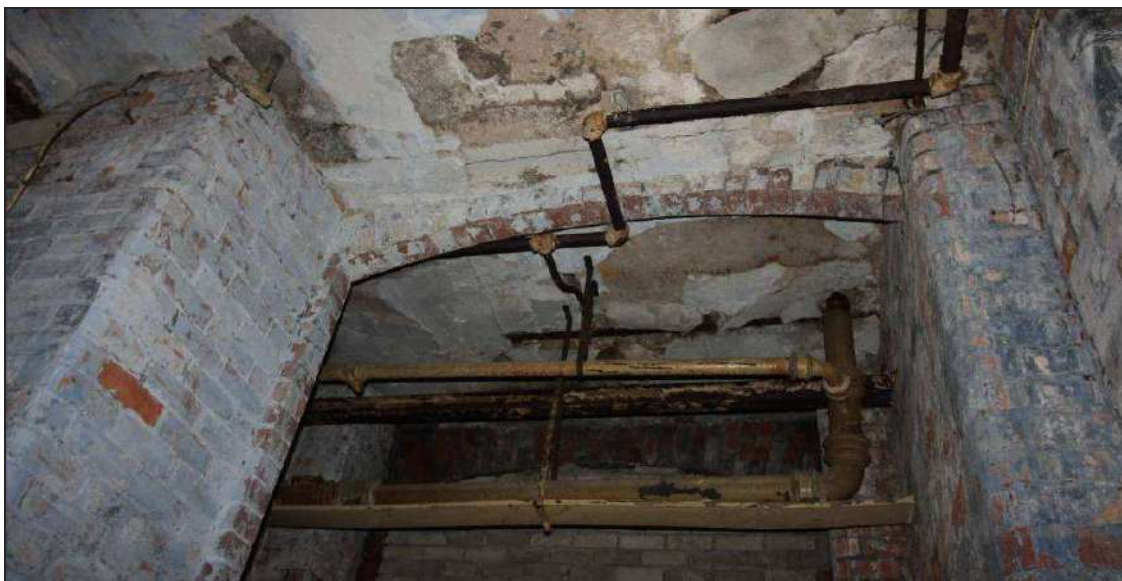
Plate 55: Remains of the segmental arch head of the earlier window within the basement
