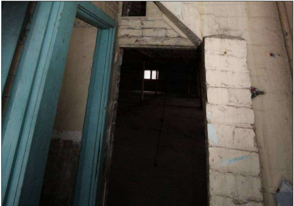
Plate 80: Detail of the remodelled entrance into ventilation and humidification tower
