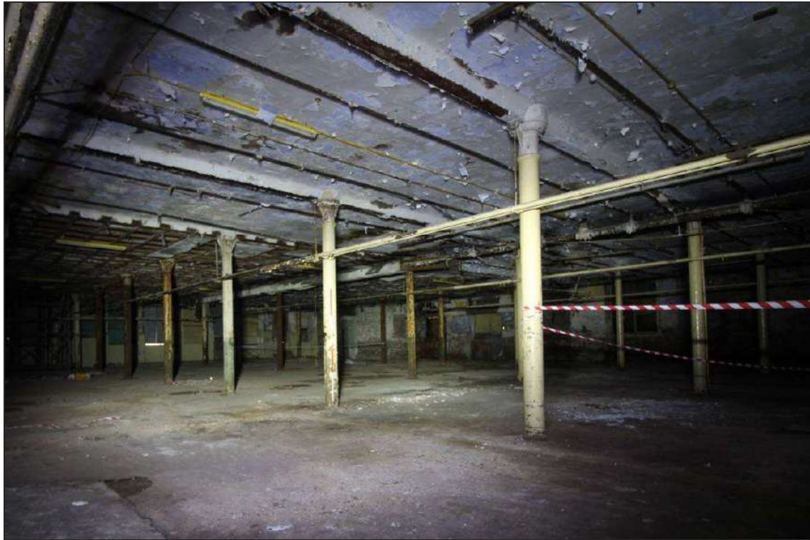
Plate 43: General view of the lower ground floor
