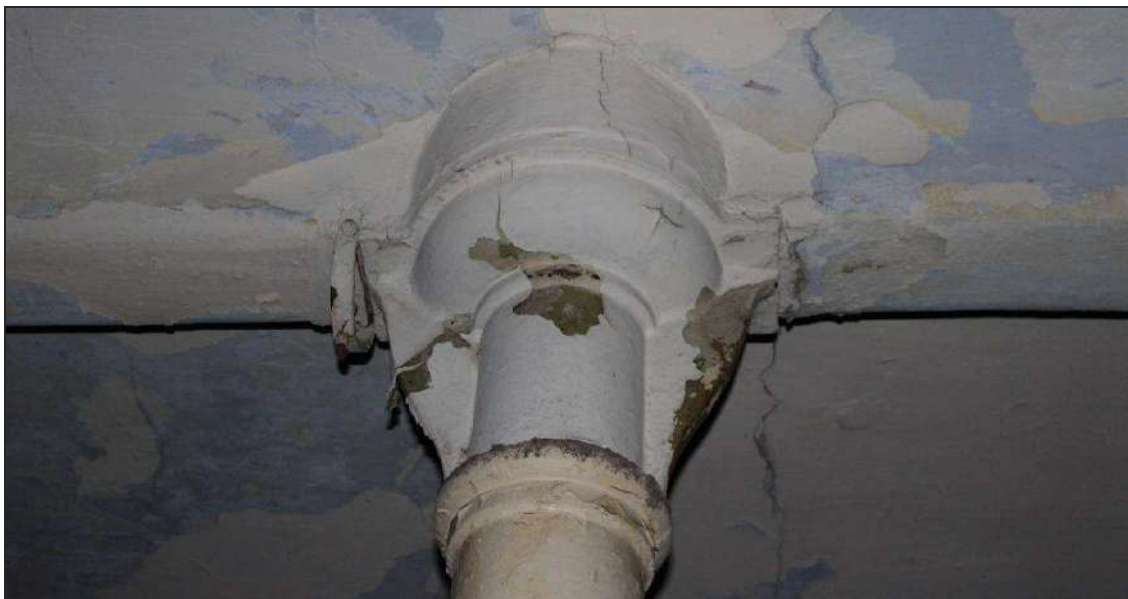
Plate 65: Detail of column capital
