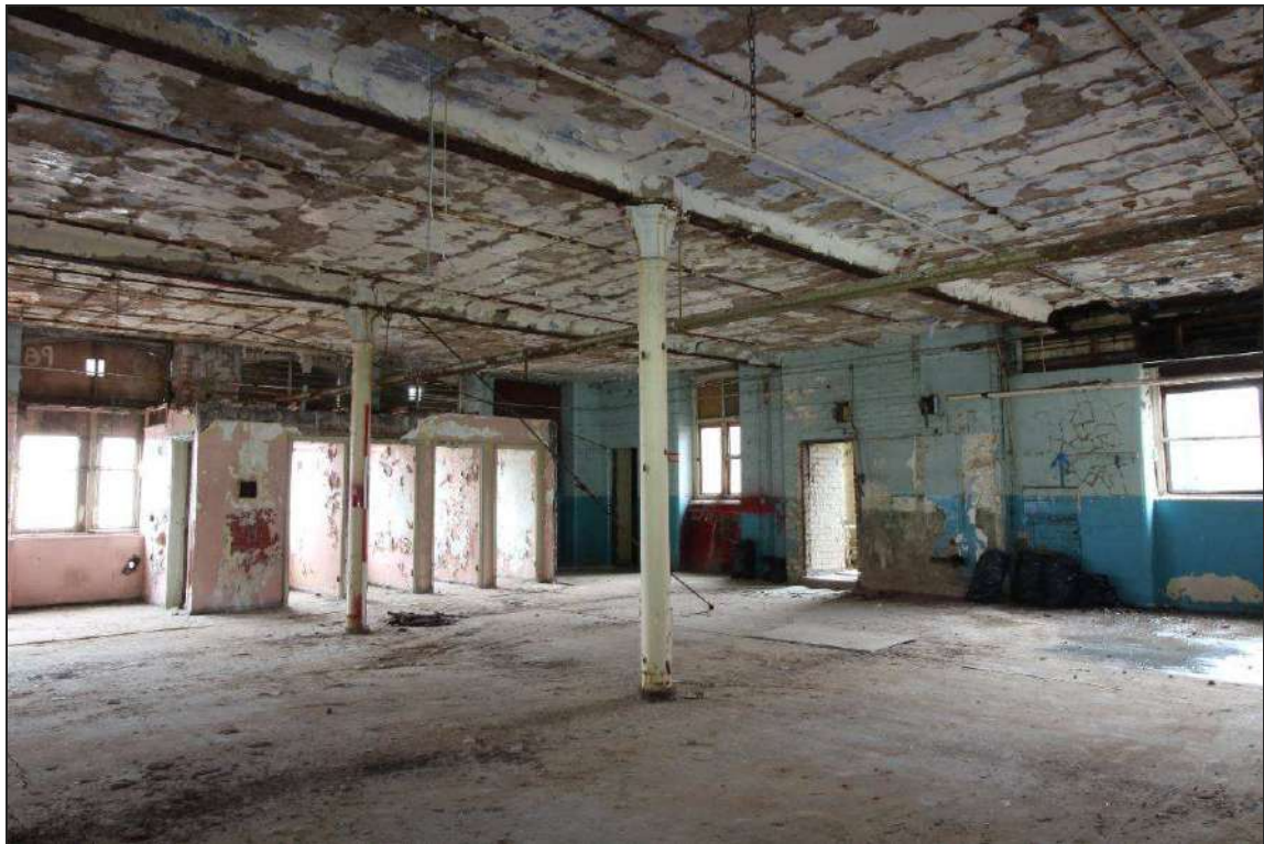
Plate 76: Detail of the columns on the second-floor
