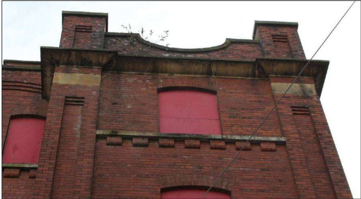
Plate 13: Detail of upper stair tower
