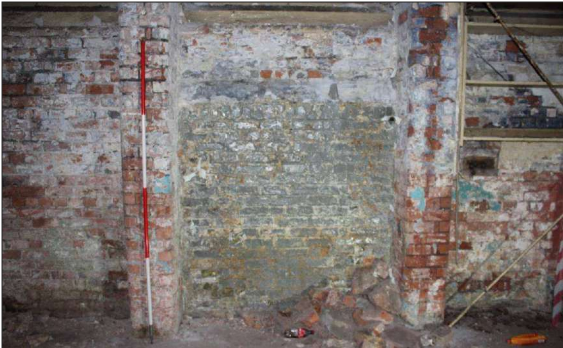
Plate 51: Blocked entrance into the southern tunnel below Bengal Street
