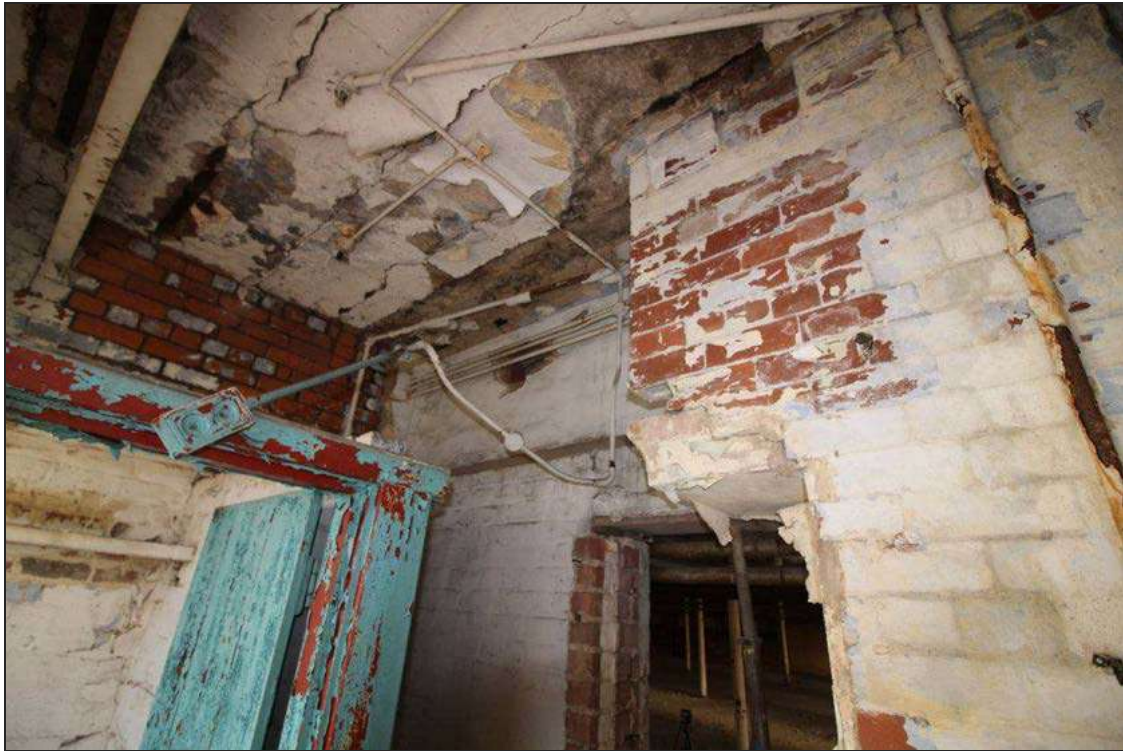
Plate 90: Detail of the removed external lintel arch of the original window aperture
