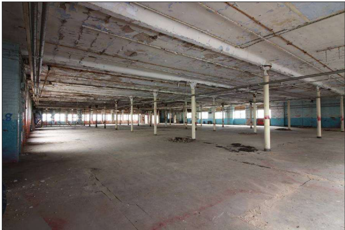
Plate 75: General view of the second floor
