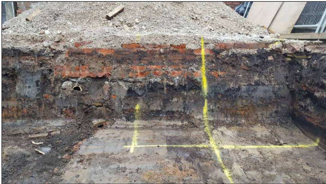
Plate 98: Wall 002 exposed in the north section of the excavated trench
