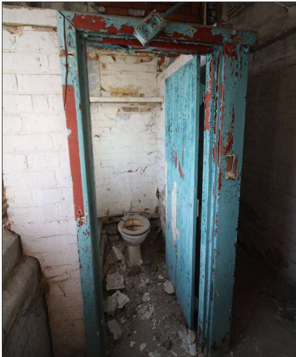
Plate 89: Toilet cubicle with wall scar for cistern within the later privy on the third floor
