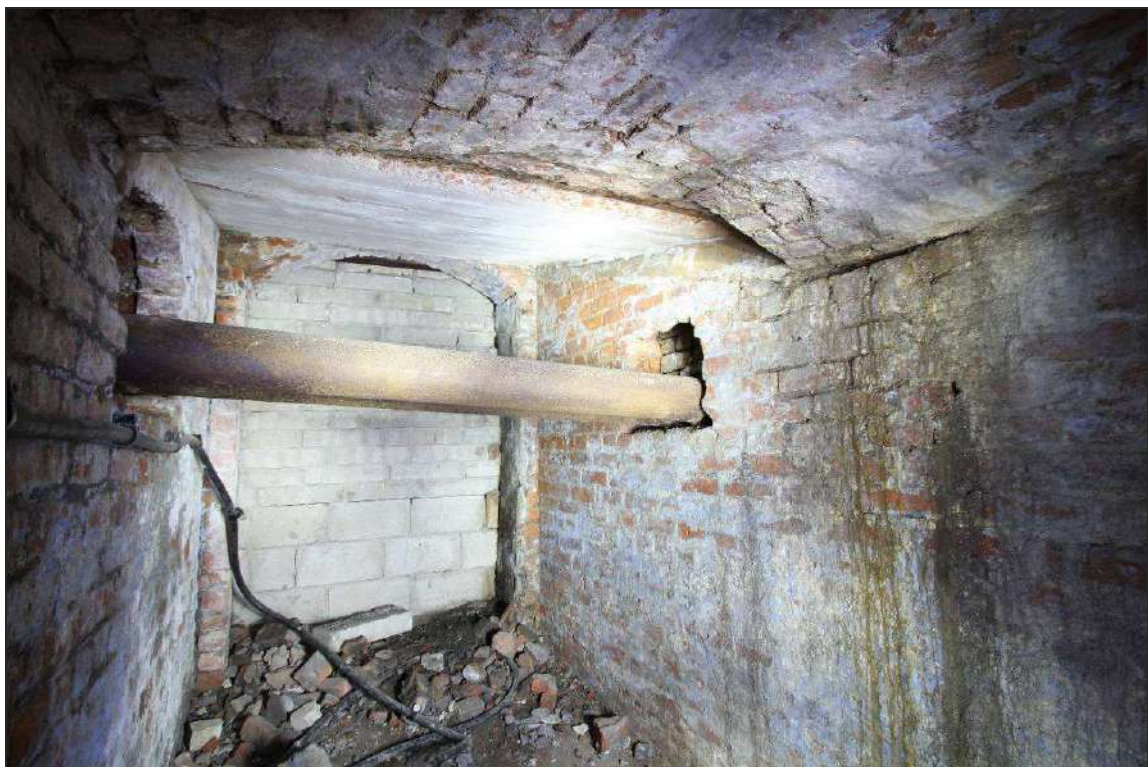
Plate 42: Blocked doorway into the basement of New Mill and inserted water main pipe
