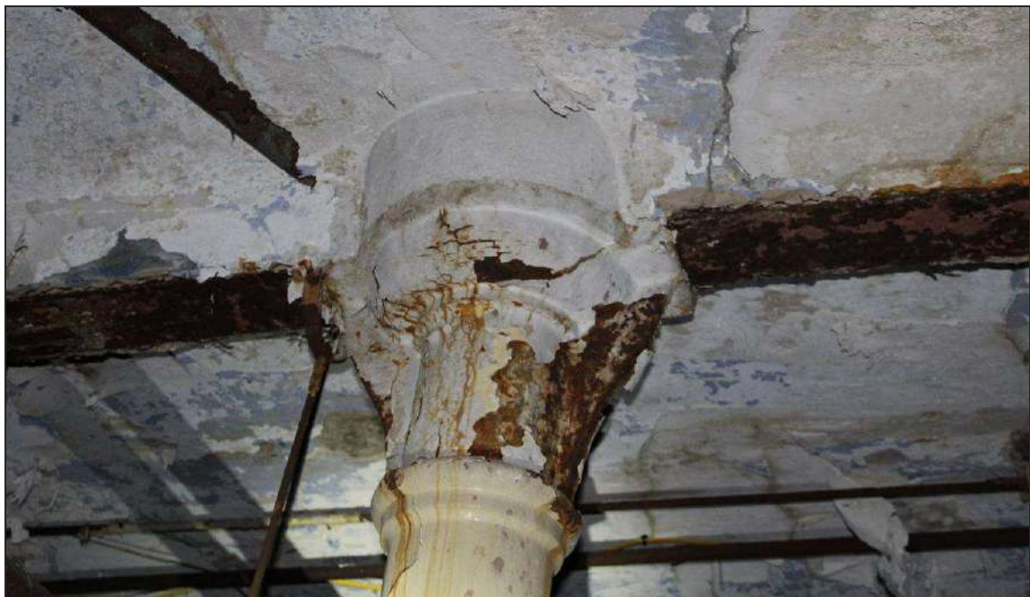
Plate 33: Detail of the astragal capital of the columns on the ground floor
