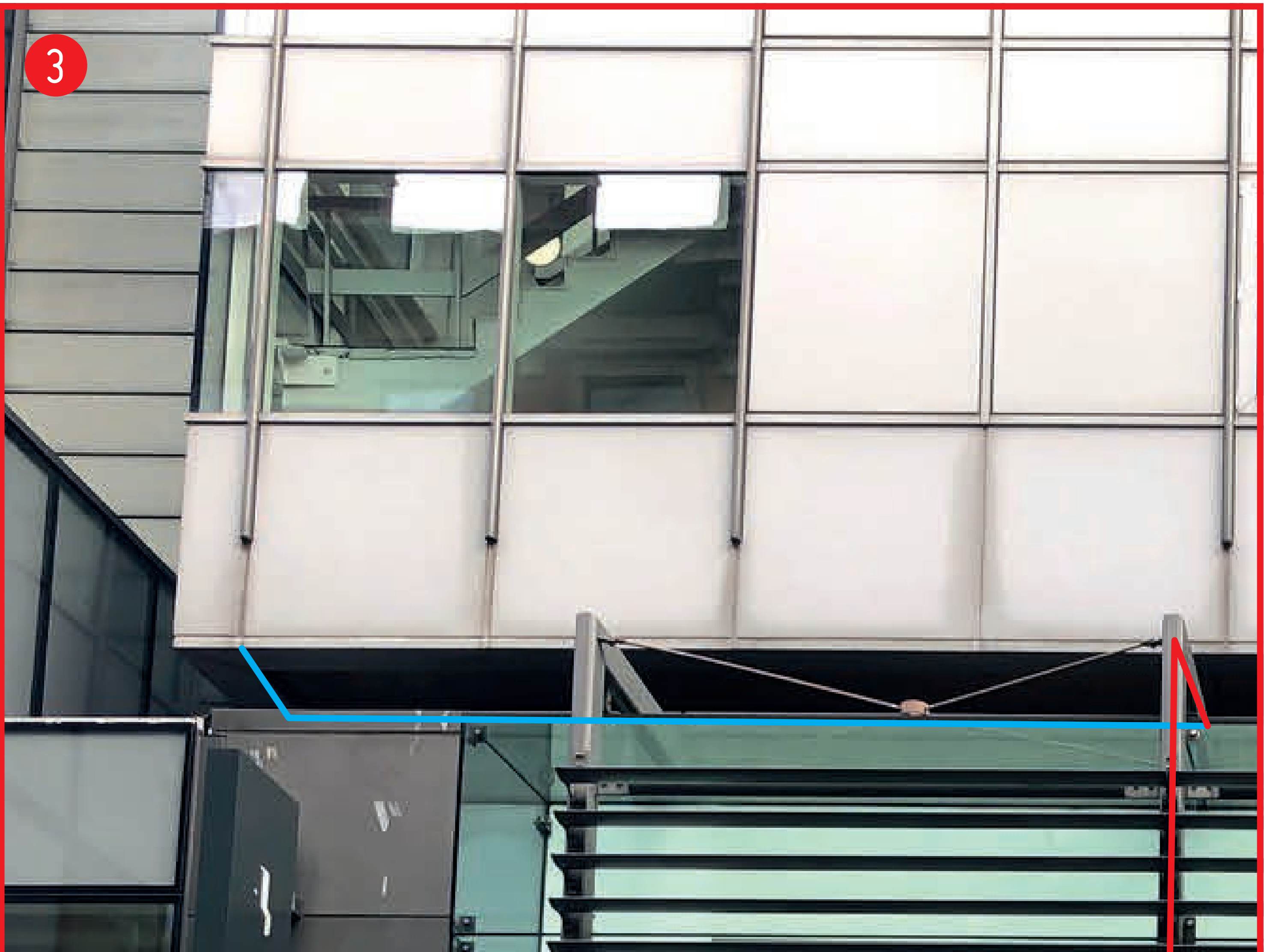
3 FEED IS TO THEN RUN ACROSS THE ROOF TO A WINDOW, AND FED THROUGH THE WINDOW TO A FUSED SPUR ON THE INSIDE OF THE BUILDING
