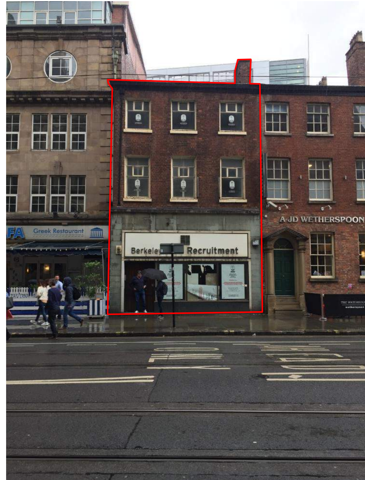
Figure 1 – Front elevation of 65 Princess Street
