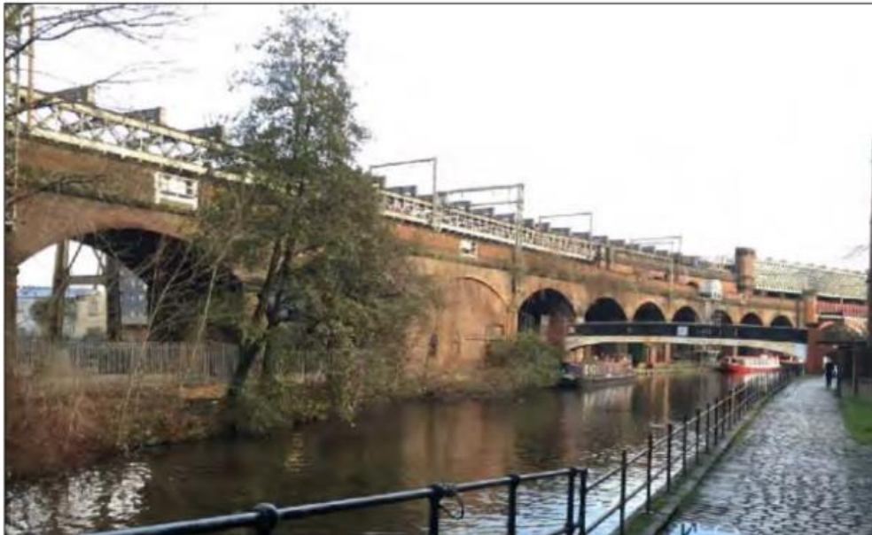
Figure 4.4: Manchester South Junction and Altrincham Railway Viaduct, viewed from the Bridgewater Canal towpath, looking north-east (December 2016)
