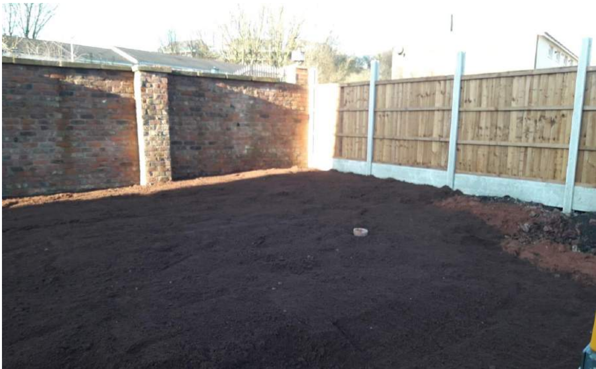
Photograph 6 Plot 1 after 200mm of topsoil emplaced overlying the subsoil and granular break layer.
