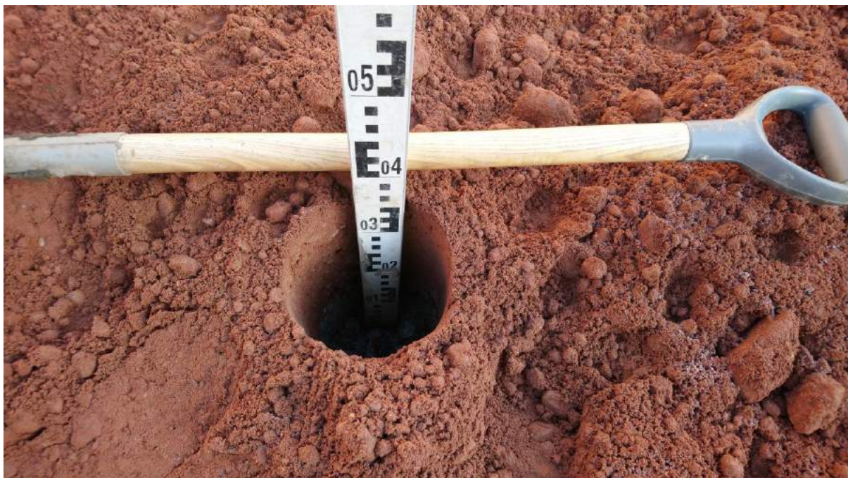
Photograph 4 Plot 1 showing 200mm of subsoil overlying a 200mm granular break layer, prior to the emplacement of the topsoil.
