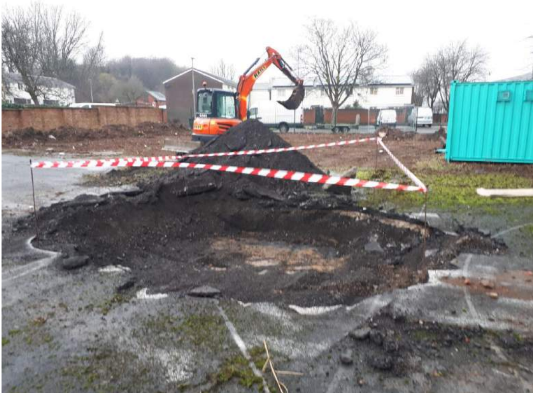
Photograph 1 Area of TP1 excavated to 0.60mbgl into the natural Alluvial Sand.
