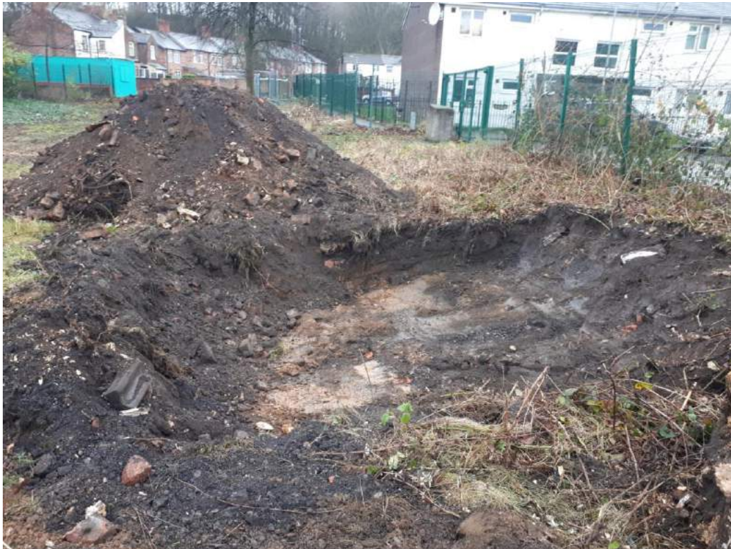
Photograph 3 Area of TP6 excavated to the top of the natural strata.
