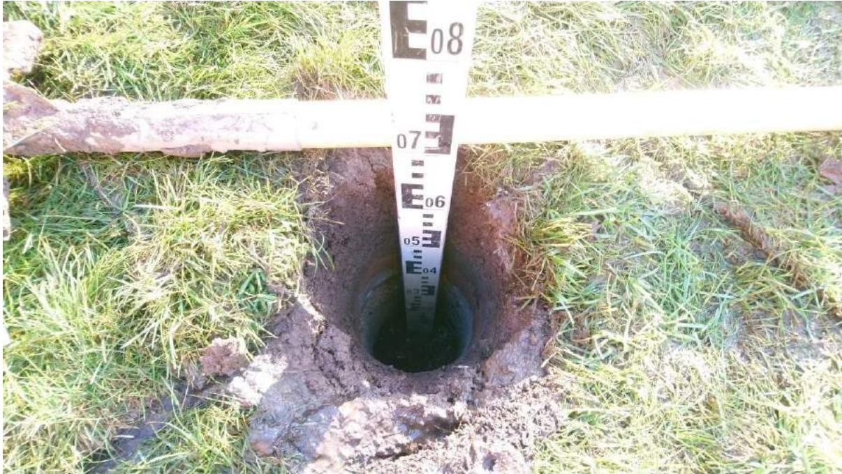
Photograph 7 Plot 5 showing 250mm of topsoil, 200mm of subsoil and a 200mm granular break layer.
