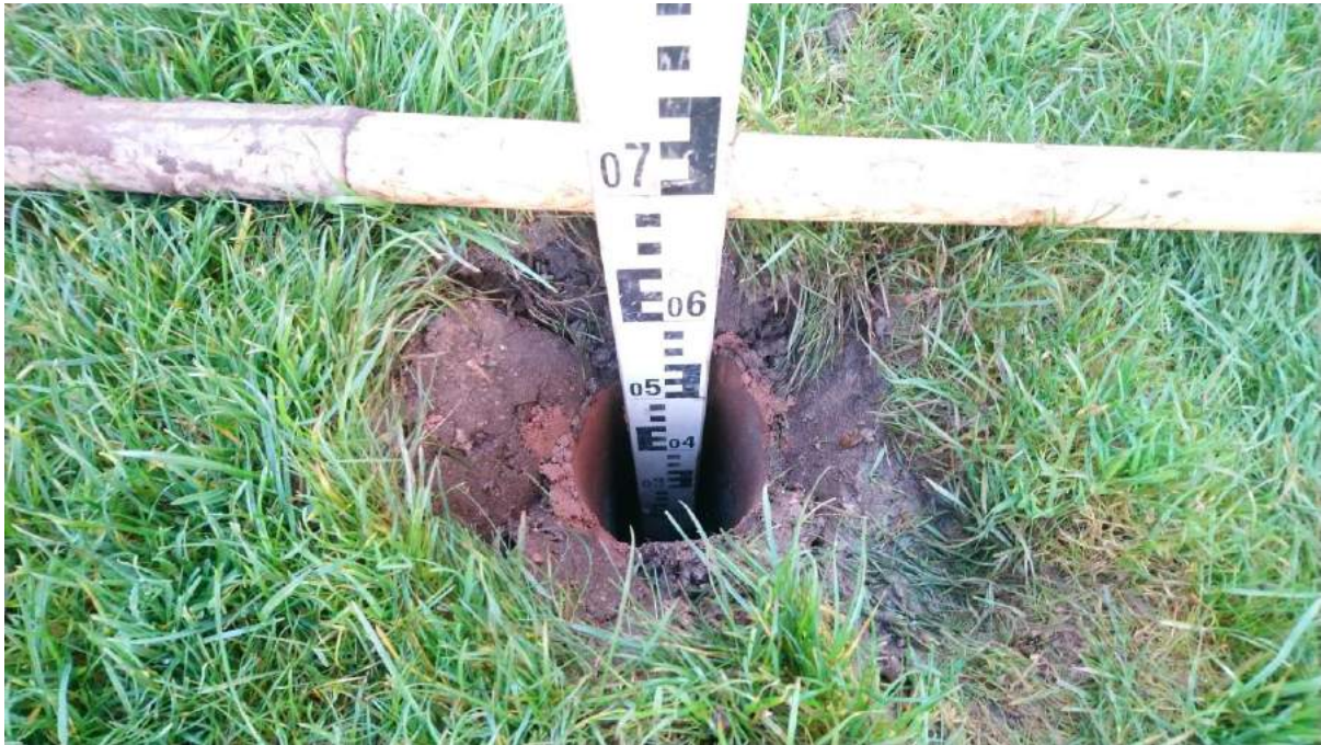
Photograph 11 Plot 10 showing 150mm of topsoil, 250mm of subsoil and a 200mm granular break layer.
