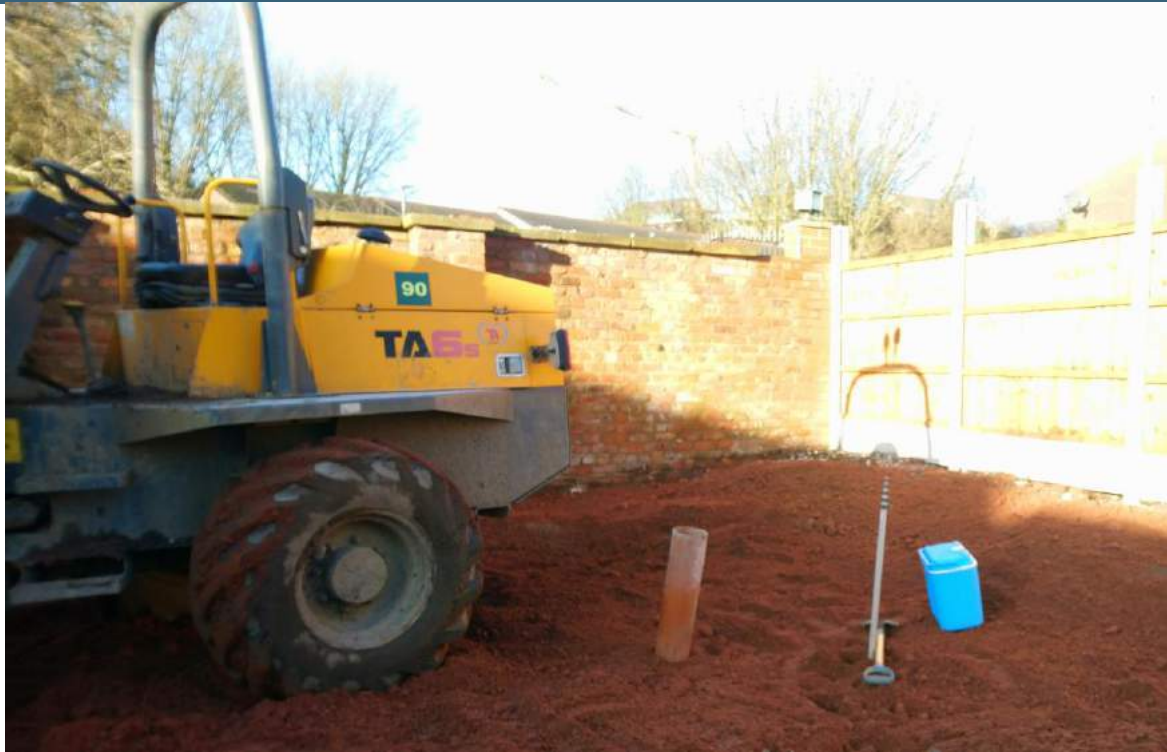
Photograph 5 Plot 1 showing pit location prior to the emplacement of topsoil.
