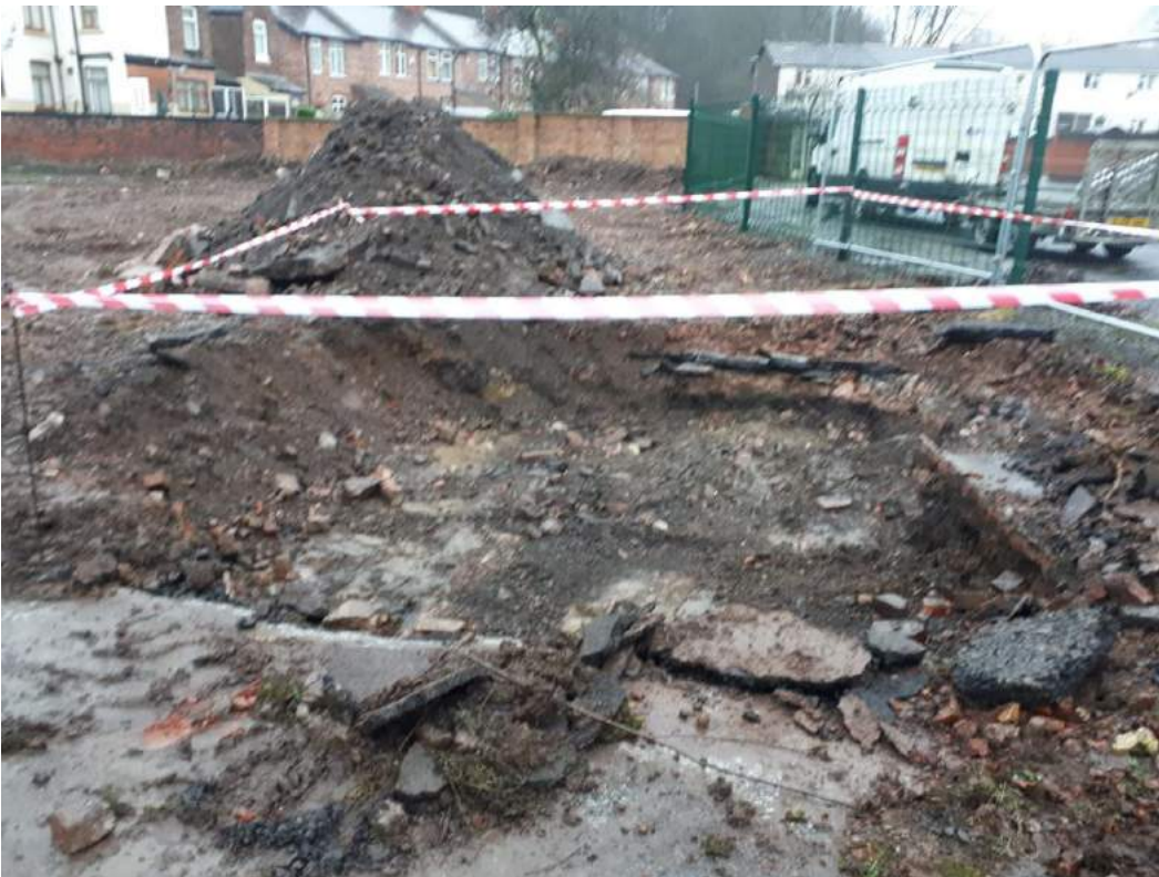
Photograph 2 Area of TP3 excavated to formation level.
