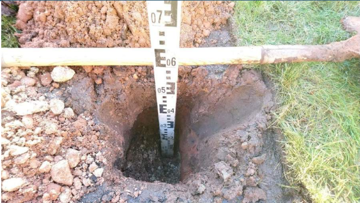
Photograph 9 Plot 7 showing 200mm of topsoil, 200mm of subsoil and 200mm granular break layer.
