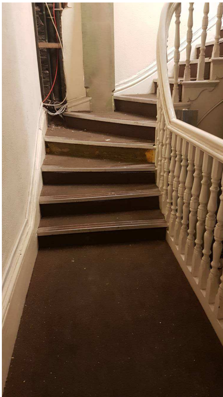
Image 8 – Ground to first floor stairs.
