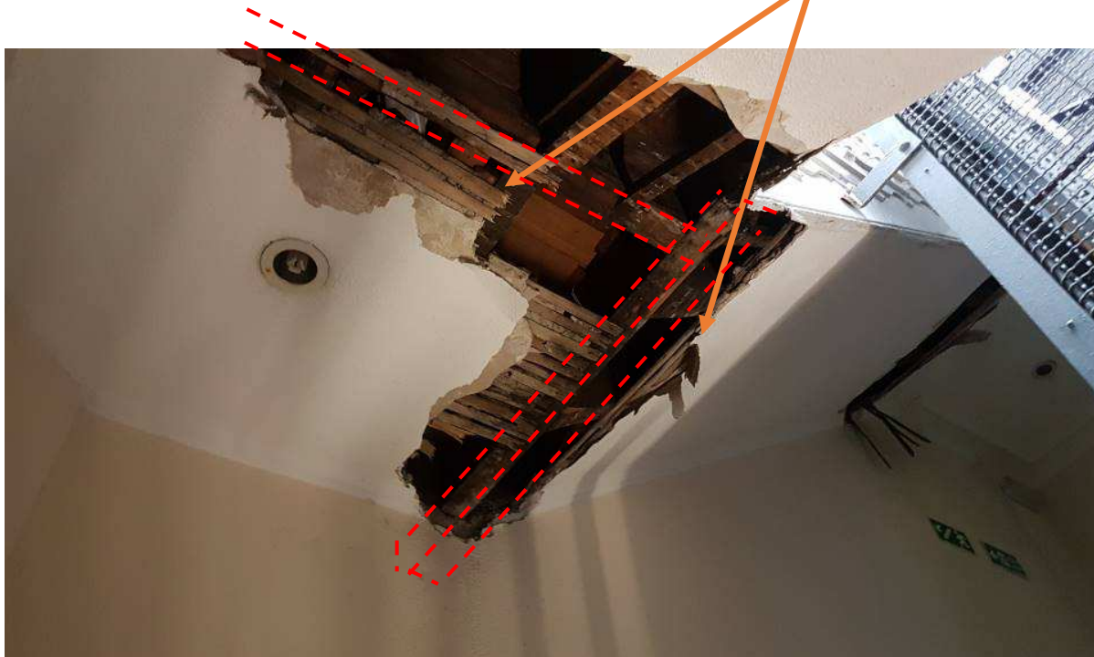
Image 5 – Existing Supporting cantilevered half landing.
