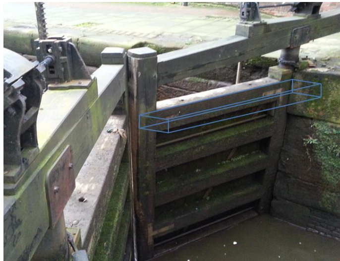
Detail of load transfer beam
