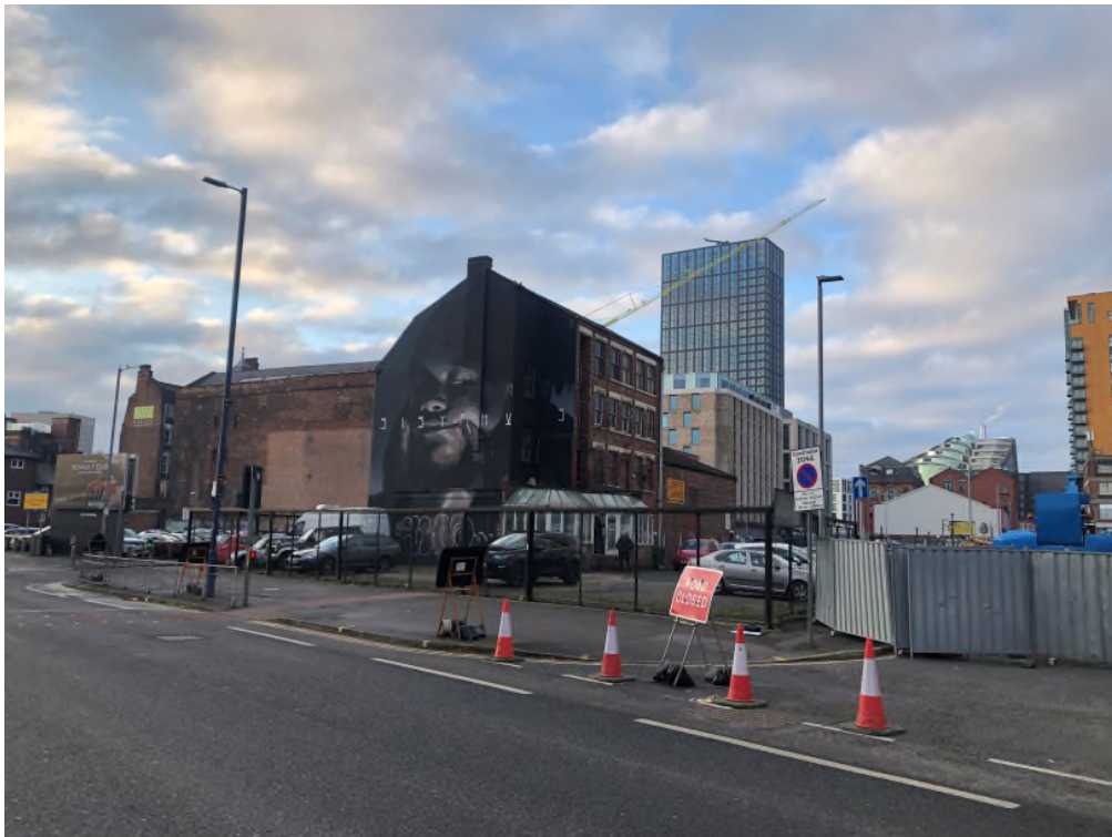
Oldham Road frontage
