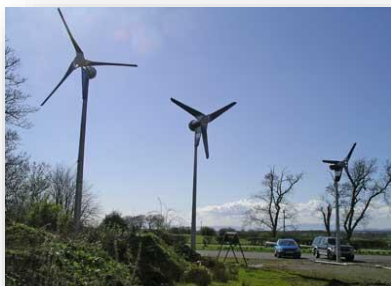
Wind Turbine Installation
