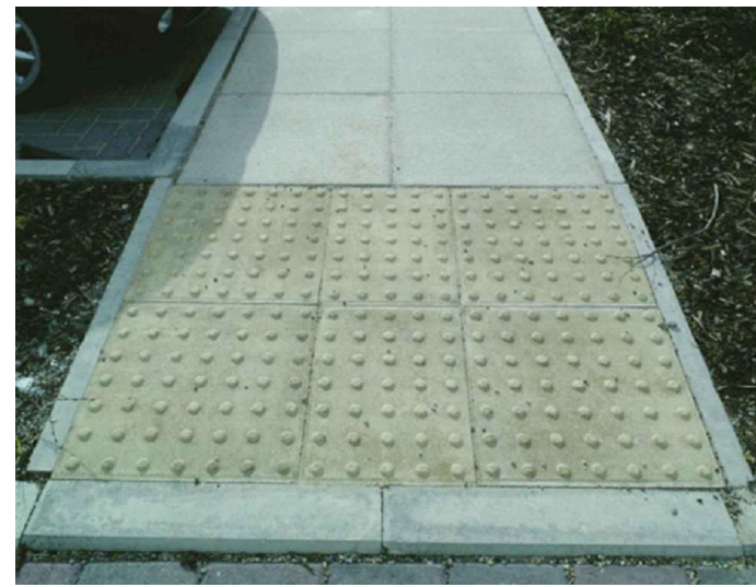
TACTILE PAVING TO CROSSING THRESHOLDS
