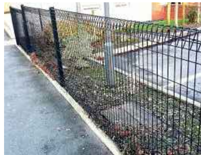
1.2M HEIGHT WELDMESH FENCING
