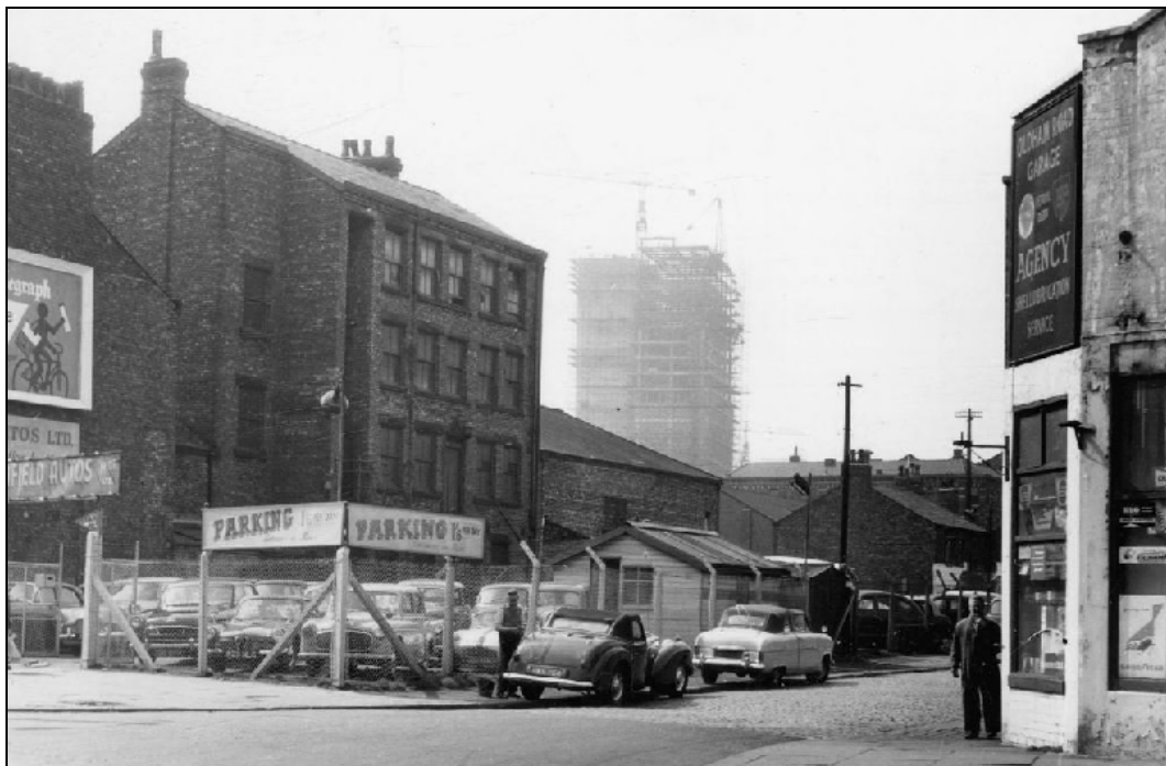
Plate 15: Marshall Street and the Site, in 1961, viewed from Oldham Road. Note the construction of the CIS tower in the background, which was the tallest building in the country upon its completion in 1962
