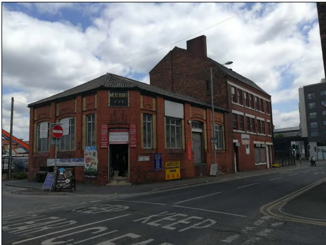
Plate 20: The Site viewed from the corner of Addington Street and Chadderton Street
