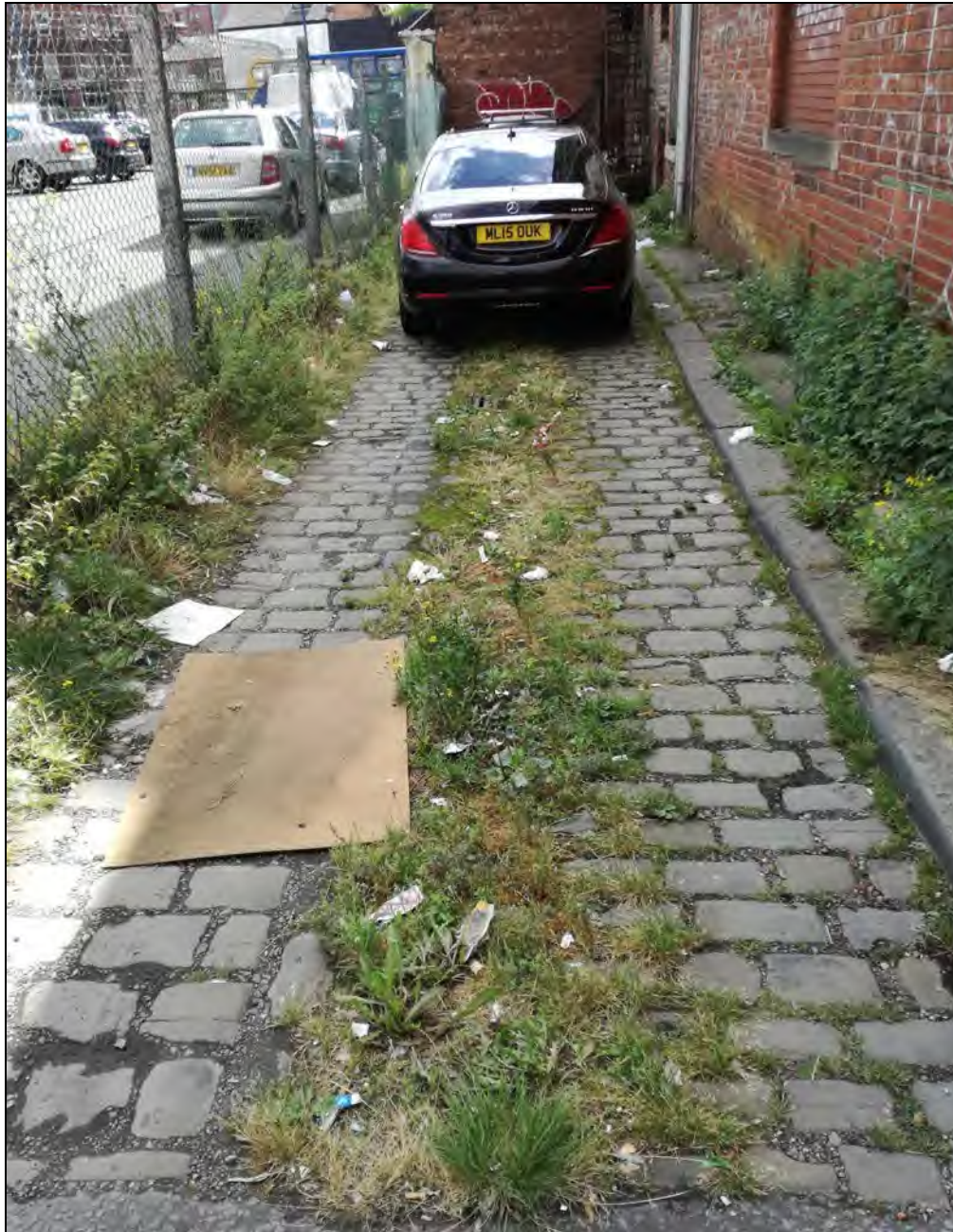
Plate 17: This alleyway of granite setts and large granite kerbs running down the centre of the Site off Chadderton Street was first shown on Swire's map of 1824 and is the only surviving visible evidence of the early 19 th -century occupation of the Site.
