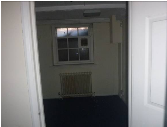
P9 Used section of cellar, no outside bat access
