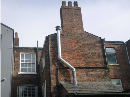
P3 Rear aspect, lit by lights around car park
