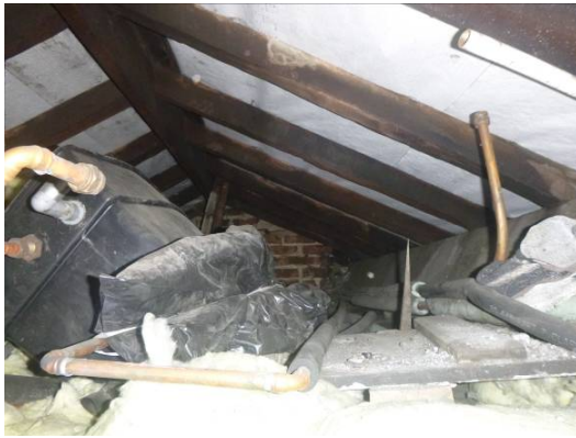
P7 Small roof void
