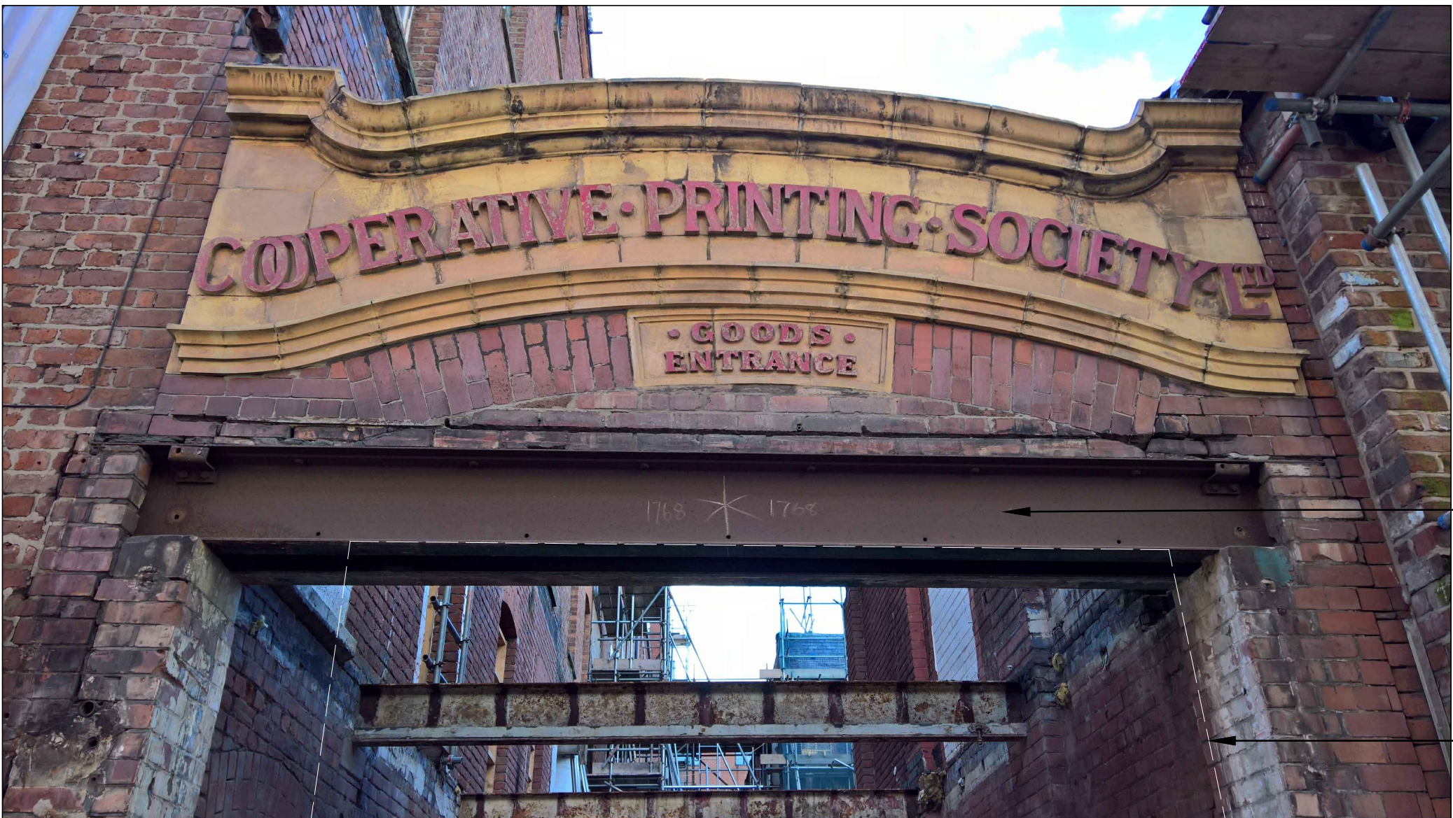
PHOTOGRAPH AFTER REMOVAL OF MODERN BRICKWORK INFILL AND ROLLER SHUTTER
