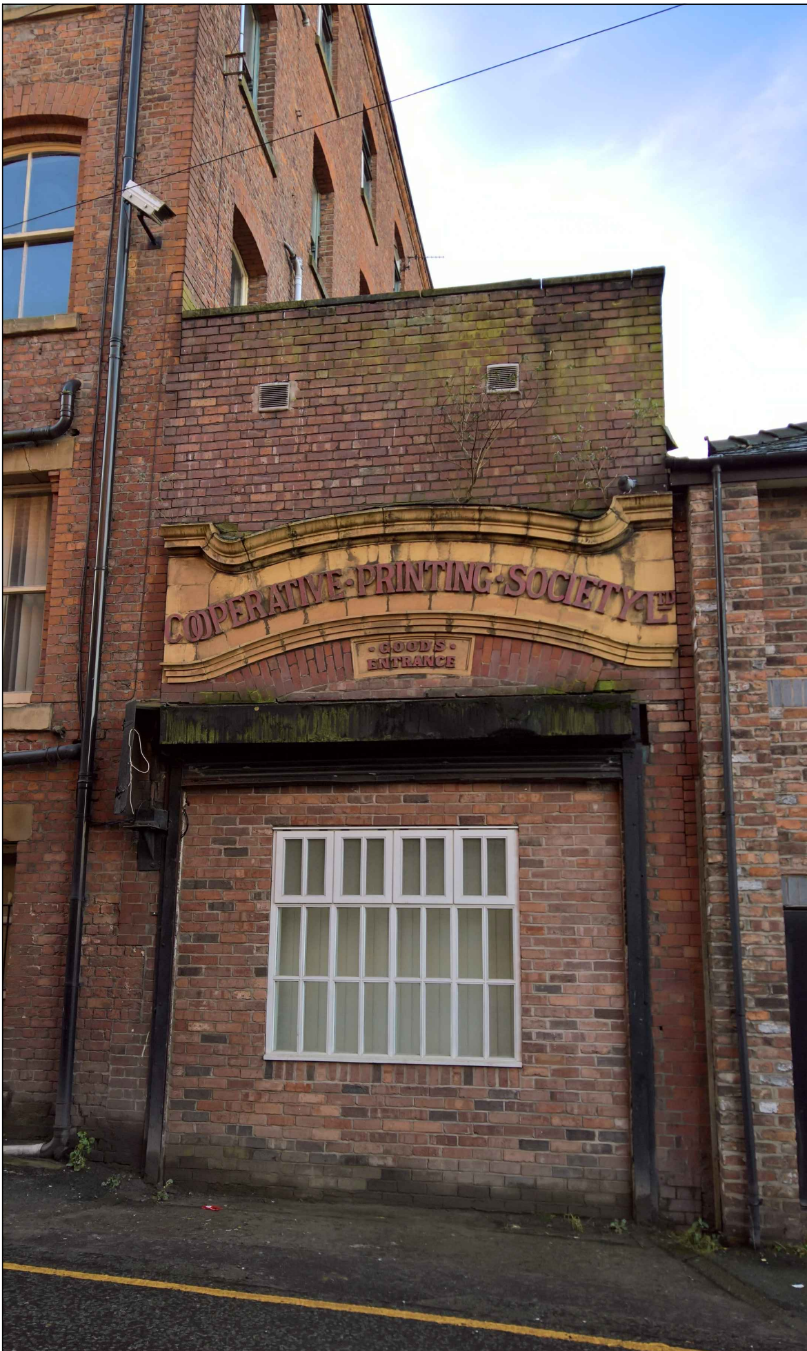
PHOTOGRAPH PRIOR TO REMOVAL OF MODERN BRICKWORK INFILL AND ROLLER SHUTTER
