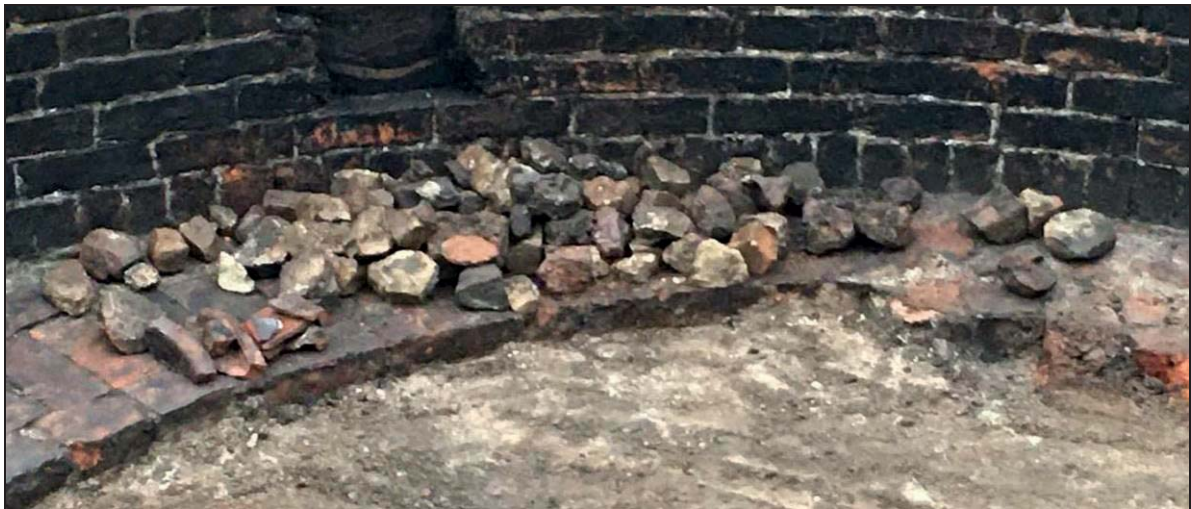
Plate 6: A selection of the material retained from rubble fill (128)
