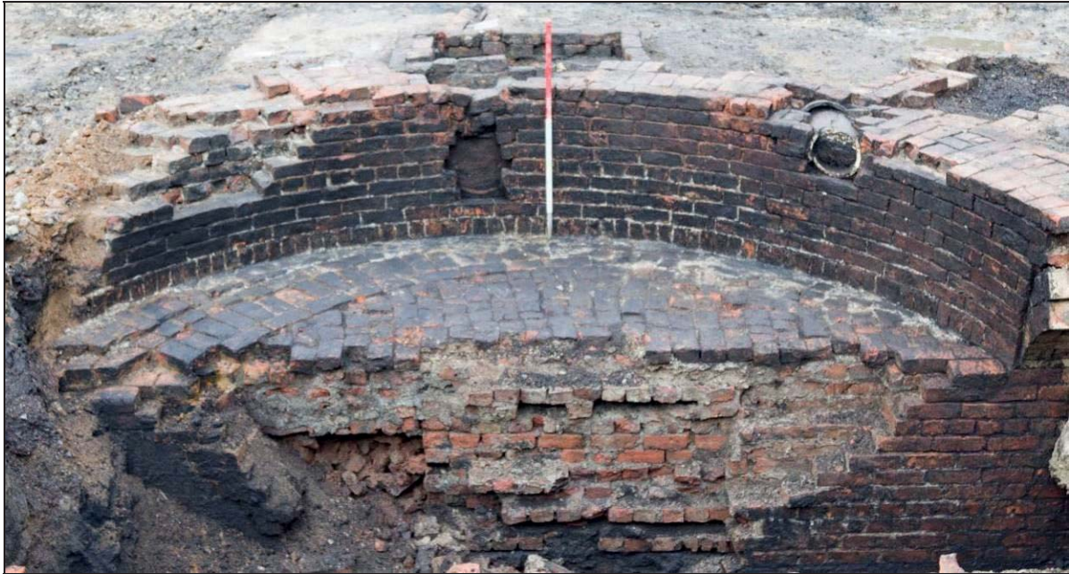
Plate 17: Off-centre circular brick pattern in surface (024) east, and features (138) (right) and (064) (left) built into furnace wall (016), looking north-east. Scale 1m
