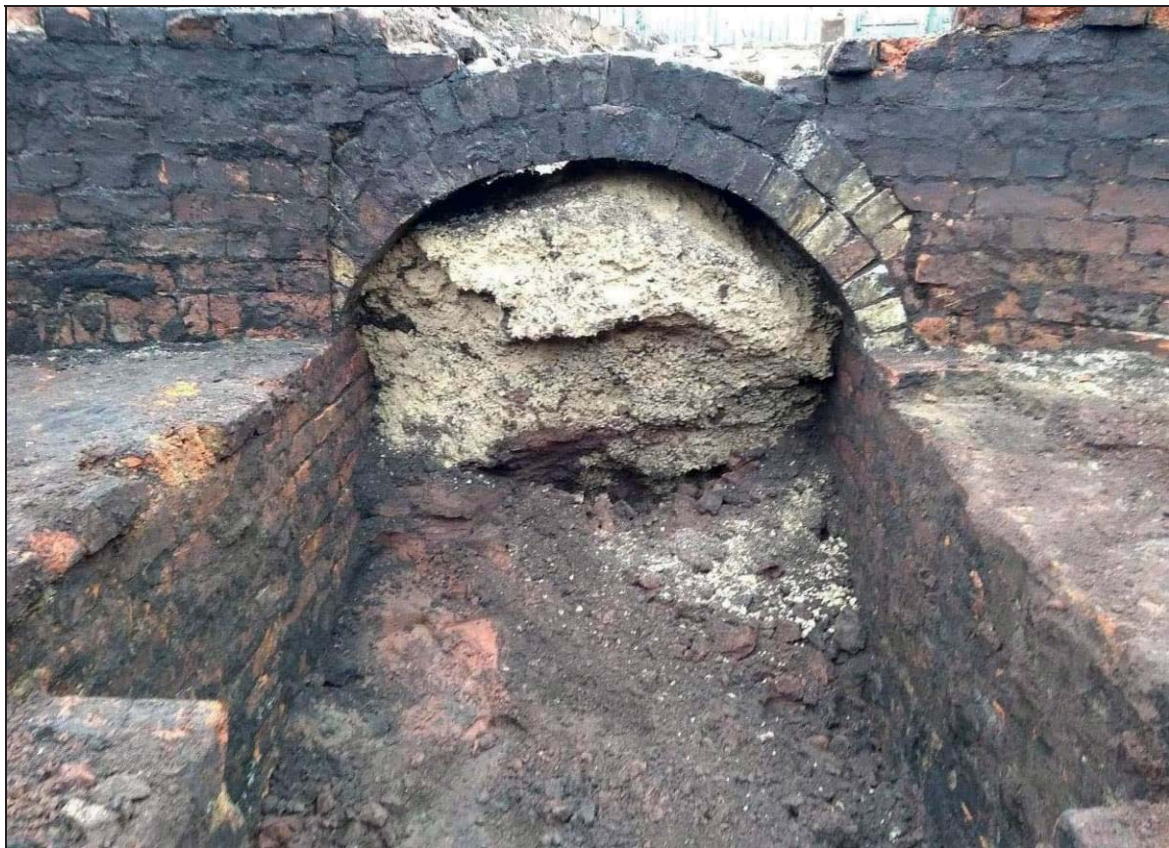
Plate 10: Brick-vaulted arch (026) at the south-east end of the central flue, looking south-east
