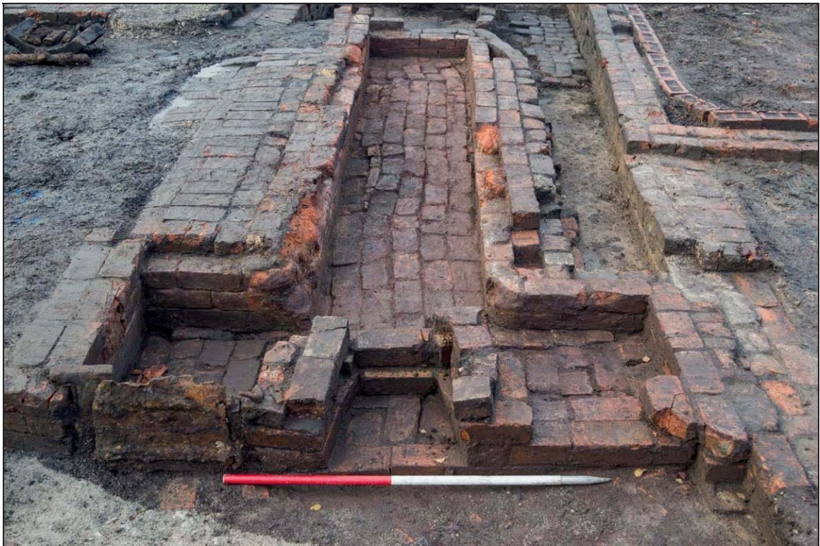
Plate 36: Remains of Cornish boiler bed (118/117/124), looking north. Scale 1m
