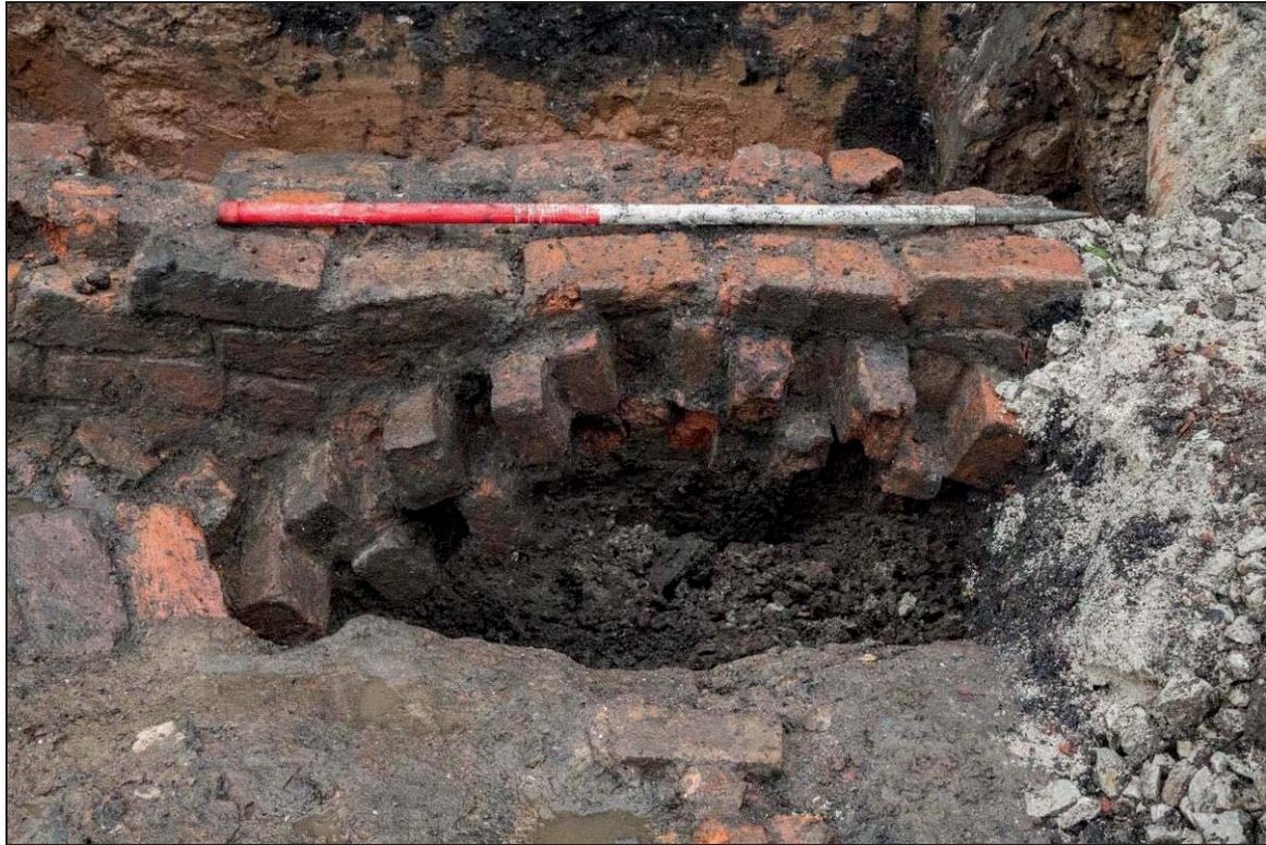
Plate 11: Evidence of the vaulted flue (131) passing through the south-east wall (085) of the workshop, looking south-east. Scale 1m
