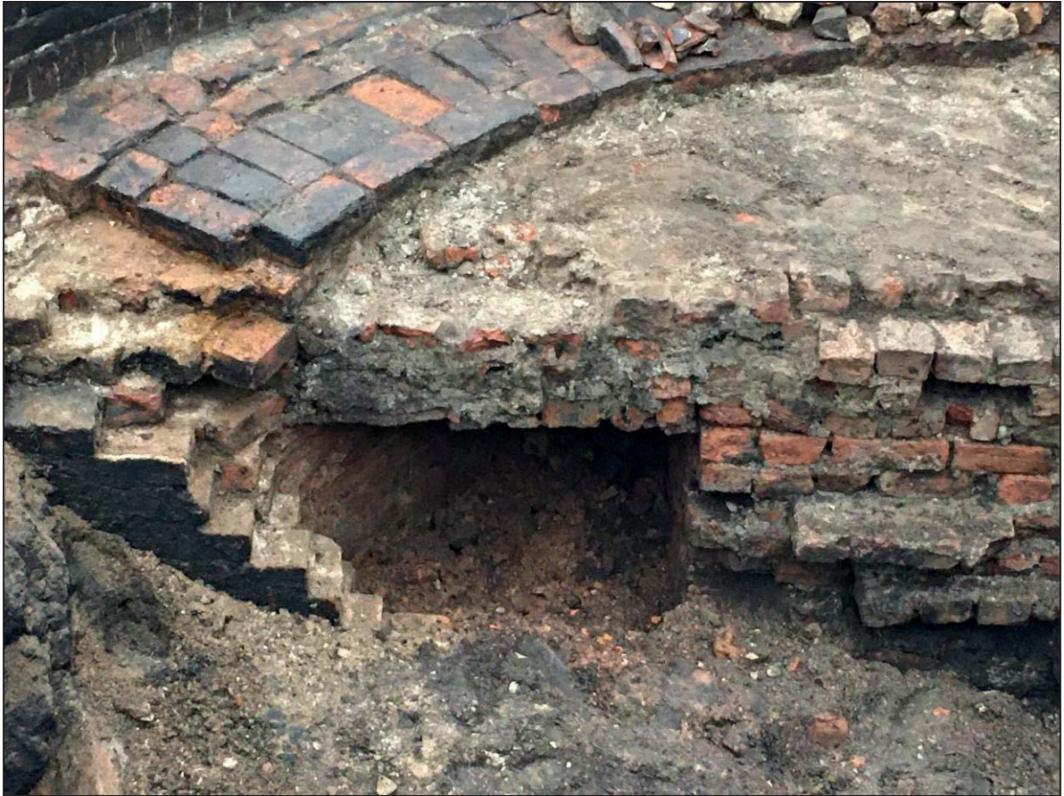
Plate 5: Segment exposed after the collapse of part of wall (153) and the fill (128) partly removed. Brick layer (137) was still in place covering the segment, looking north-east
