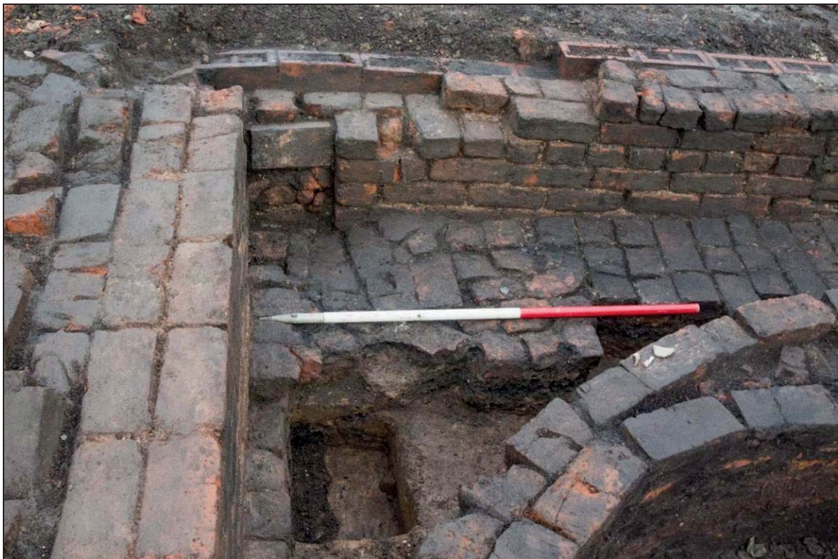
Plate 34: Brick floor (016) inside the northern corner of the workshop, black cinder and waste glass layer (121) lie below, looking north-east. Scale 1m
