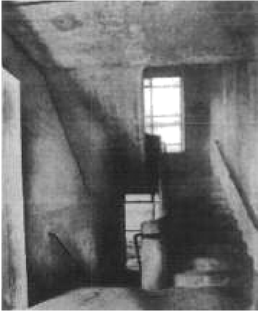
Figure 80 – The main staircase before finishing, as seen in June 1937.
