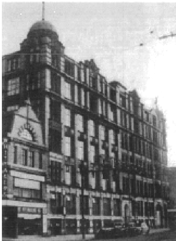
Figure 5 - c1936 – The former corset factory used by the Daily Express from 1927 following the death of James Simpson Blair, seen here shortly before the first phase of demolition in 1936. Whittaker's cabinet makers can be seen at No. 9 Great Ancoats Street to the left of the block.
