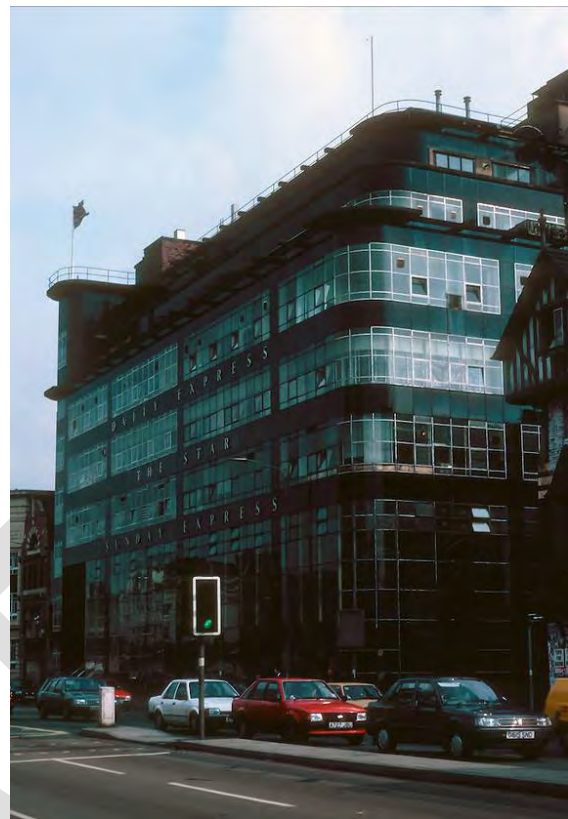
Figure 41 – 1990 – The Great Ancoats Street elevation showing the original 1930s curtain walling.
