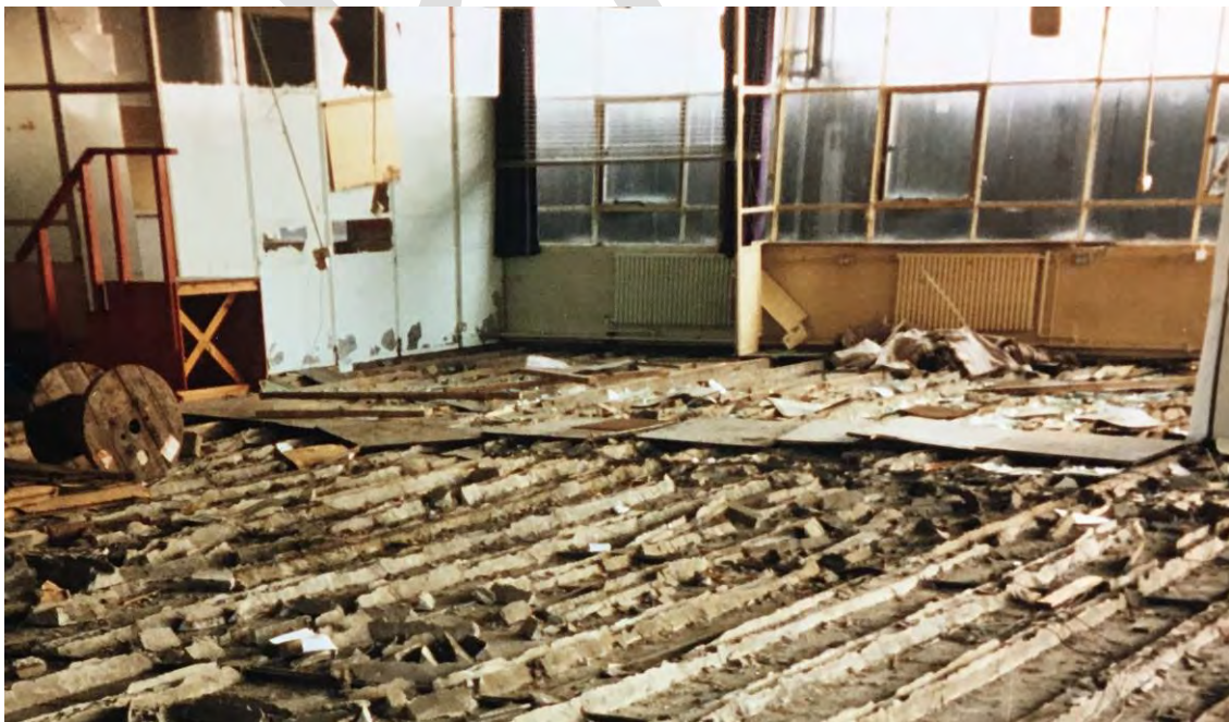
Figure 35 - One of the open-plan floors during demolition works in January 1994 showing the remains of Sir Owen Williams 3ft ply/lino floor tiles and service cavities beneath the flooring.
