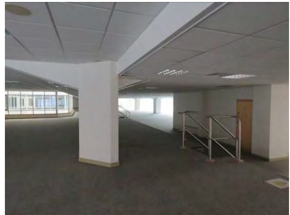
Figure 85 -.Looking across the first floor from the north.
