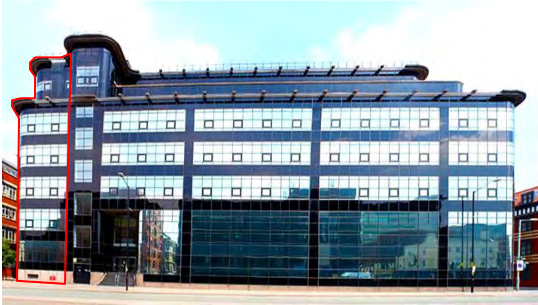
Figure 57 - The same view as seen in 2016, showing the 1992-3 extension to the left (outlined red) and the 1993 replacement glazed curtain walling, and solar film (added in 1998).
