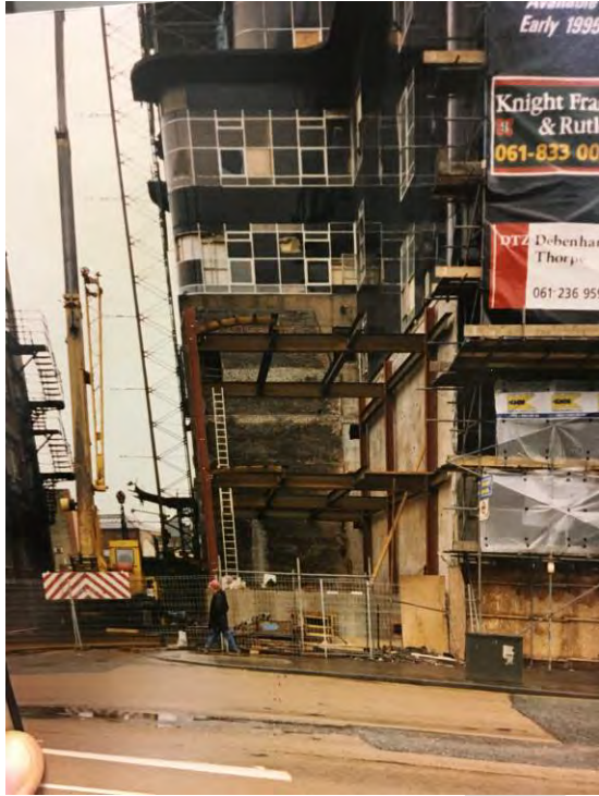
Figure 42 - Erection of ground floor and second floor steelwork, April 1994.
