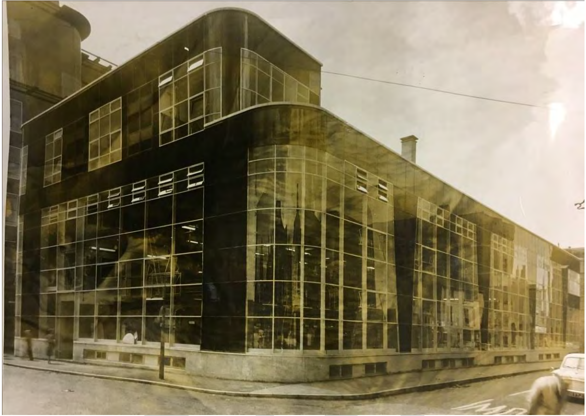
Figure 61 – The newly completed extension as seen in May 1962.
