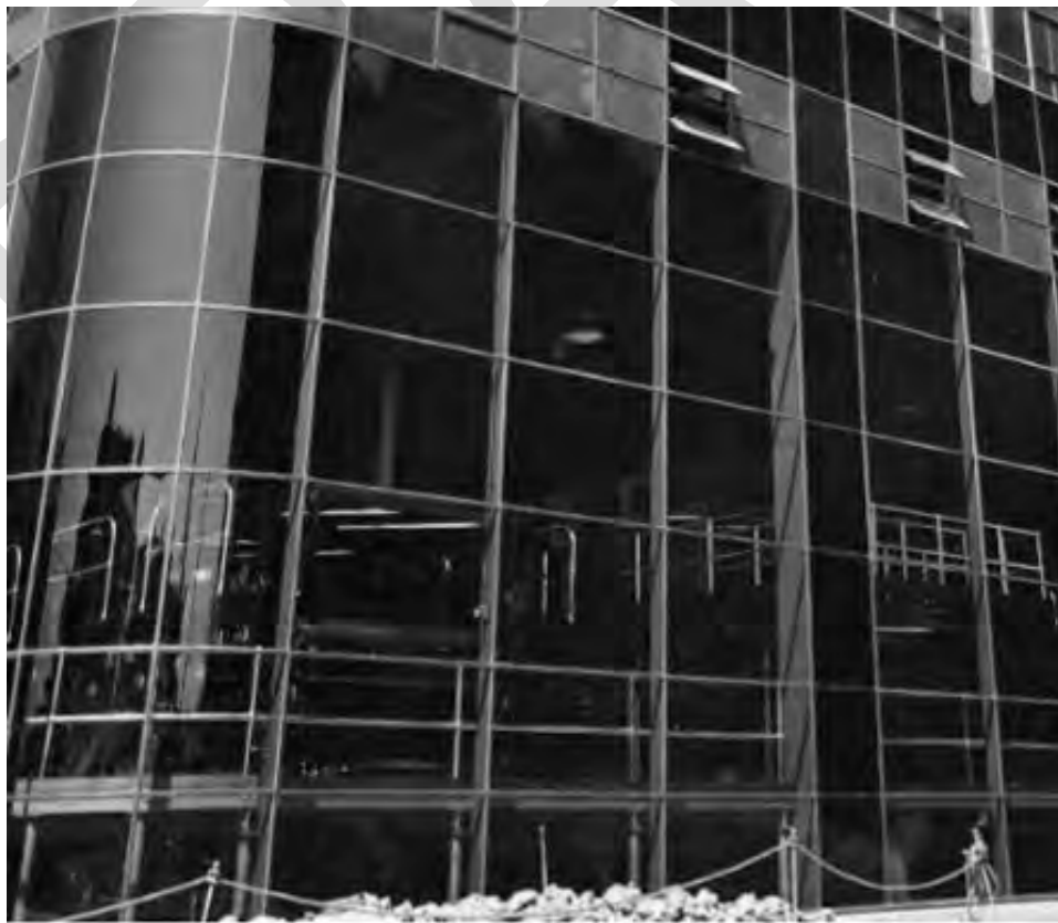
Figure 13- 1939 – A view looking through at the large printing presses and mezzanine floor through the double-height, plain glass elevation on George Leigh Street.
