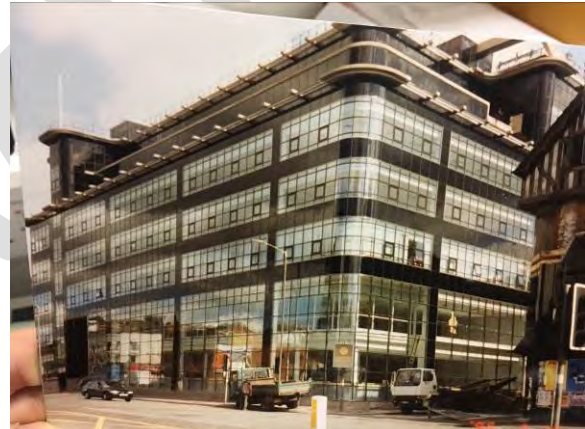
Figure 45 – The newly completed exterior of the building, May 1995.
