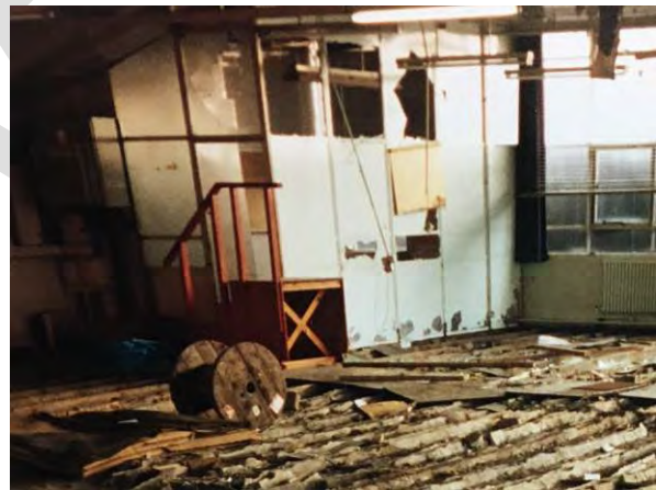
Figure 89 - Removing all internal fixtures/fittings and structures in January 1994, showing one of the original Crittal glazed offices.
