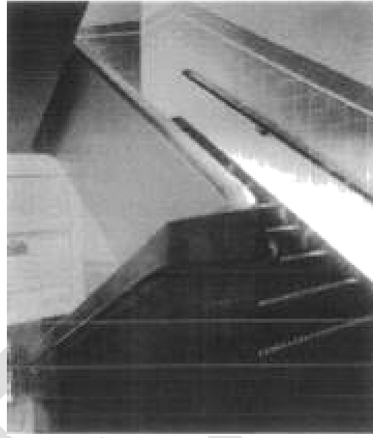
Figure 81 – The main staircase following its completion and finishing 1939.
