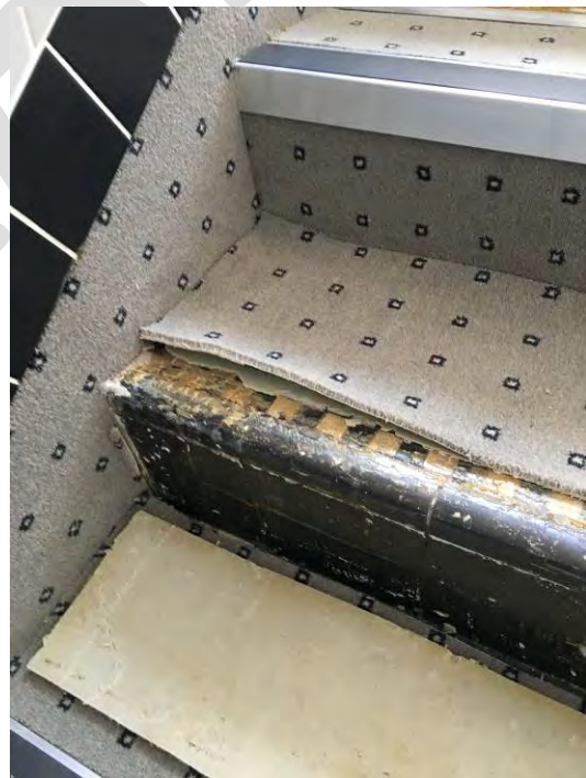
Figure 79 – One of the principal stair treads uncovered to expose the original 1930s black and white tiles (compare with Figure 79).
