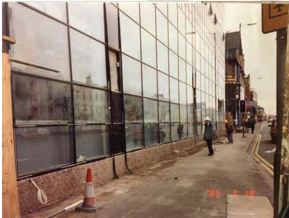
Figure 44 – New curtain walling nearing completion, March 1995.
