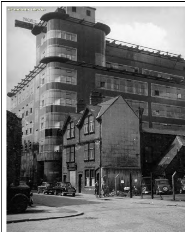
Figure 29 - 1958 – A closer view of the Gun Street elevation, showing the site before the 1960 building was erected.
