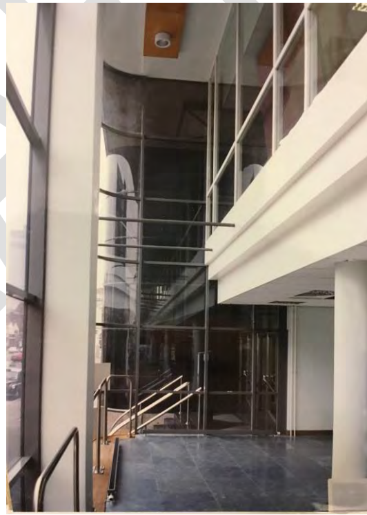
Figure 71 – The same view as seen in 2017, showing the extended 1990s mezzanine floor.
