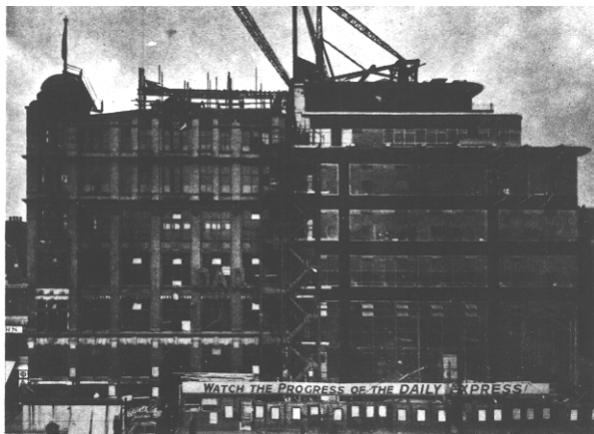
Figure 7 – The Great Ancoats Street elevation showing the point in which the new building (right) is completed, awaiting the existing corset factory (left) to be demolished.
