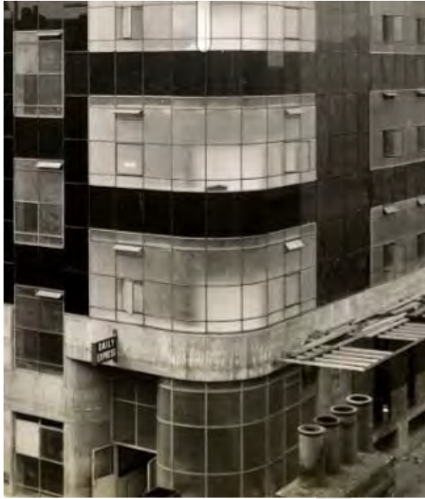
Figure 14 – 1939 – The side entrance on George Leigh Street, showing the original Daily Express sign above the door, and the original configuration of rounded corner Crittall windows to the toilets on each floor. This configuration was shorted in 1993.
