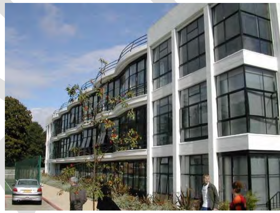
Figure 50 – The Pioneer Health Centre, Peckham, 1934-5. Grade II*.
