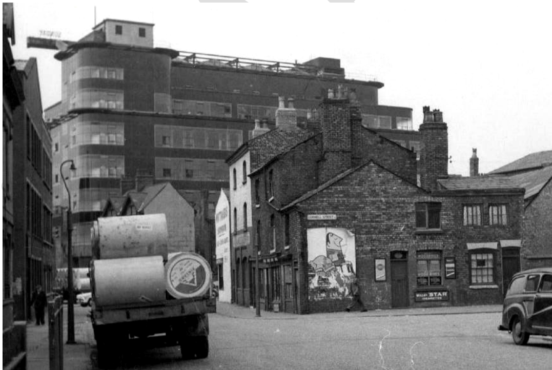
Figure 58 – A view looking south-west along George Leigh Street in 1959, showing the original buildings which were demolished to allow for the construction of the 1960 extension.
