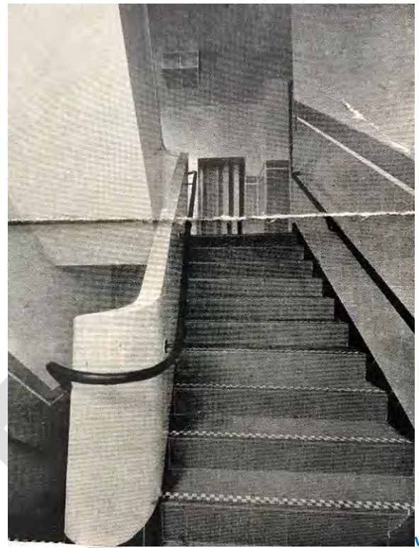
Figure 30 - 1939 – A view of the main staircase on Great Ancoats Street, showing the original black and white glazed tiles to the steps, and tiling to the walls.
