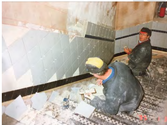
Figure 82 – 5 th to 6 th floor re-tiling of main staircase January 1995.
