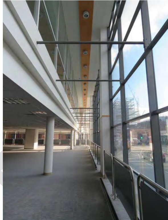
Figure 87 - A view taken from the same position looking along in the opposite (south-easterly) direction, showing the 1992-3 replacement curtain walling and extended mezzanine floor.
