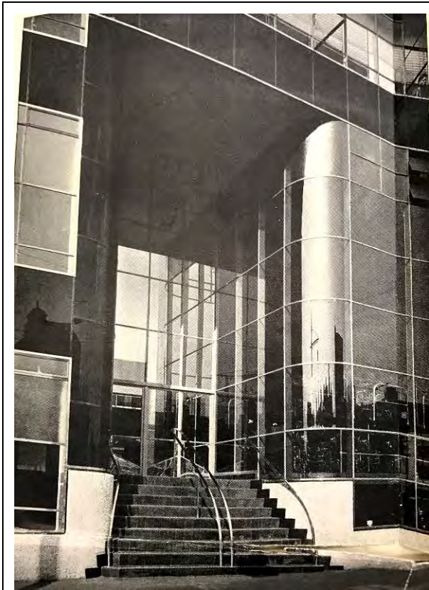
Figure 66 - A view of the original principal entrance into the building in 1939.
