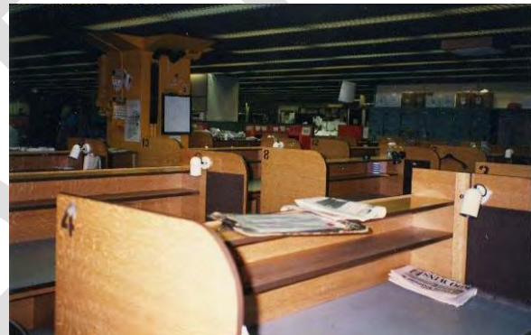
Figure 39 – 1986 – An open-plan office floor showing the subsequent c1970s suspended ceilings.
