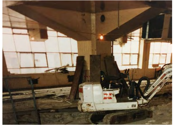
Figure 34 - Demolition works to the internal floors in February 1994, showing the exposed original column.
