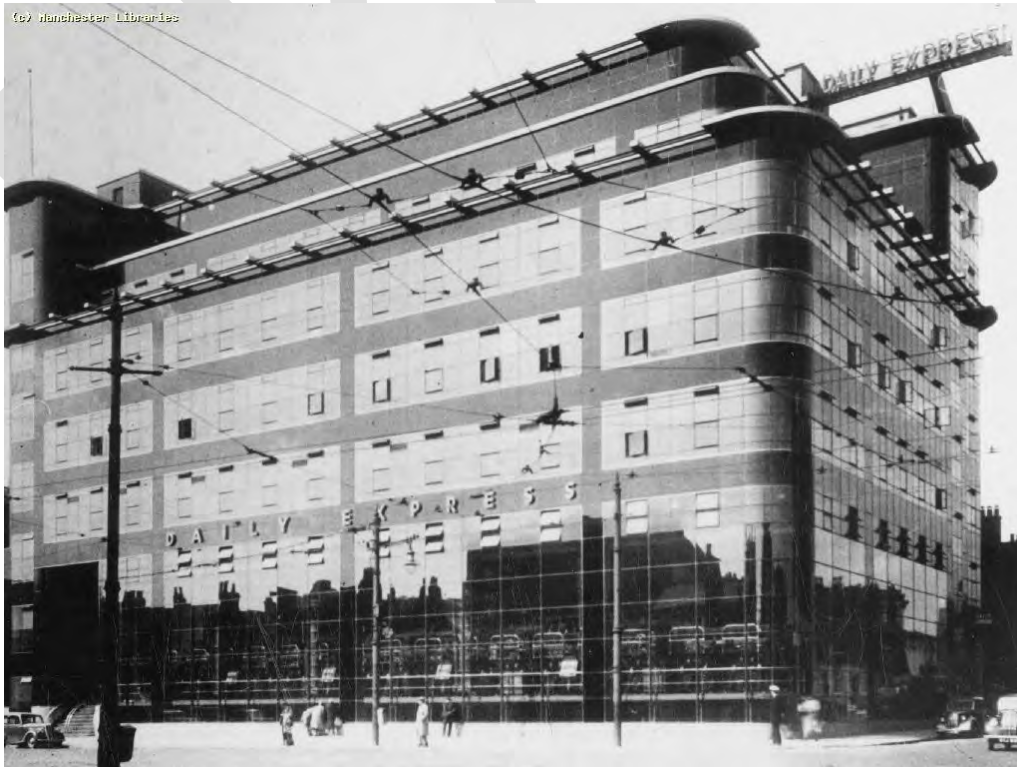
Figure 11: The principal elevation of the new building in 1939, showing the original printing presses clearly visible through the clear glazing of the double-height press hall at street level.
