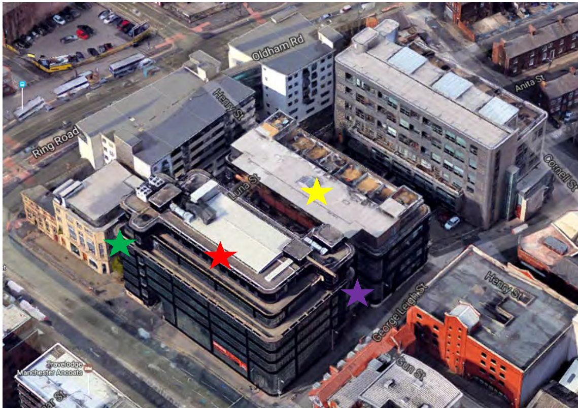
Figure 55 - An aerial view of the site showing the different phases. The red star denotes the original 1936-9 building. The green star denotes the 1992-3 6-storey extension in replacement of No. 9 Great Ancoats Street. The yellow star denotes the 1960 extension with floors added in 1978 and 2001. The purple star denotes the former Gun Street access road, with floors added in 1978.
