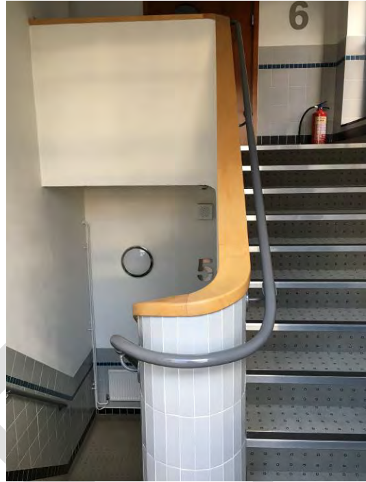
Figure 77 - The same view in 2017, showing the re-tiled walls, new timber banister and carpeted floors. It appears that the metal handrails are the originals.
