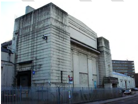
Figure 51 - Palace of Industry building, originally part of the British Empire Exhibition, Wembley, 1924. Unlisted.
