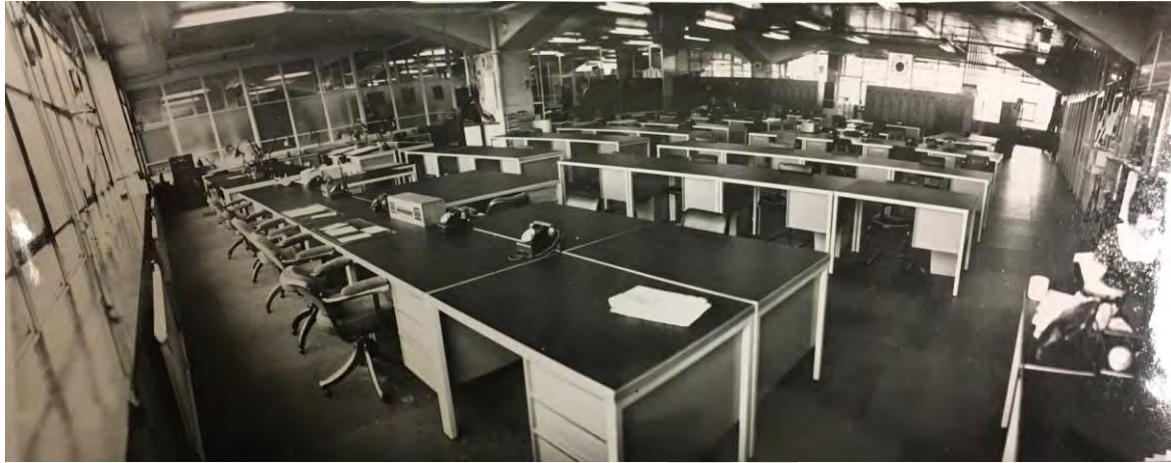
Figure 37 – A general view of an office floor in the early 1960s, showing the concrete cruciform columns and glazed metal-framed internal office partitions.
