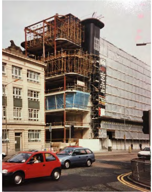
Figure 43 – Erection of new steelwork to fifth and sixth floors of the extension, June 1994.
