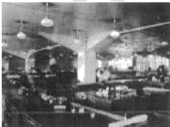
Figure 84 - An office view in 1939. Note the exposed concrete columns and ceiling, with pendant lights.
