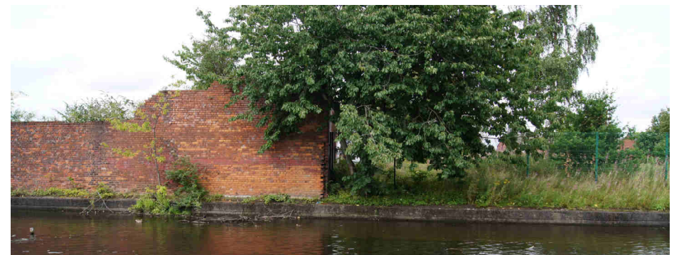
Fig 7. Existing view of wall to western boundary of proposed site.
