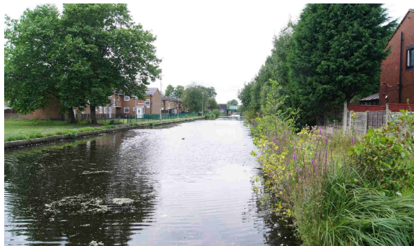
Fig 11. View along Rochdale Canal looking west
