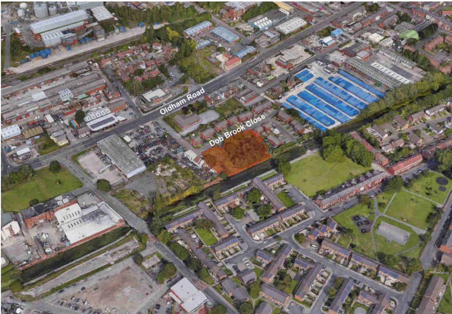
Fig 2. Aerial view of Site
