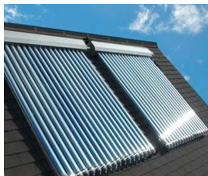
Picture of evacuated solar tube collector
