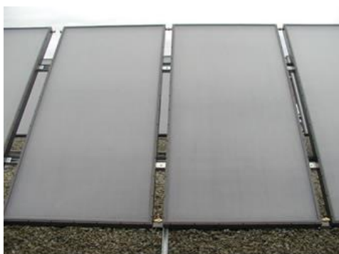
Picture of flat plate solar collector
