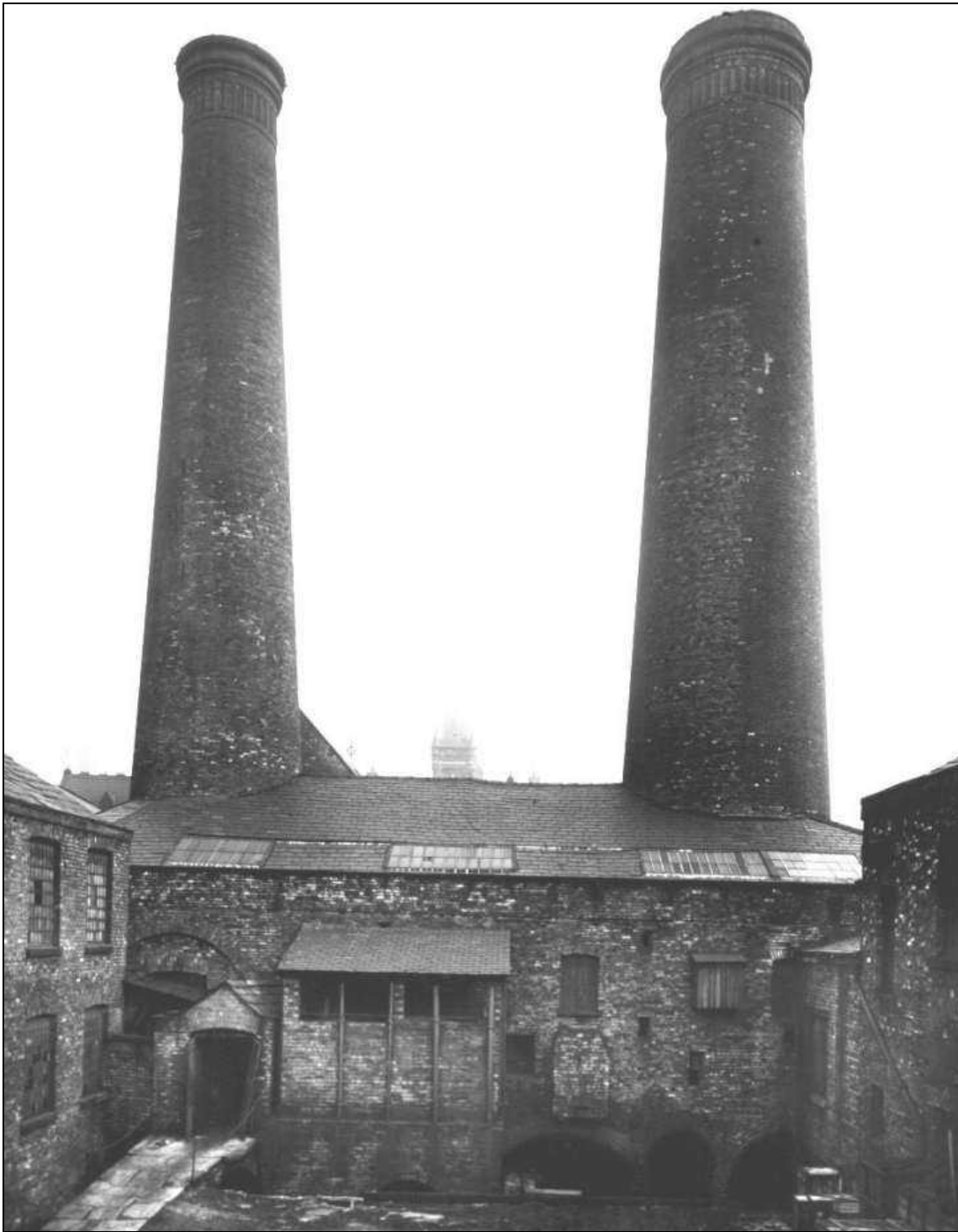
Plate 2: View of two of the glass-melting furnaces at the Molineaux Webb & Co Manchester Flint Glass Works prior to demolition
