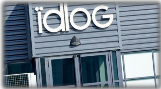
(Thorlux Realta LED as installed)
