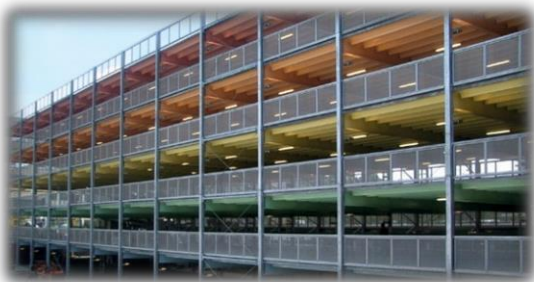
(Thorlux Thoroproof LED as installed)
