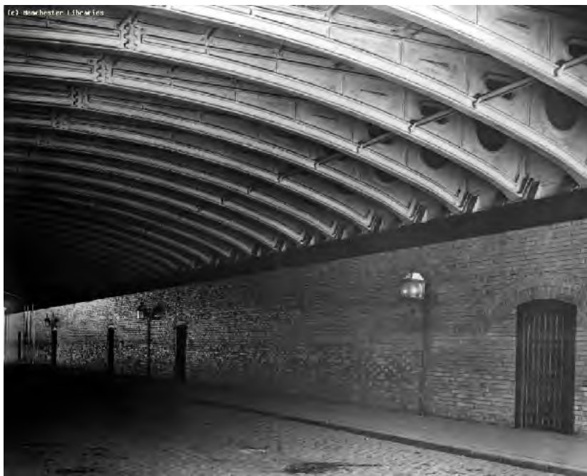
Figure 17: The north side of Great Bridgewater Street, beneath the 1870s viaduct as seen in 1905, showing the original cast-iron roof structure and white glazed brick walls, which remain largely unaltered.
