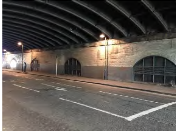
Figure 11: Looking east beneath the viaduct, showing the original glazed brick walls and cast-iron roof structure along the southern side of the street. Note the c1990s arched openings into the former car sales room.
