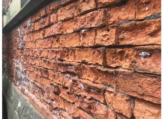
Spalled masonry.
