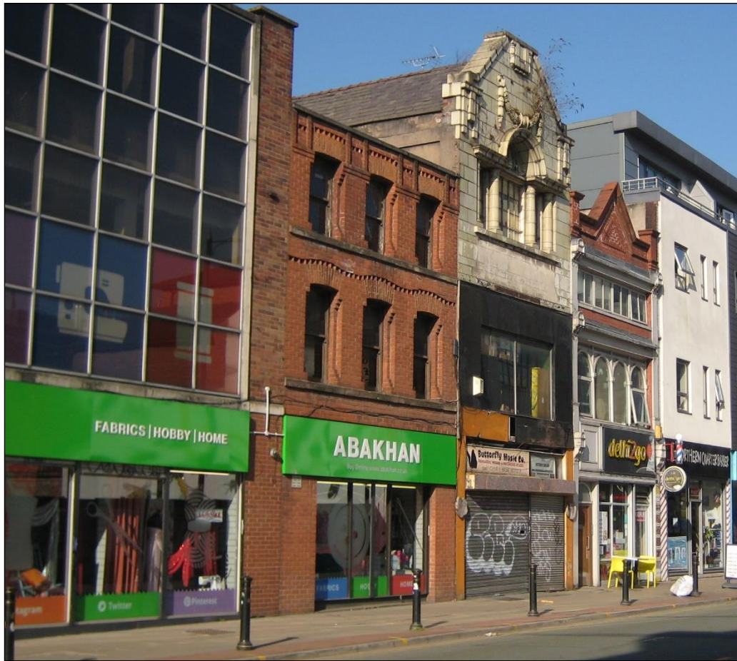
Figure 13: Poor quality signage/shopfronts and condition of buildings.
