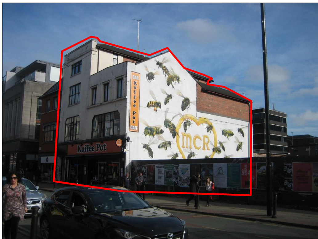
Figure 2: 84-86 Oldham Street – Front and gable of building, looking from Oldham Street.
