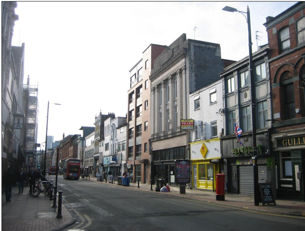
Figure 10: Variable building heights and materials
