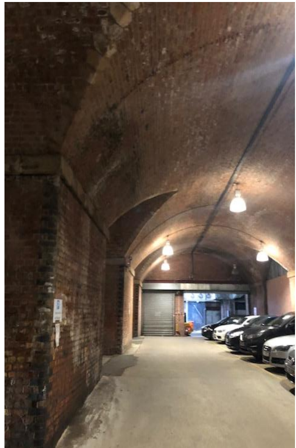
Figure 5: Example of brick undercroft which forms part of the grade-II listed viaduct structure where columns are to be inserted to support the new tower structure above. Whilst the insertion of columns which are to be inserted into the space will result in some adverse visual impact, the revised design will still allow for the architectural character of the undercroft to be understood and appreciated.
