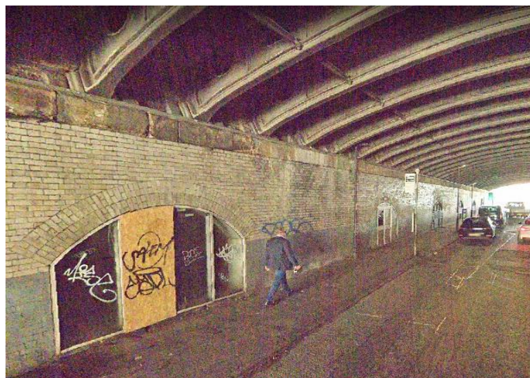
Figure 6: Image taken looking west along Great Bridgewater Street, illustrating the white glazed brick elevation to the listed undercroft featuring arched entrances. The cast iron detailing to the Victorian Bridge is also apparent. Large sections of the bridge are to be removed, allowing for the dark streetscape to be lit by natural light. The brick piers to the arches are to be altered to allow for commercial units.
