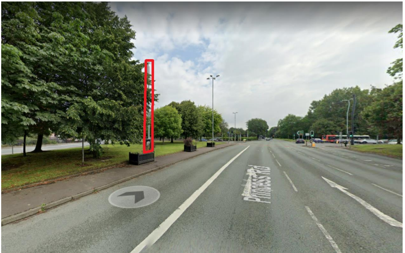
View northwards towards junction with Barlow Moor Road and Princess Road – existing mast highlighted red
