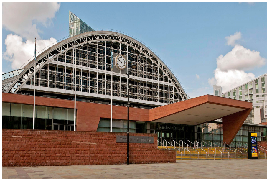
Manchester Central North-East (front) gable view
