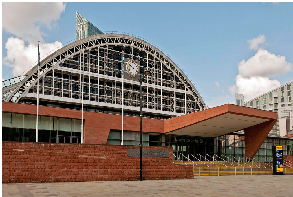
Views of front façade Stephenson Bell extension
