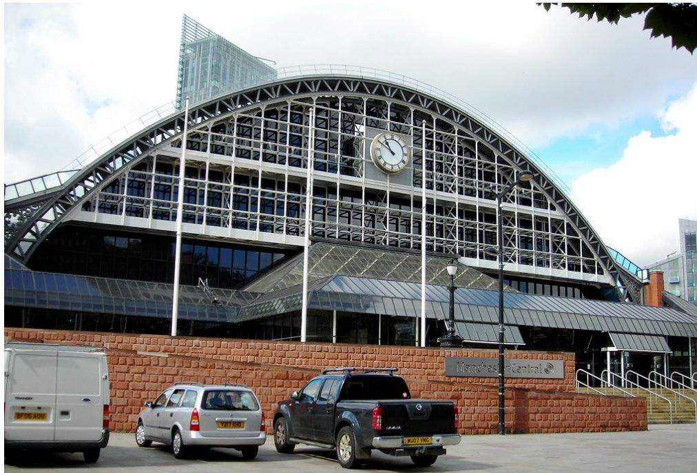
Views of front façade EGS glazed extension
