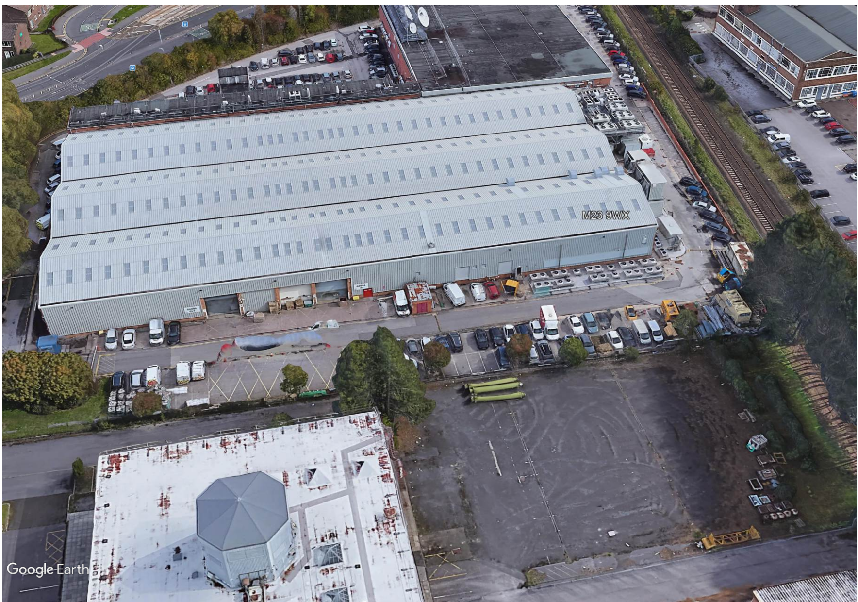
Photo 4: View looking towards the west elevation where the louvre and 12no. condenser units are to be installed.
