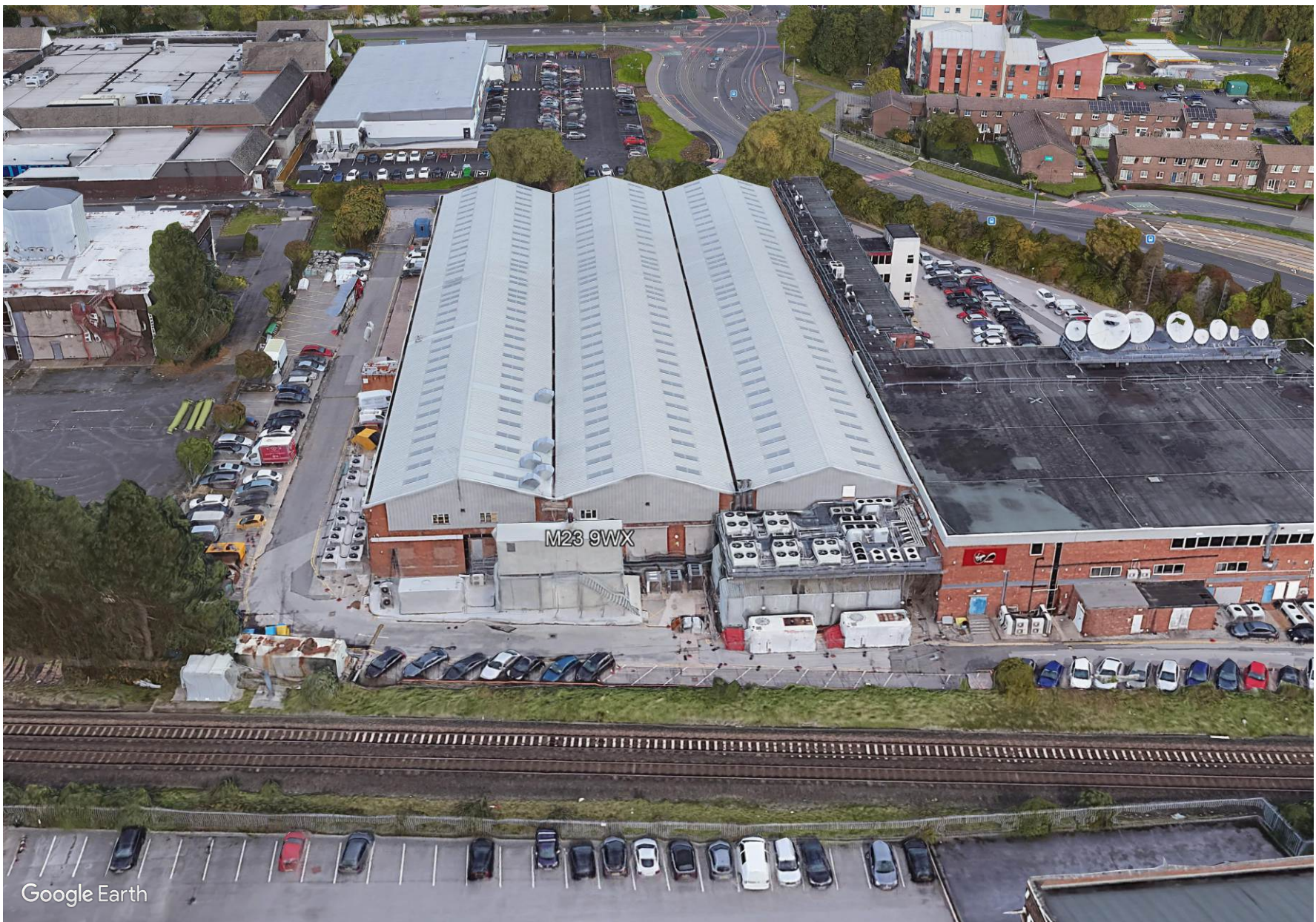
Photo 3: View looking from the south towards where 3no. condenser units are to be installed.
