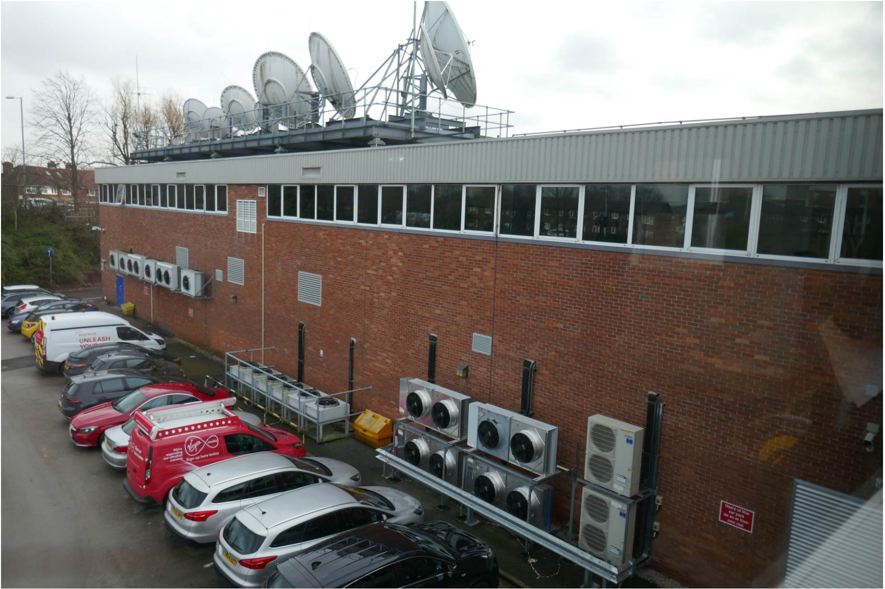
Photo 5: View looking at the north elevation where 2no. condenser units are to be installed.
