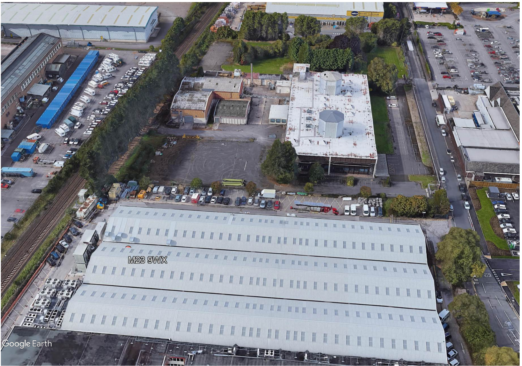
Photo 1: View looking west towards the EDF Energy Building.
