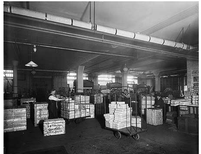
Image 3 showing the basement of Churchgate House, taken in 1900 (Historic England archives). Original form of basement windows is just visible, as are the three presses.
