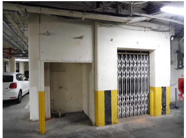
Image 17 showing later-dated lift and hoist openings, towards the front elevation in the basement.
