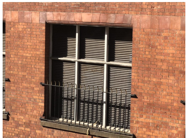
Images 10, 11, 12 showing the canal side elevation with later altered windows and the double timber door.
