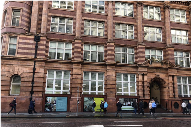
Image 5 showing the front elevation of Churchgate House on Oxford Street. The later altered windows at street level (basement internally) are clearly different when compared to the rest of the building's façade.
