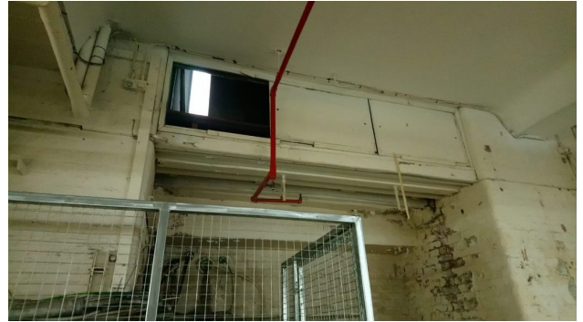
Image 16 showing the underside of the windows to the Oxford Street elevation.
