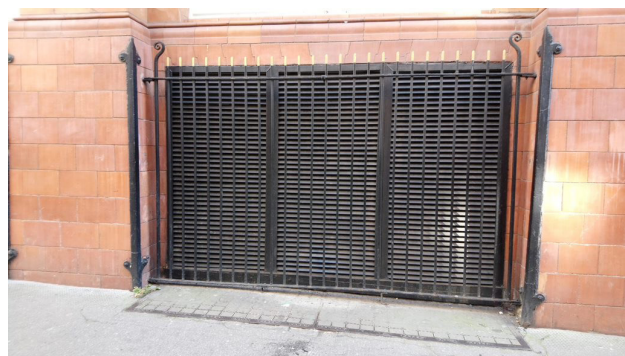
Image 13 showing the louvres added to the Great Bridgewater side elevation.
