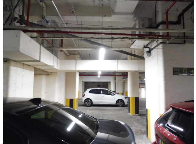
Image 14 showing typical view of the basement area with columns.
