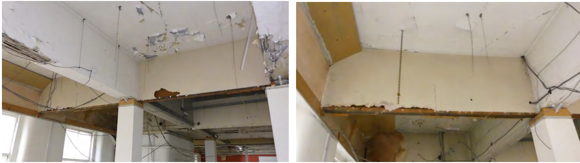
Asbestos insulation board firebreak at high level between the Main Staircase and Back George Street
