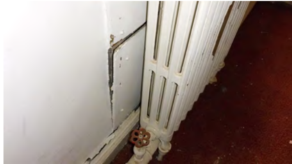
Asbestos cement boarding to the wall behind the radiator
