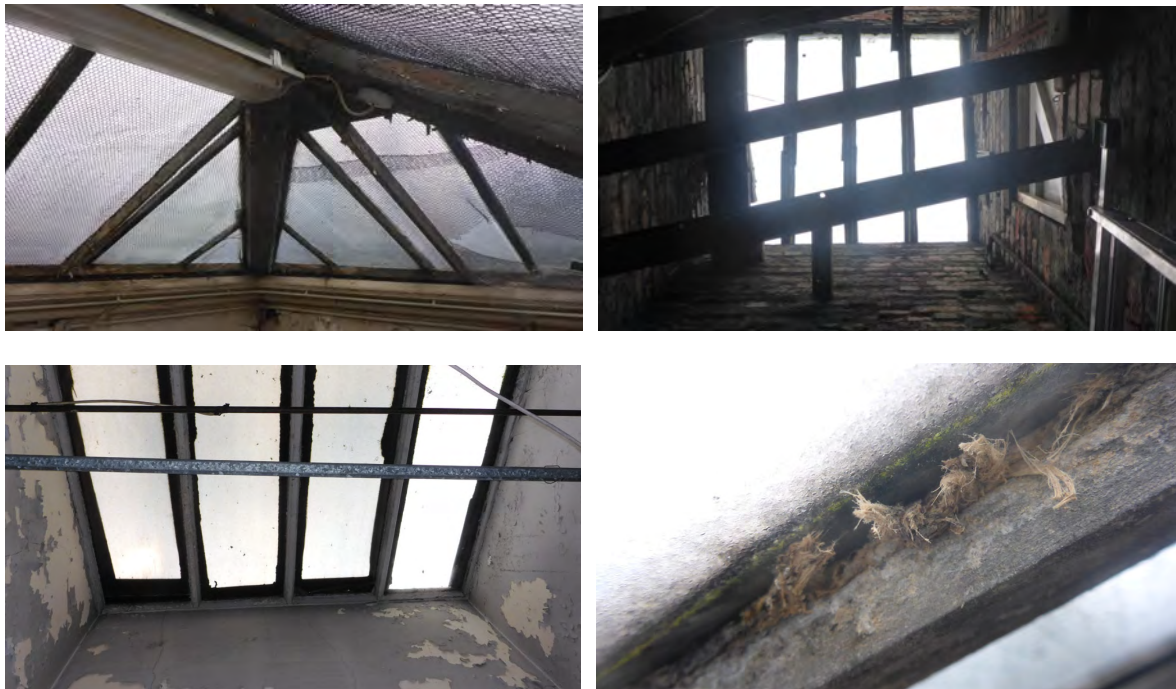
Asbestos rope bedding to the various roof top skylights
