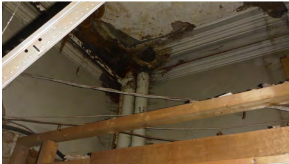
Asbestos thermal insulation to 2 vertical pipes within the box-work and above the Lightwell Lobby Store
