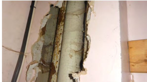
Asbestos thermal insulation to 2 vertical pipes within the box-work and above the Lightwell Lobby Store
