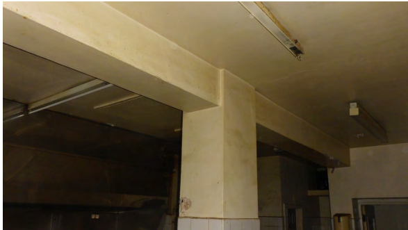
Asbestos insulation board cladding to the structural beams
