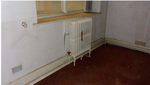
Asbestos cement boarding to the wall behind the radiator
