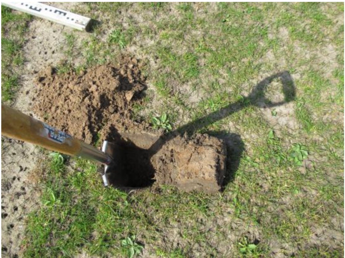
Senior pitch centre-circle trial pit - soil overlying a sand layer. Note the poor grass cover and capped surface soil
