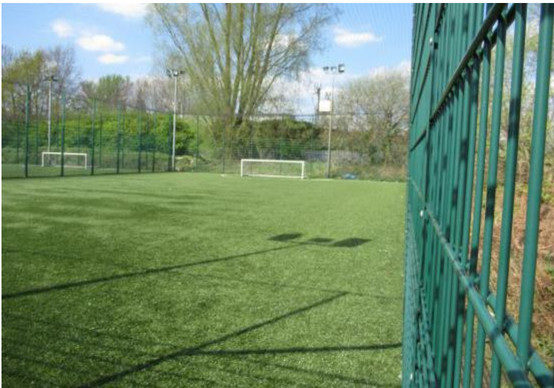
3G court surface and floodlighting in the background. 4m fence and 7metre masts
