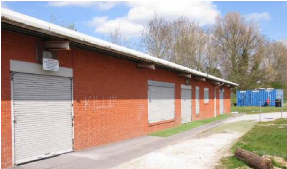
The existing pavilion building
