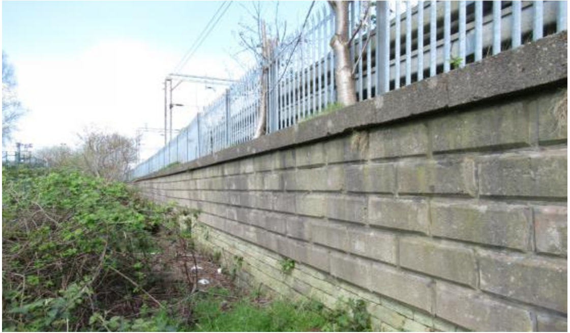
Eastern boundary retaining wall to the Manchester-Crewe railway lines
