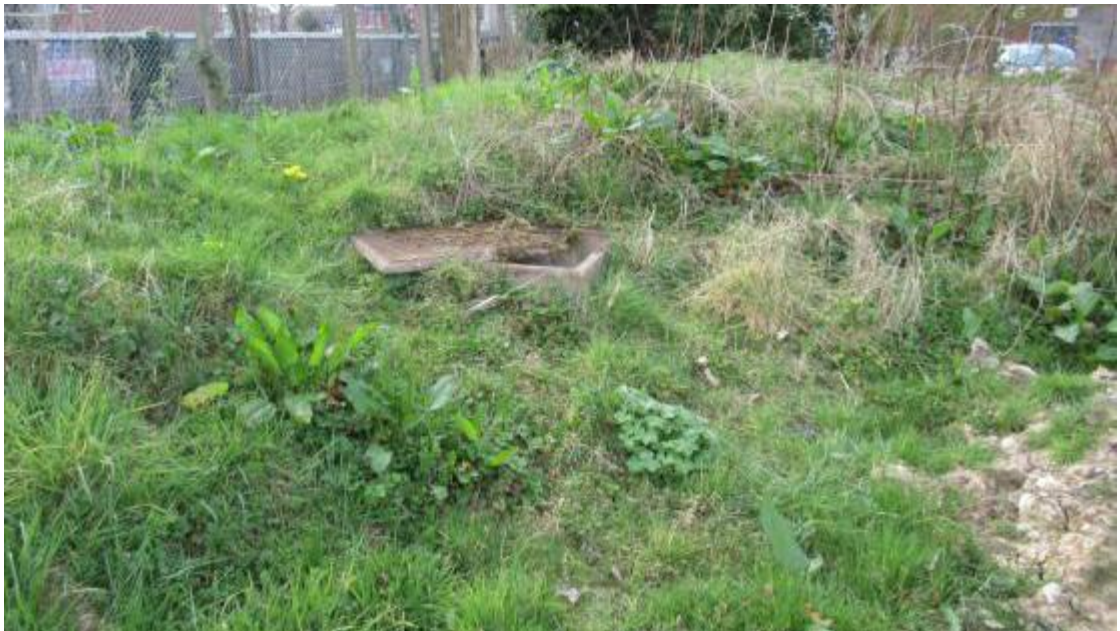
The outfall chamber was installed with the pitch drainage, on the spoil from the drain trenches
