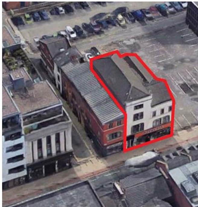
Figure 1 Street view of site
