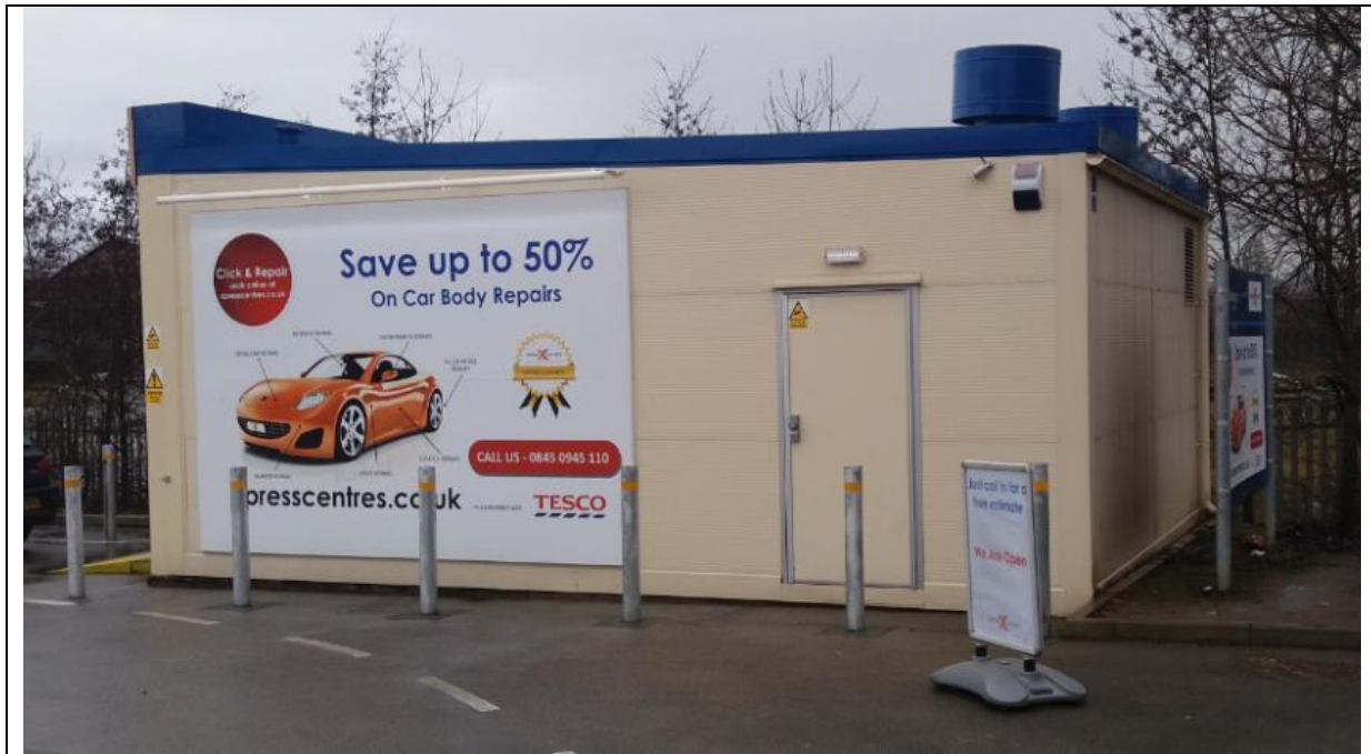
The unit showing the location of the fire door which could be open in summer days.
