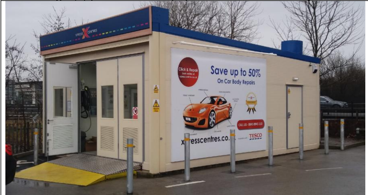
The unit showing front vehicle access and doors closed when vehicle is being worked on. The doors are closed and also vacuum sealed when compressor is on to carry out the processes on the vehicle.
