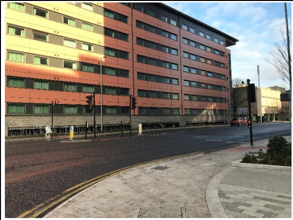
Photograph 4.8 Booth Street West Pedestrian Facilities
