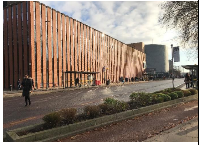
Photograph 4.6 Oxford Road (northbound) Bus Stop, north of junction with Booth Street West
