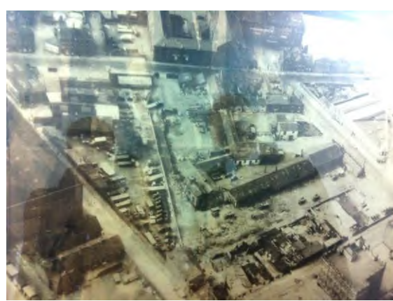
Figure 4: A view looking in a westerly direction over the wider site in the 1930's, showing the Bonded Warehouse and stables on Grape Street to the bottom left corner and the filled in Junction Canal network to the centre of the view. The Victoria and Albert Warehouses can be seen to the top right corner and the remaining townhouses forming Lower Irwell Street to its left.
