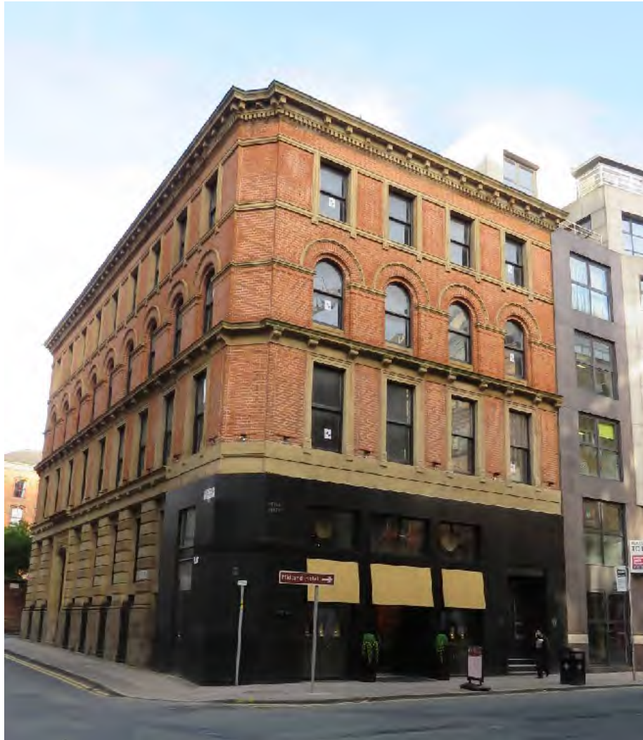
Figure 1: A view of 47 Peter Street looking north-east
