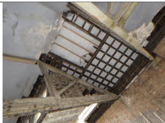
Figure 32: internal view of the roof structure and covering; note former opening has been covered.
