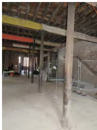
Figure 18: view of the first floor looking north. The area where the principal staircase for the building was once located can be seen to the right.
