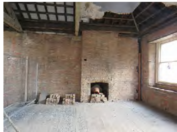
Figure 28: south-east corner of the third floor, illustrating former fireplace and chimney flue. Note various coverings to the roof.
