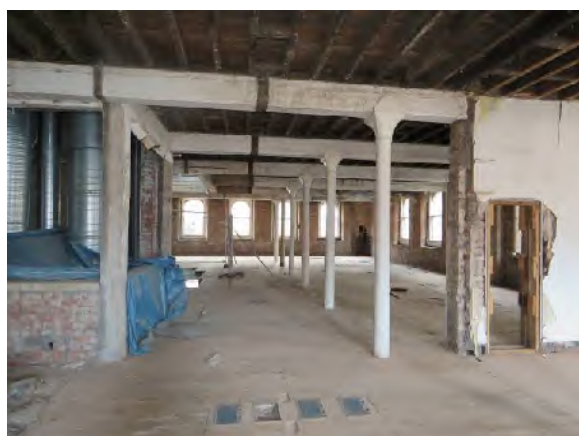
Figure 19: View of the second floor looking south, as per Figure 17.
