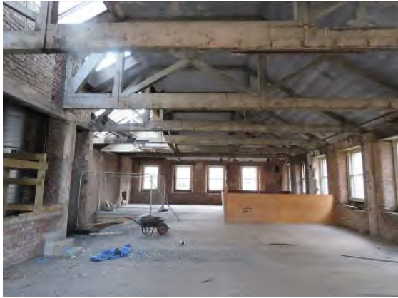
Figure 25: view of the third floor looking south illustrating the timber roof structure.
