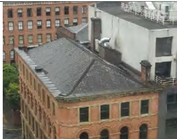
Figure 29: External view of the roof looking north illustrating the pitched form of the roof, the remains of 3 chimney stacks to the left (west) side, and the remaining chimney stacks and flues to the right (east).
