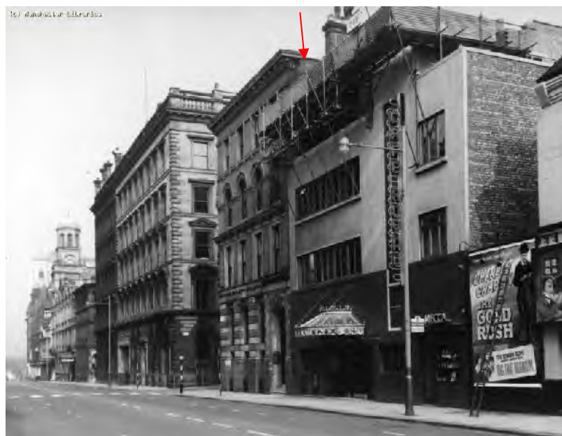
Figure 7 – c.1955 photo of Peter Street – note original ground floor elevation of No.47 and what appears to be new brickwork to the parapet (denoted by red arrow). The building next door to No.47, the Café Royal, still has scaffolding to its upper levels, presumably in light of bomb damage the building suffered.
