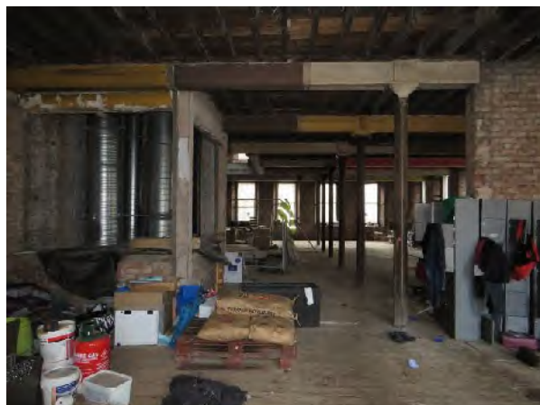
Figure 17: view of the first floor looking south. Later lightwell structure (now used as a riser) seen to the left. A row of columns to the centre of the open-plan floor plate is the only notable original feature left internally. Remains of an altered brick wall, possibly marking the former location of the 1896 inserted staircase is seen to the right.
