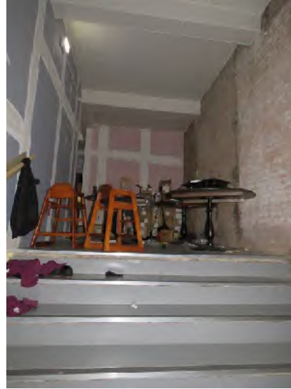
Figure 11: view from the side entrance off Peter Street looking up the internal entrance stairs to the raised ground floor. Modern plasterboard partitions were inserted as part of the refurbishment works for the restaurant. The pink plasterboard marks the location of a lift core. There are not historic fixtures or fittings of note in this space.
