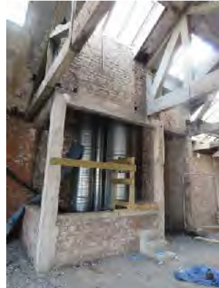
Figure 26: view of the former lightwell structure (later addition, possibly post-bomb damage), now used as a dry riser. This photo also illustrates the various rooflights to this side (east) of the roof.
