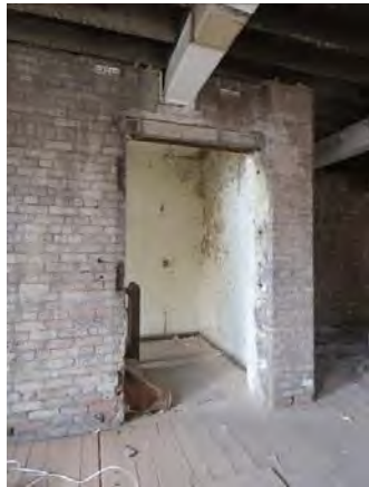
Figure 21: View back towards the rear/ service staircase – note alterations to the opening
