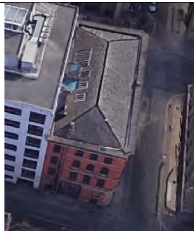
Figure 30: External view of the roof looking south which provides a clearer view of the west side of the roof with its existing roof lights and flues.
