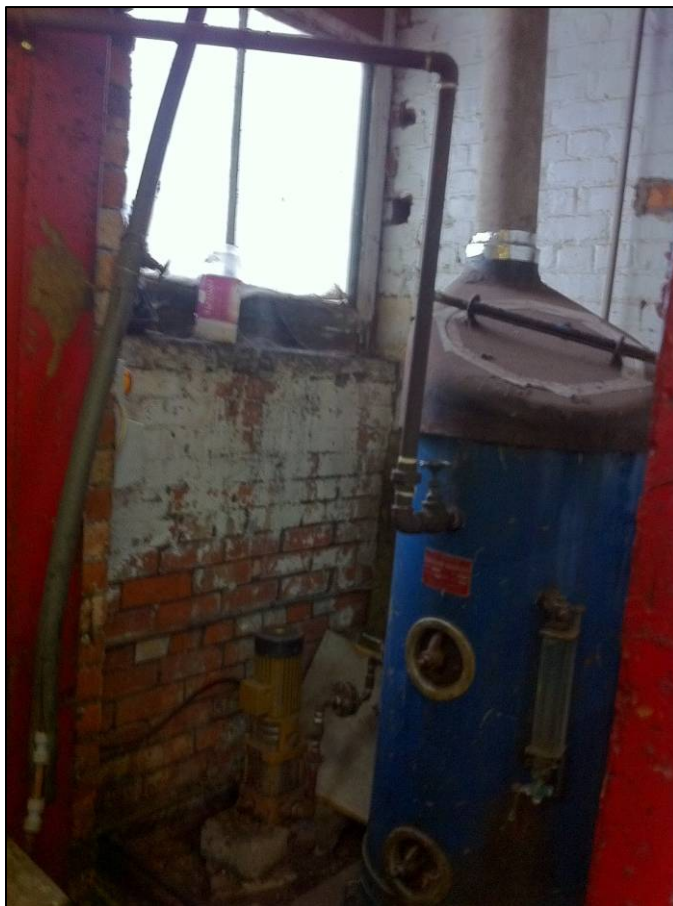
Plate 12 Interior of Section C of the building
