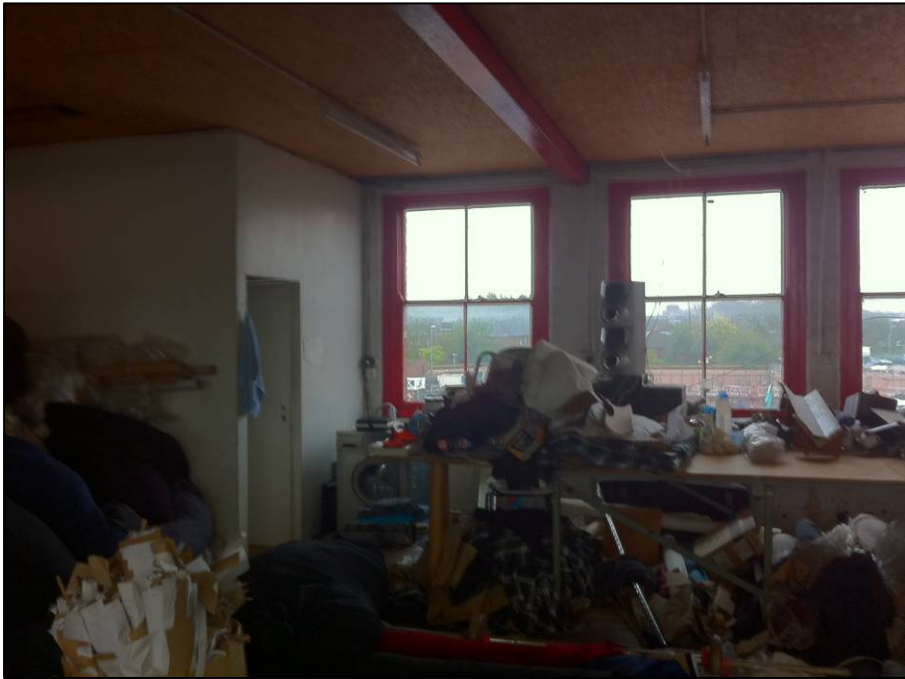
Plate 9 Interior of Section B of building - the 2 nd Floor
