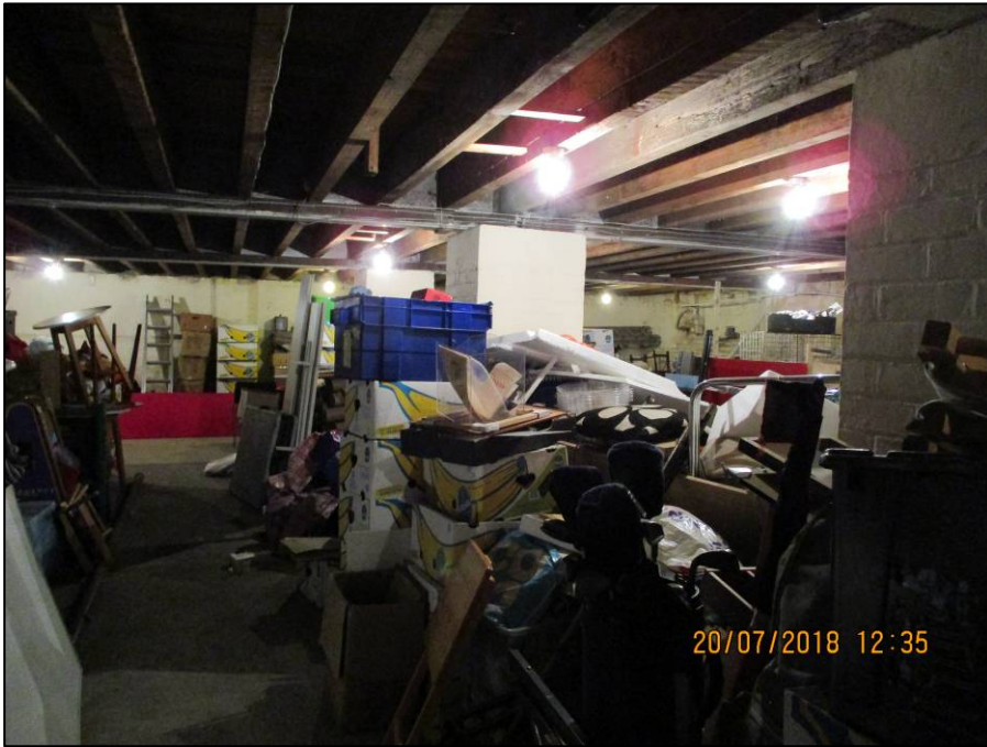
Plate 7 Interior of Section A of building showing enclosed cluttered space
