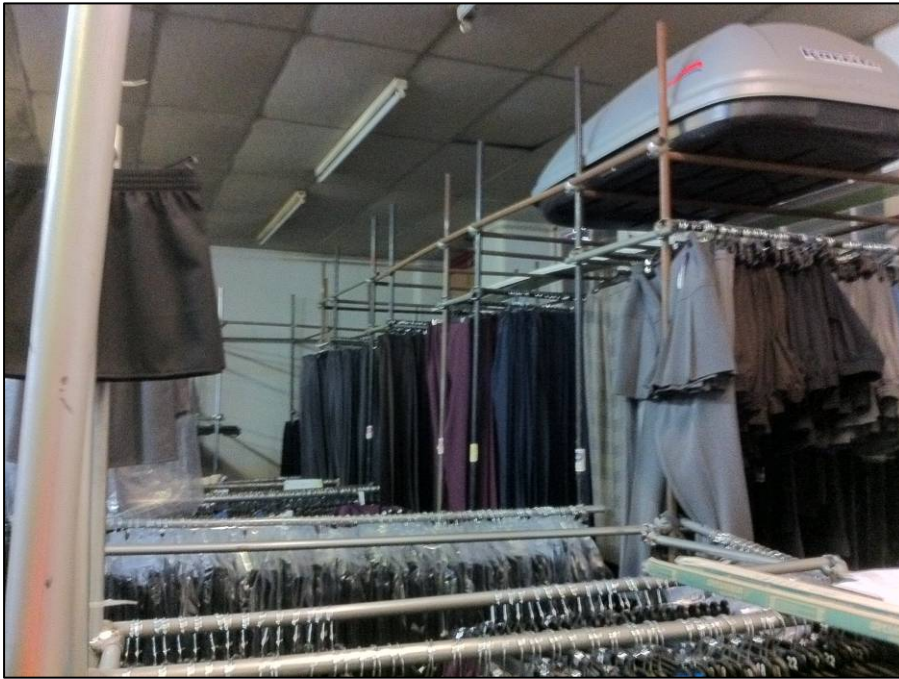
Plate 11 Interior of Section B of building - Ground Floor
