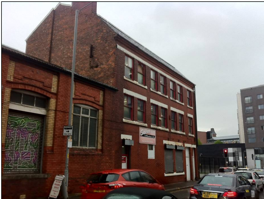
Plate 1 The exterior of the building facing onto Addington Street, showing slate mansard roof
