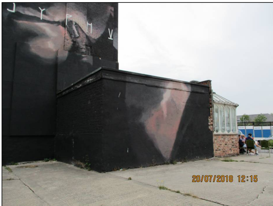
Plate 4 Exterior of small building with flat roof
