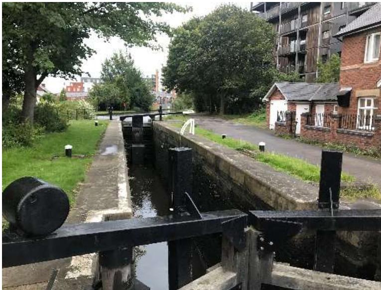
Figure 3.4 Lighting bollards east of Allan Turing Way
