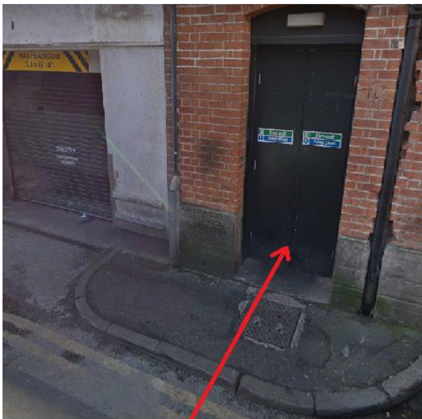
All servicing through the rear doors on Bootle Street
