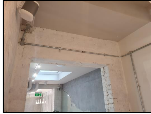
Fig 2 & 3 – Photos of the structural beam restricting internal route of extract.
