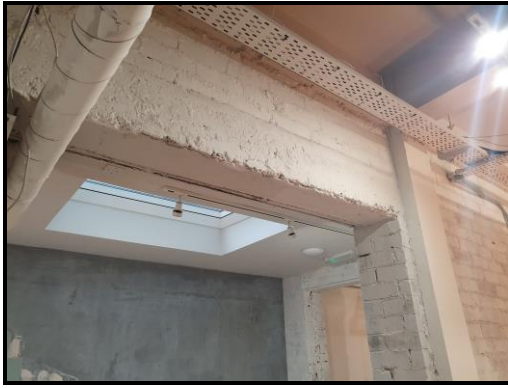
Fig 2 & 3 – Photos of the structural beam restricting internal route of extract.
