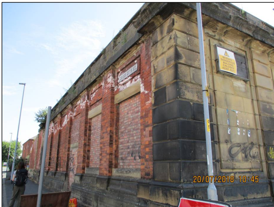
Plate 2 Exterior elevation, facing onto Cross Keys Street, showing exterior wall construction
