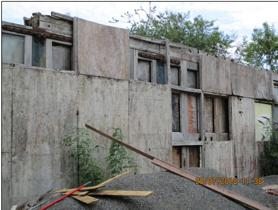
Plate 9 Wooden hoarding / doors with metal pillars
