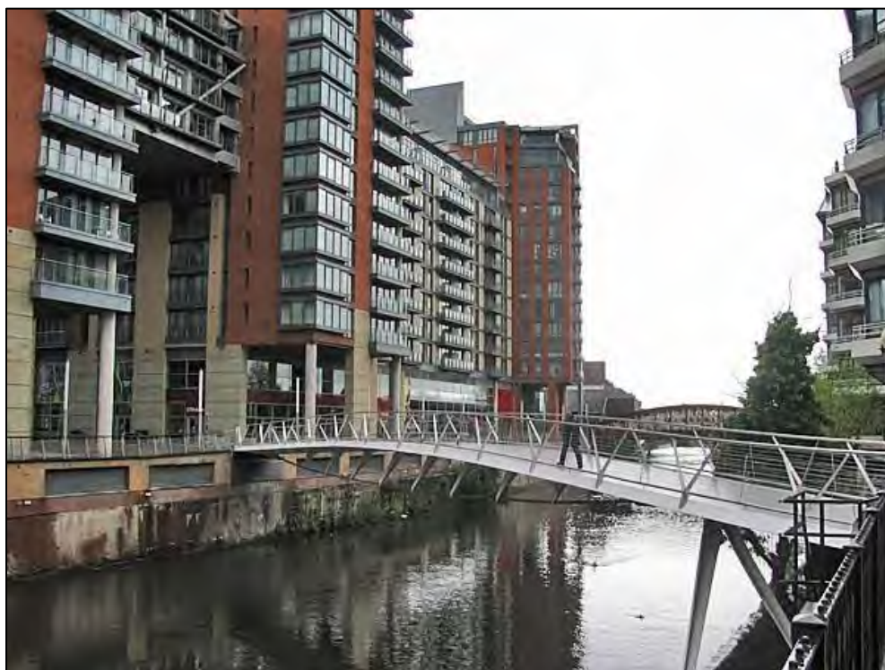
Figure 5.1 Irwell Pedestrian Footbridge
