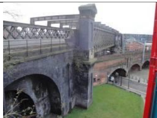
Figure 26: Castlefield Viaduct as it appears in Castlefield; the structure dominates the character of the area.
