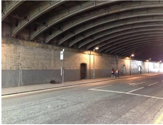
Figure 10: Looking east beneath the viaduct, showing the original glazed brick walls and cast iron roof structure along the northern side of the street.
