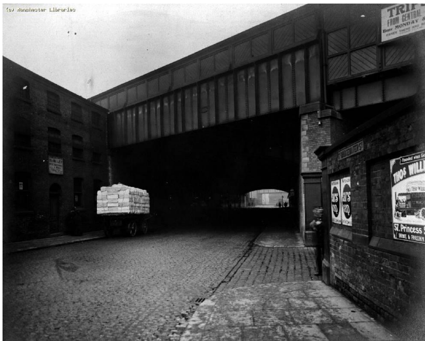
Figure 15: 1909 – A closer view of the eastern end of the bridge/viaduct seen from Great Bridgewater Viaduct as seen in 1909 following the addition of a further railway line, which can be seen running horizontally across the image on extended brick piers.
