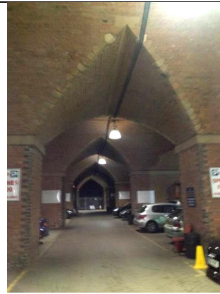
Figure 28: View of the brick undercroft of Castlefield viaduct
