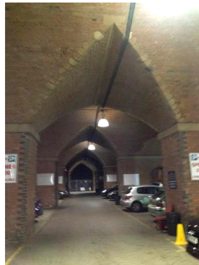
Figure 13: A view looking into the brick vaulted undercroft, now used as car parking.
