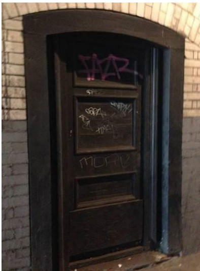
Figure 12: An example of an original doorway into the arched undercrofts from Great Bridgewater Street.
