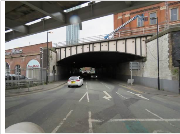
Figure 27: View of Castlefield Viaduct at its crossing with Great Bridgewater Street
