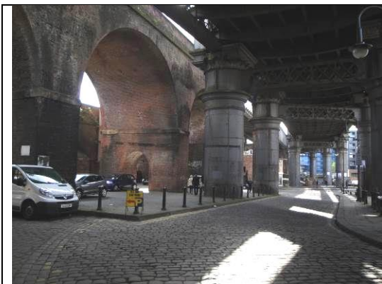
Figure 25: Castlefield Viaduct as it appears within Castlefield; the structure splits in two at this point. This is where the
