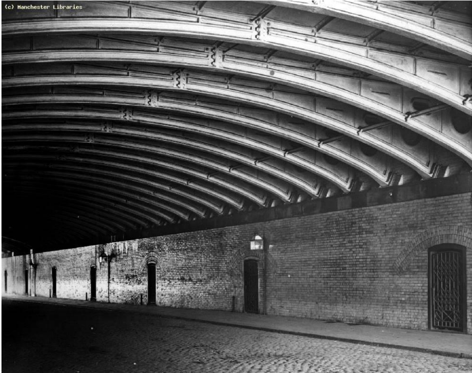
Figure 18: The south side of Great Bridgewater Street, beneath the 1870s viaduct as seen in 1905, showing the original cast-iron roof structure and white glazed brick walls, which remain largely unaltered.
