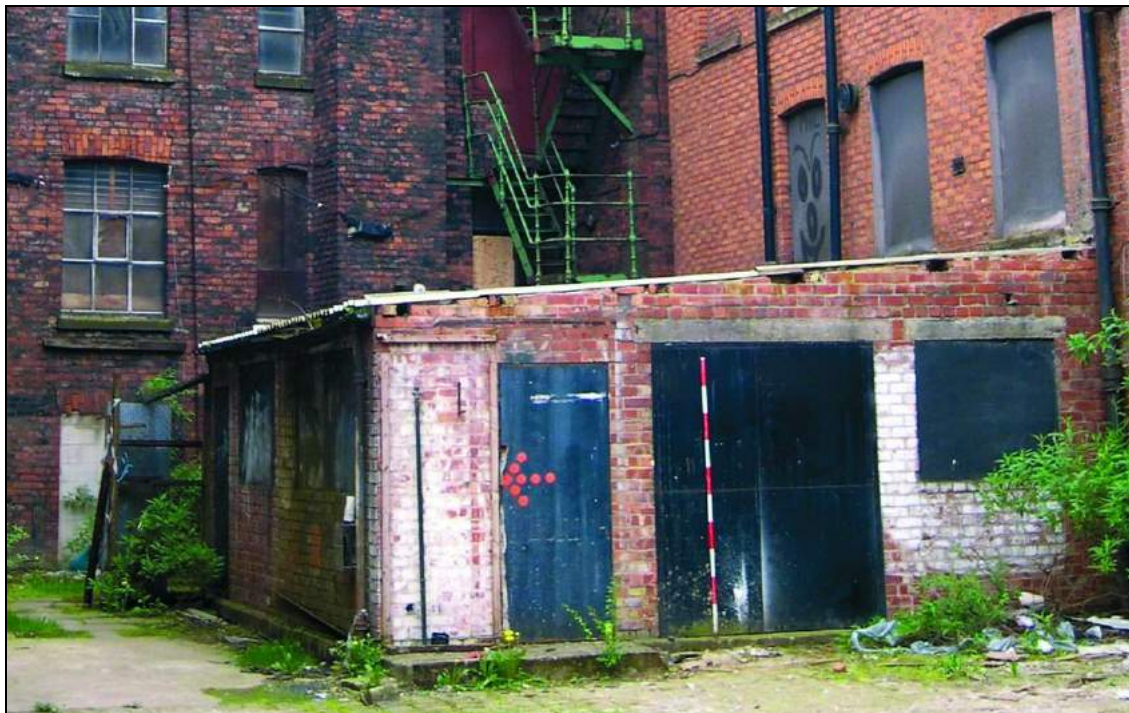
Plate 57: Single-storey shed prior to demolition in 2005
