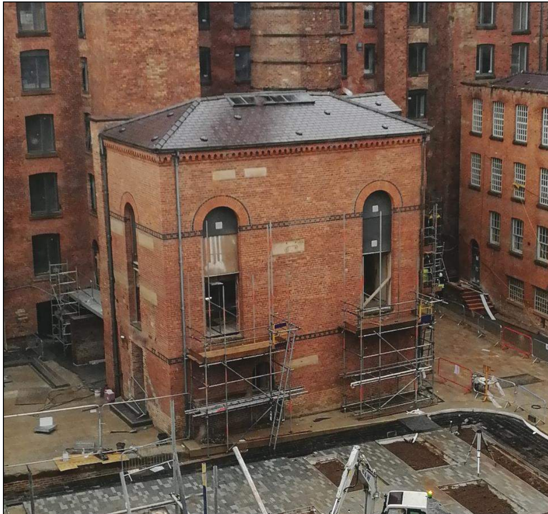
Plate 29: Old and Decker Mill Engine House during refurbishment works
