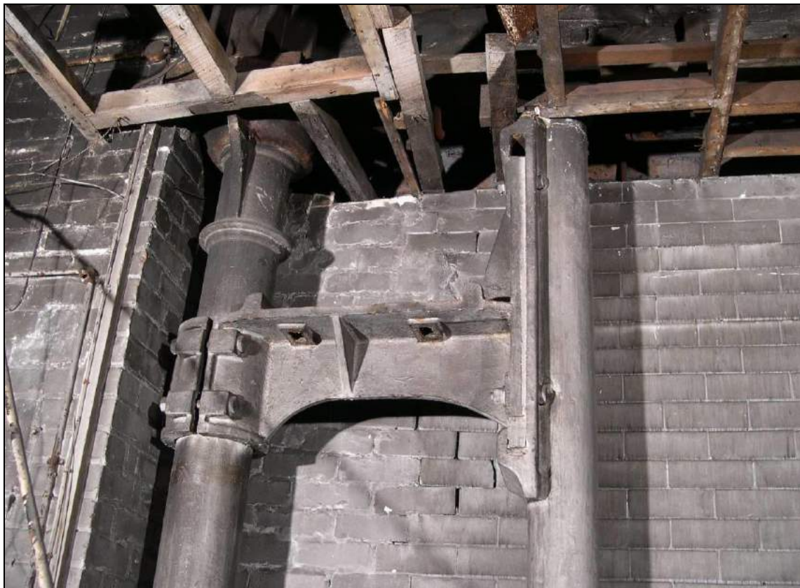
Plate 43: Additional column and carrier beam, New Mill basement, Bay 21
