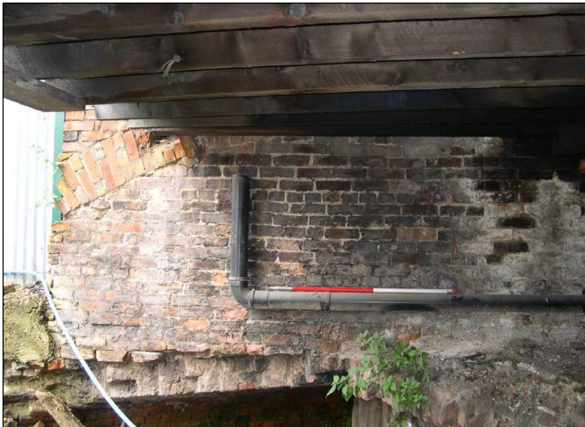
Plate 61: The relieving arch above the canal tunnel
