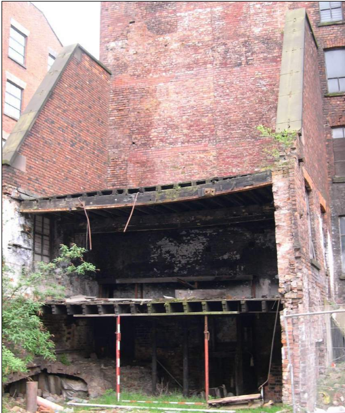
Plate 77: The last surviving two bays of the Bengal Street Block and later buttresses to Decker Mill
