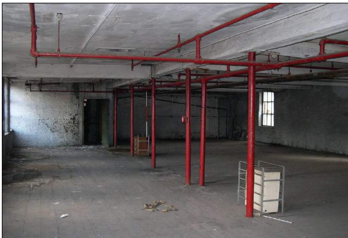
Plate 54: Replaced cylindrical columns, second floor of the Murray Street Block
