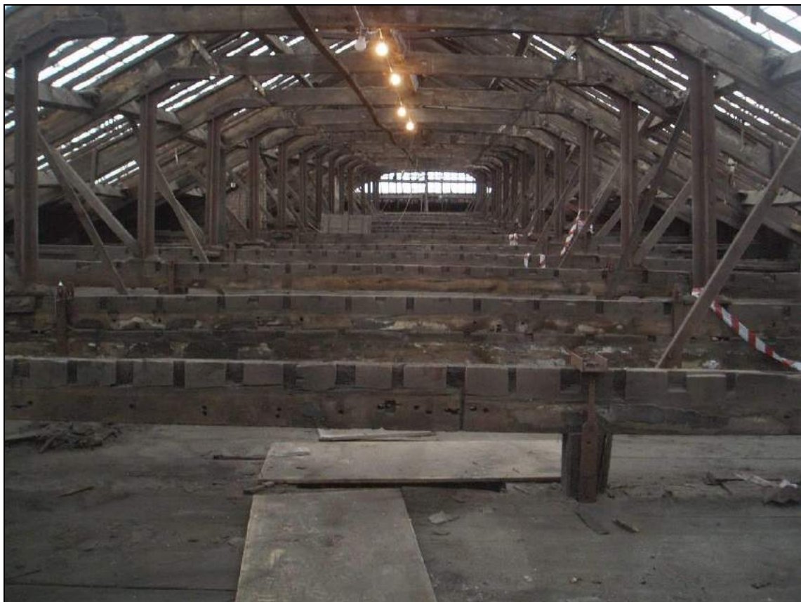
Plate 45: Cruciform-section queen struts
