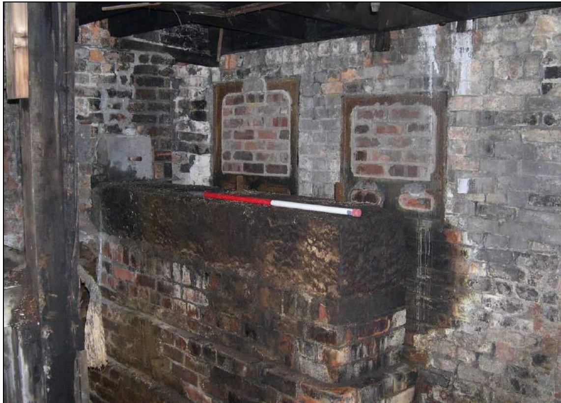
Plate 74: Pier for driveshaft housing, lower ground floor of the Bengal Street Block
