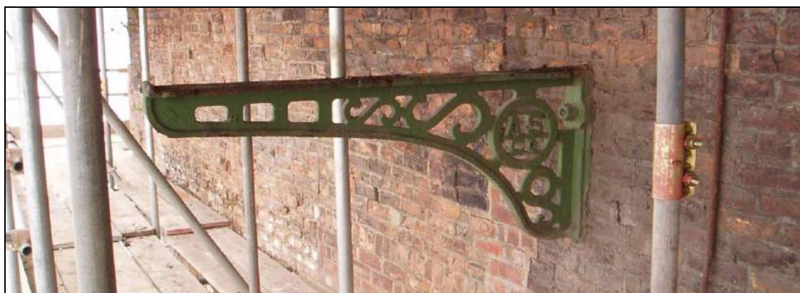
Plate 44: Detail of fire escape corbel
