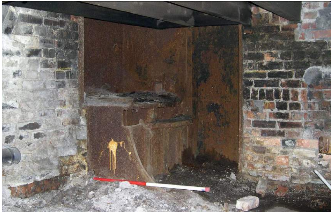
Plate 73: Cast-iron bearing box on the lower ground floor of the Bengal Street Block
