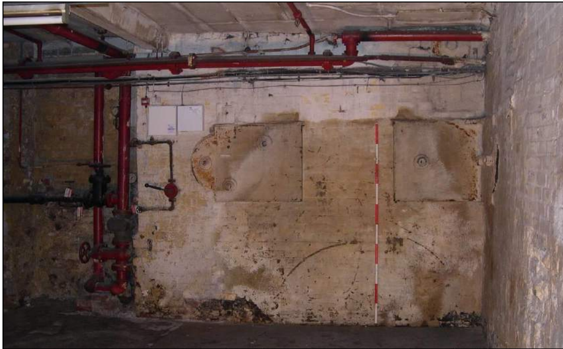
Plate 27: Large plates associated with Phase 5 engine in the basement of Old Mill
