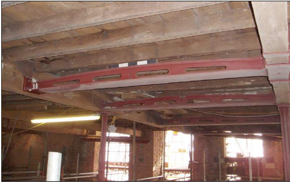
Plate 41: Open-web carrier beam, fourth floor, Bay 17
