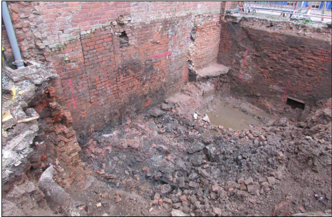
Plate 84: The remains of the late 19 th -century engine foundations removed fully
