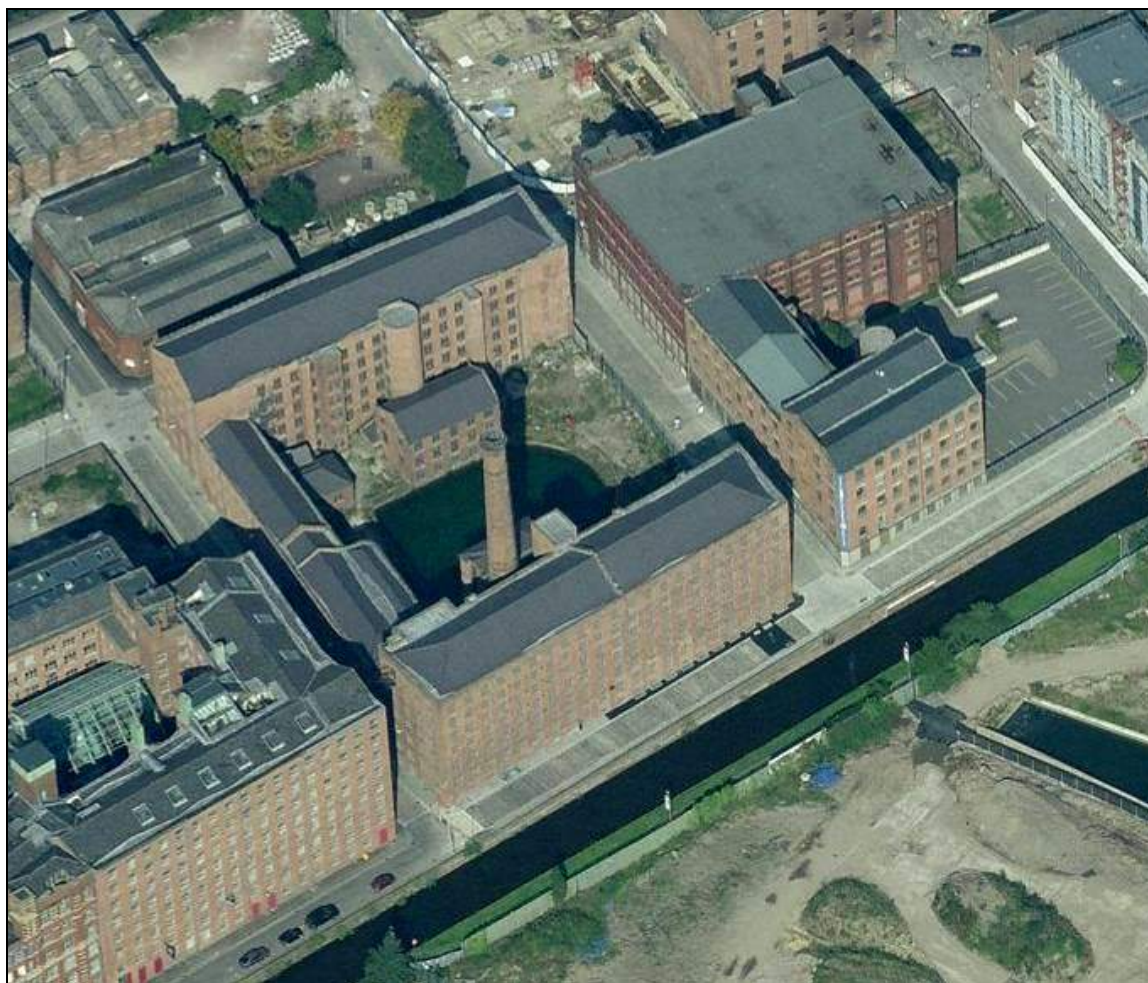
Plate 1: Aerial view across Murrays' Mills following the completion of the Shell Repair Project in 2007
