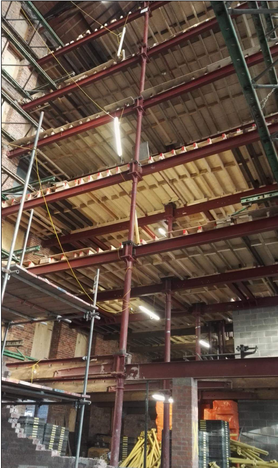
Plate 28: Section through Decker Mill necessitated to enable the removal of the lift shaft in 2017
