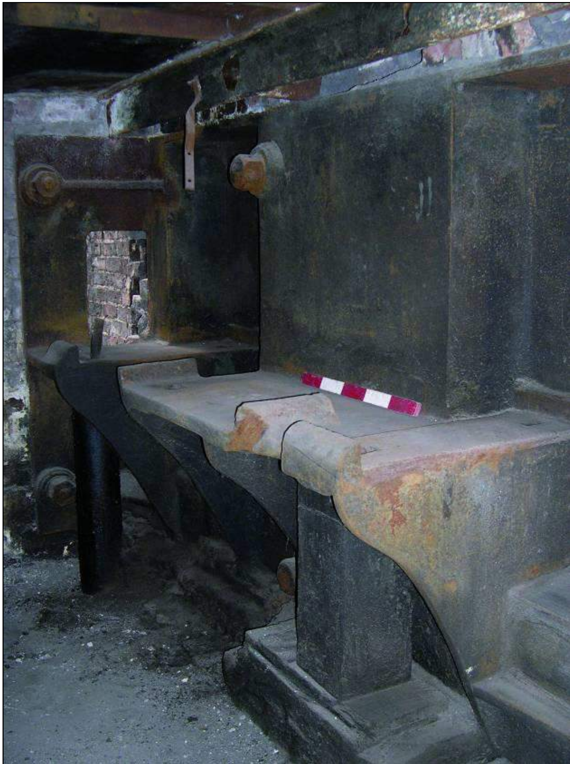
Plate 26: Huge casting for the power-transmission system installed at the base of the Old and Decker Mill stair tower
