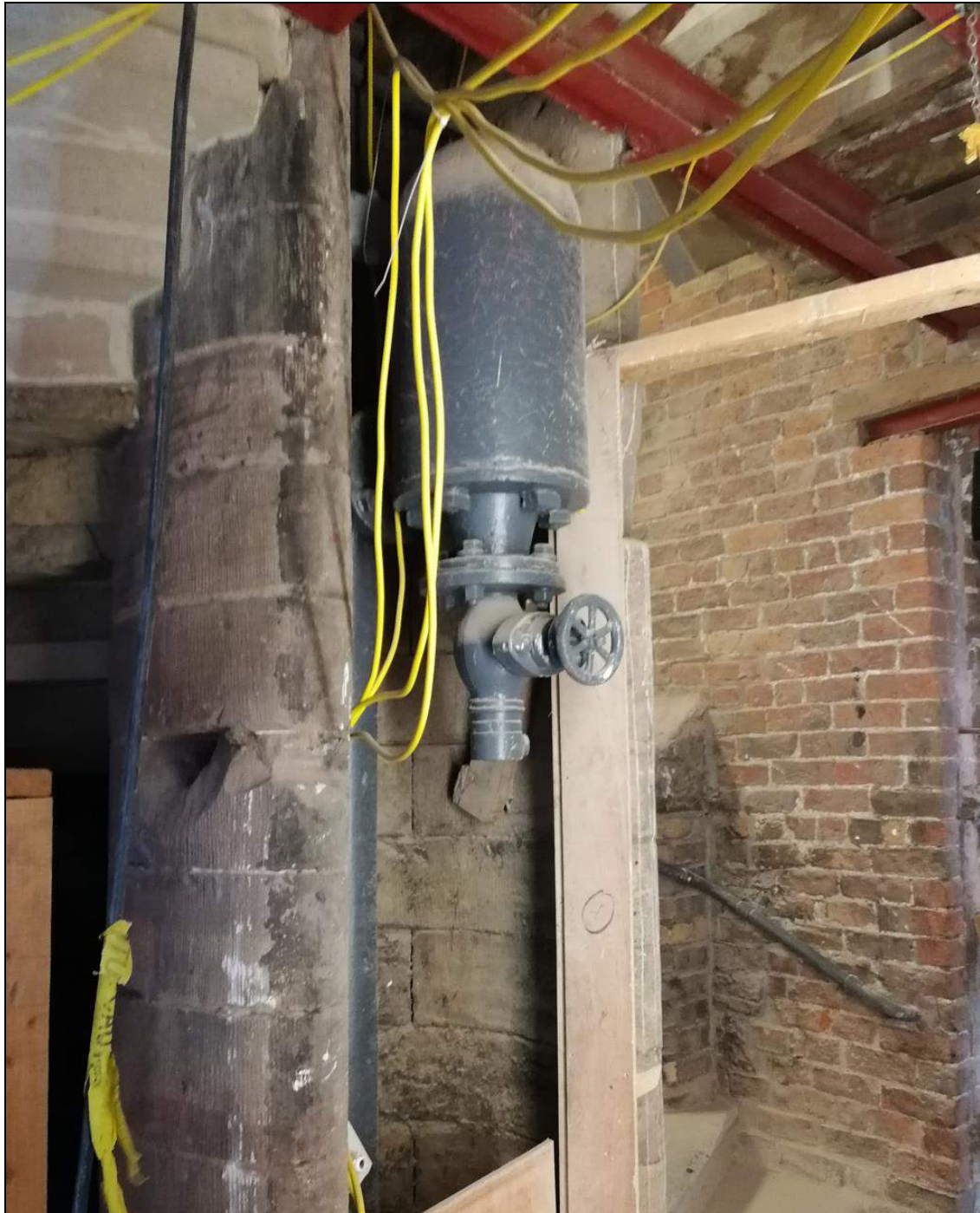
Plate 20: The fire-fighting cistern at the base of Old and Decker mills stair tower
