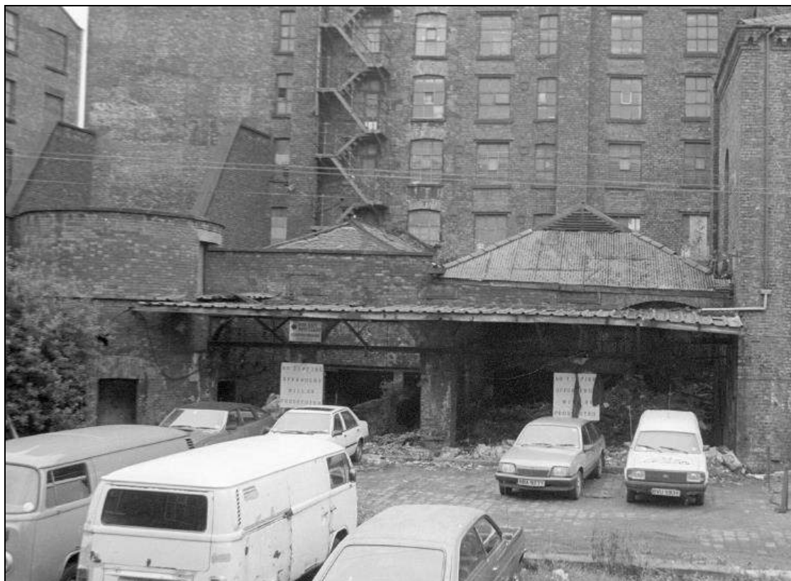
Plate 34: Photograph of the boiler house taken in 1985
