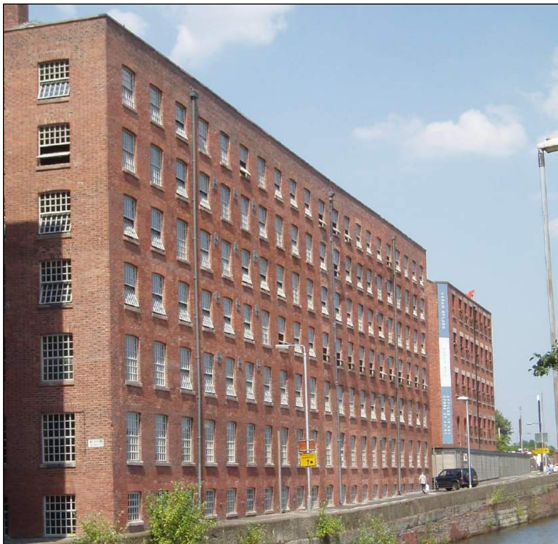
Plate 13: View of Old and Decker Mill, overlooking the Rochdale Canal
