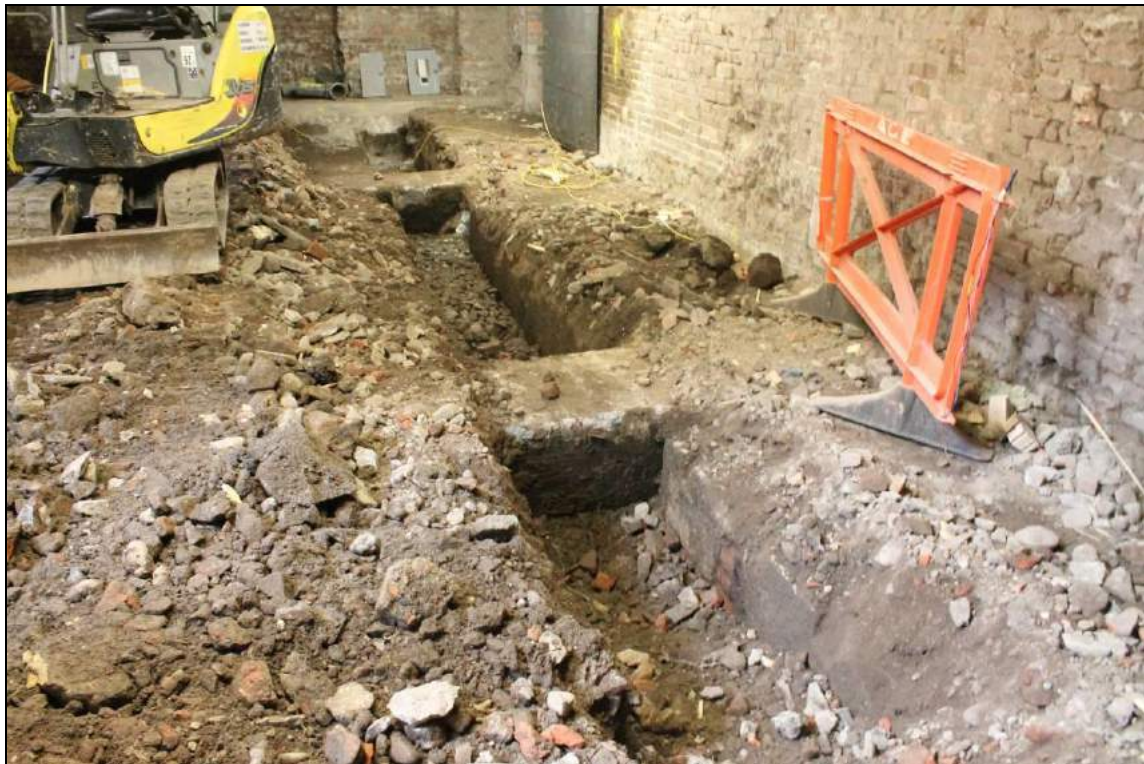
Plate 47: The engine foundation beds exposed in New Mill Engine House
