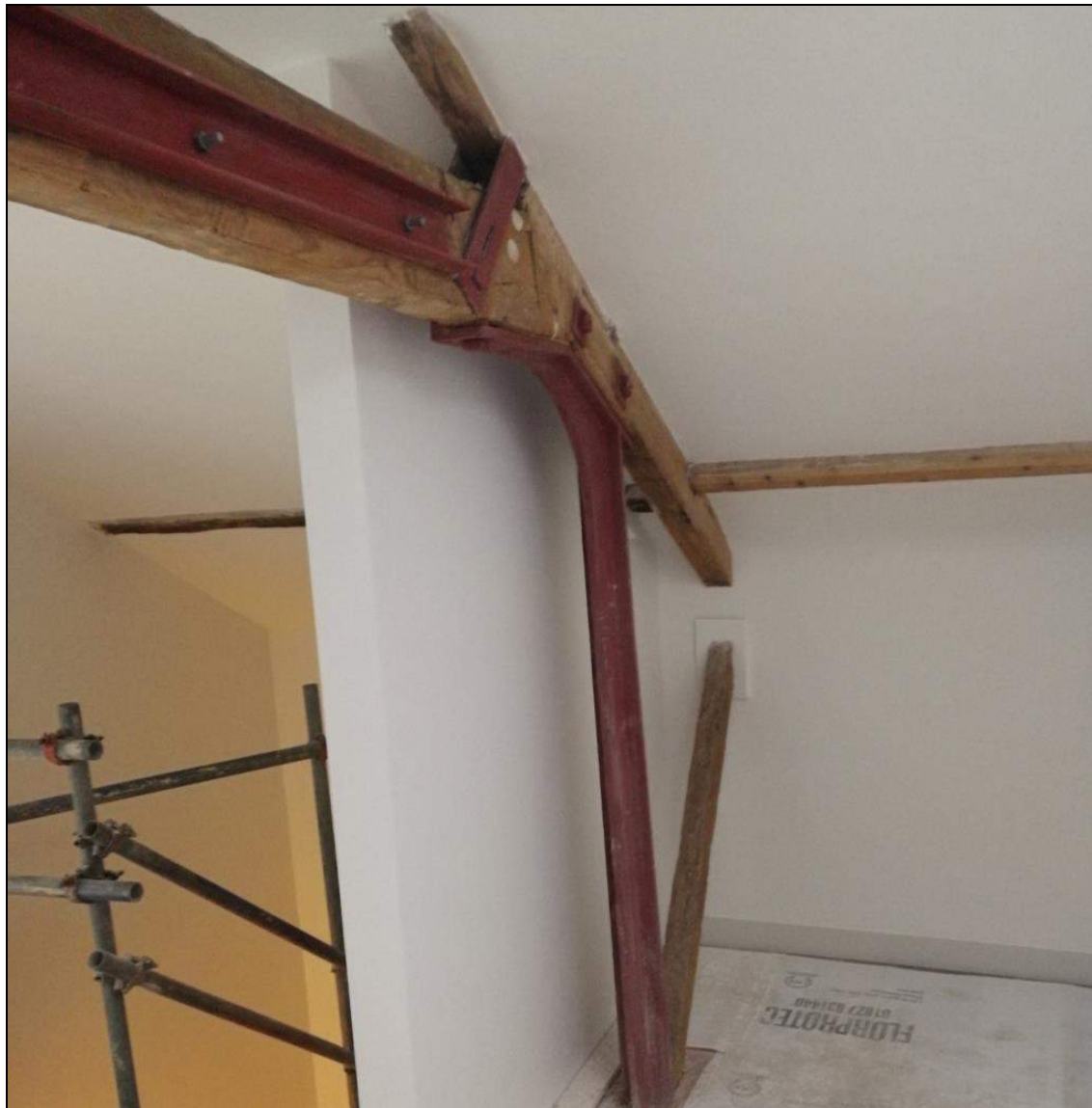
Plate 38: One of the queen struts incorporated into an apartment in the roof space of New Mill
