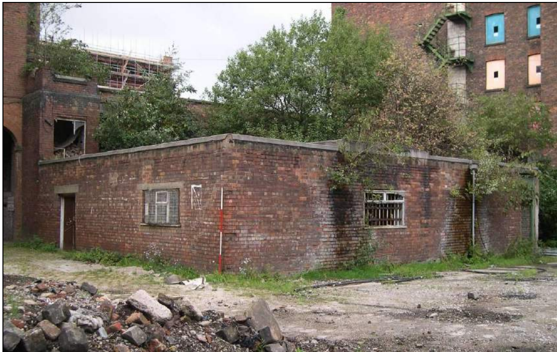
Plate 56: The putative air-raid shelter prior to demolition in 2005
