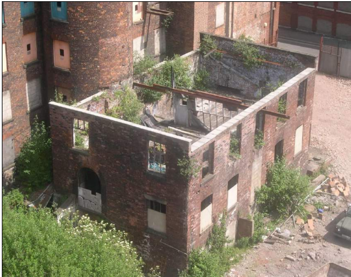
Plate 46: View of the derelict New Mill Engine House in 2004
