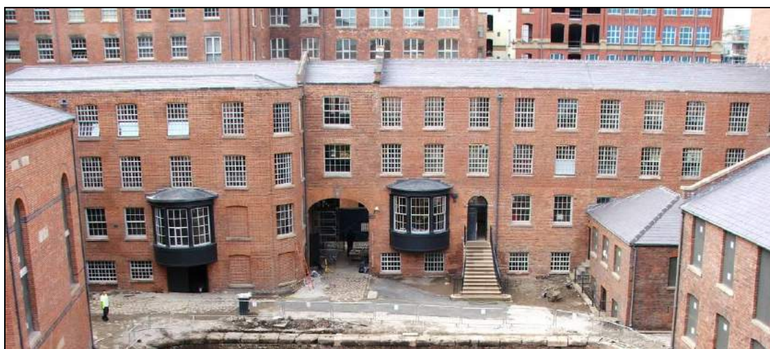
Plate 48: View of the Murray Street Block in 2007, following the reinstatement of the top two storeys
