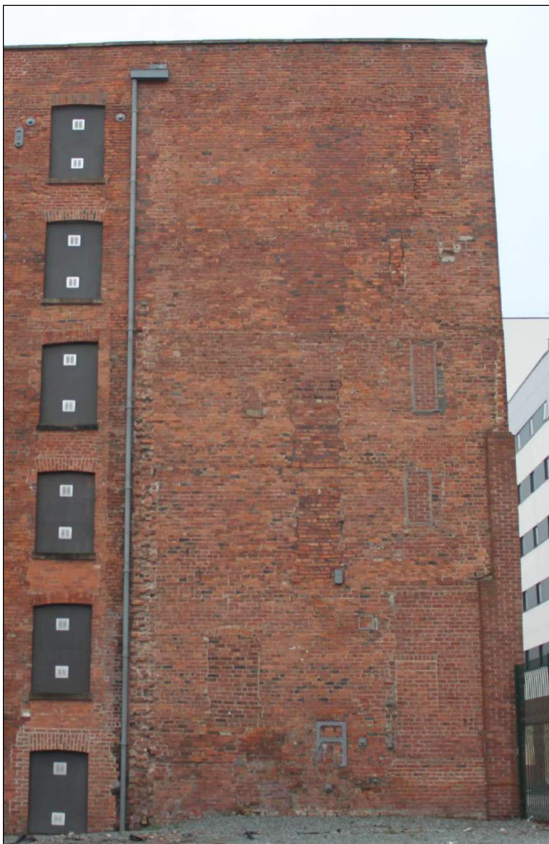
Plate 75: The eastern end of New Mill, showing features pertaining to the former Bengal Street Block
