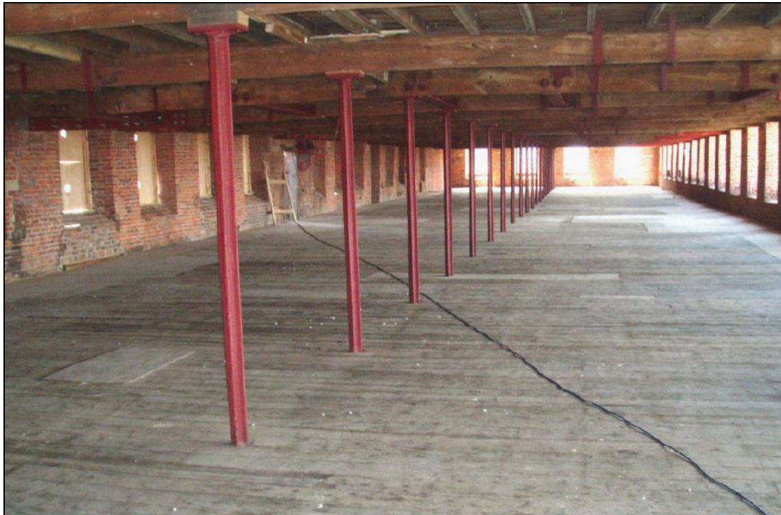
Plate 36: The cruciform columns on the top floor of New Mill prior to repurposing as apartments
