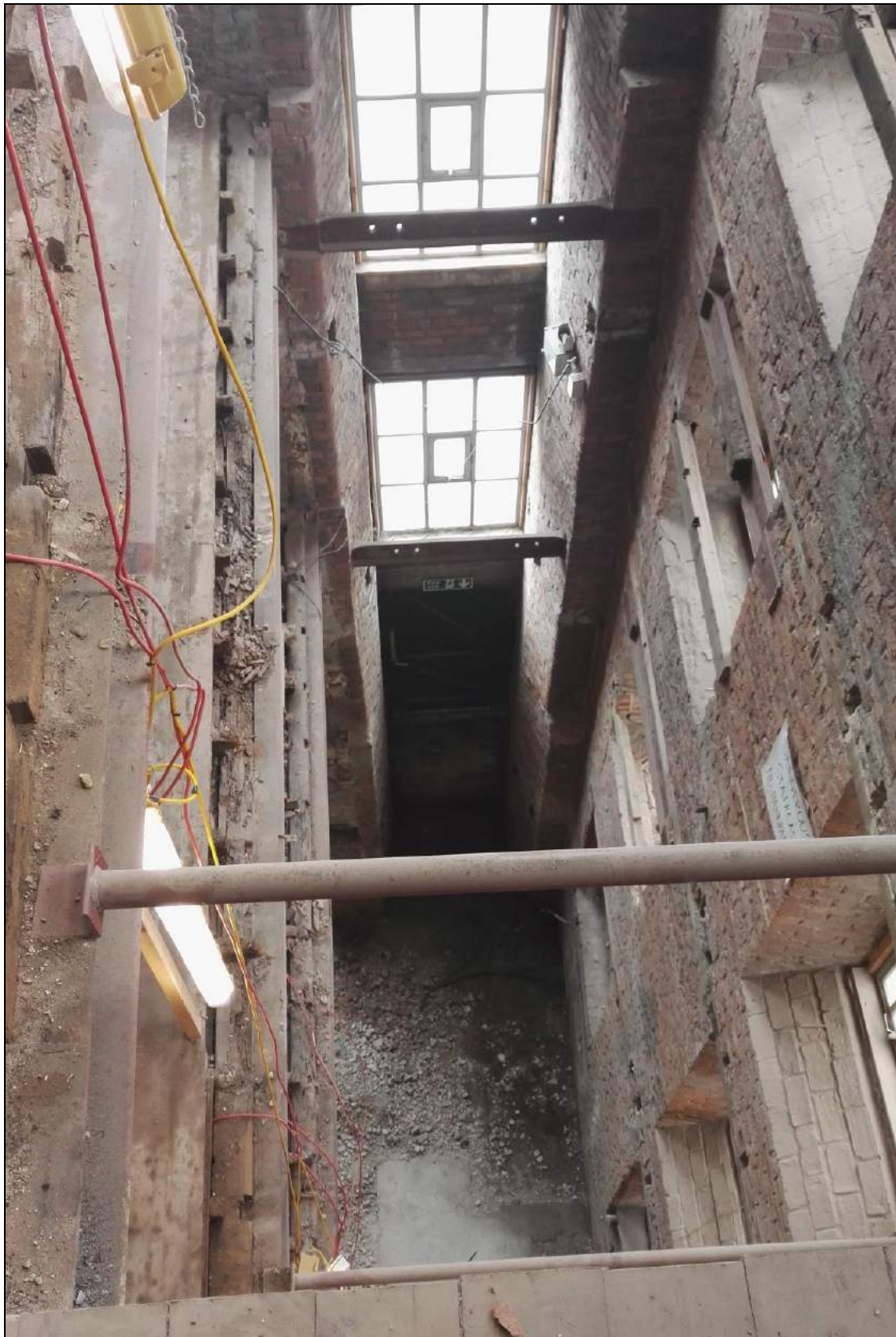
Plate 42: The rope race at the eastern end of New Mill following the removal of the mid-20 th -century stair in 2017
