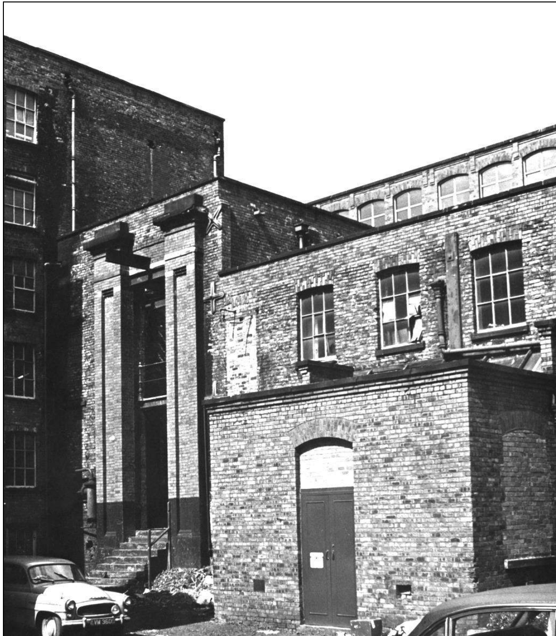
Plate 81: The late 19 th -century engine house and early 20 th -century electric substation at the northern end of the Bengal Street Block in the 1960s
