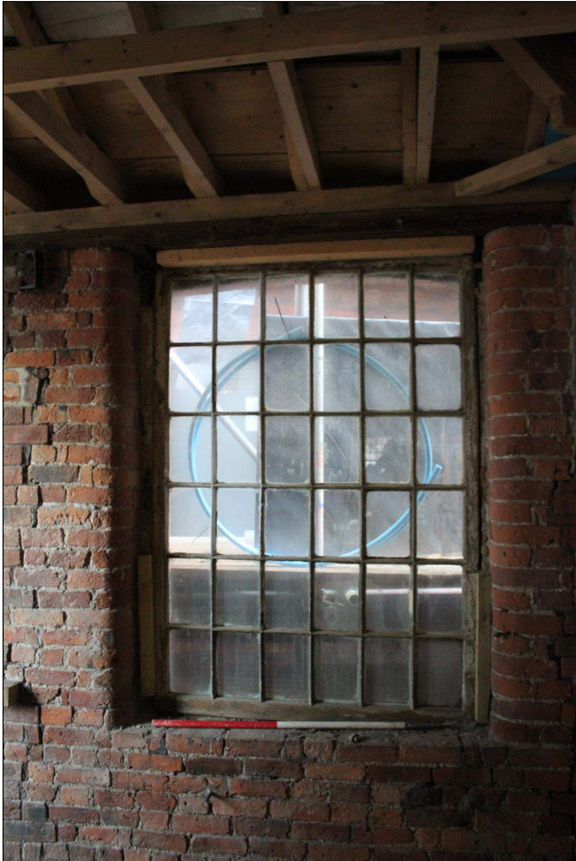
Plate 55: An original window in the Murray Street Block
