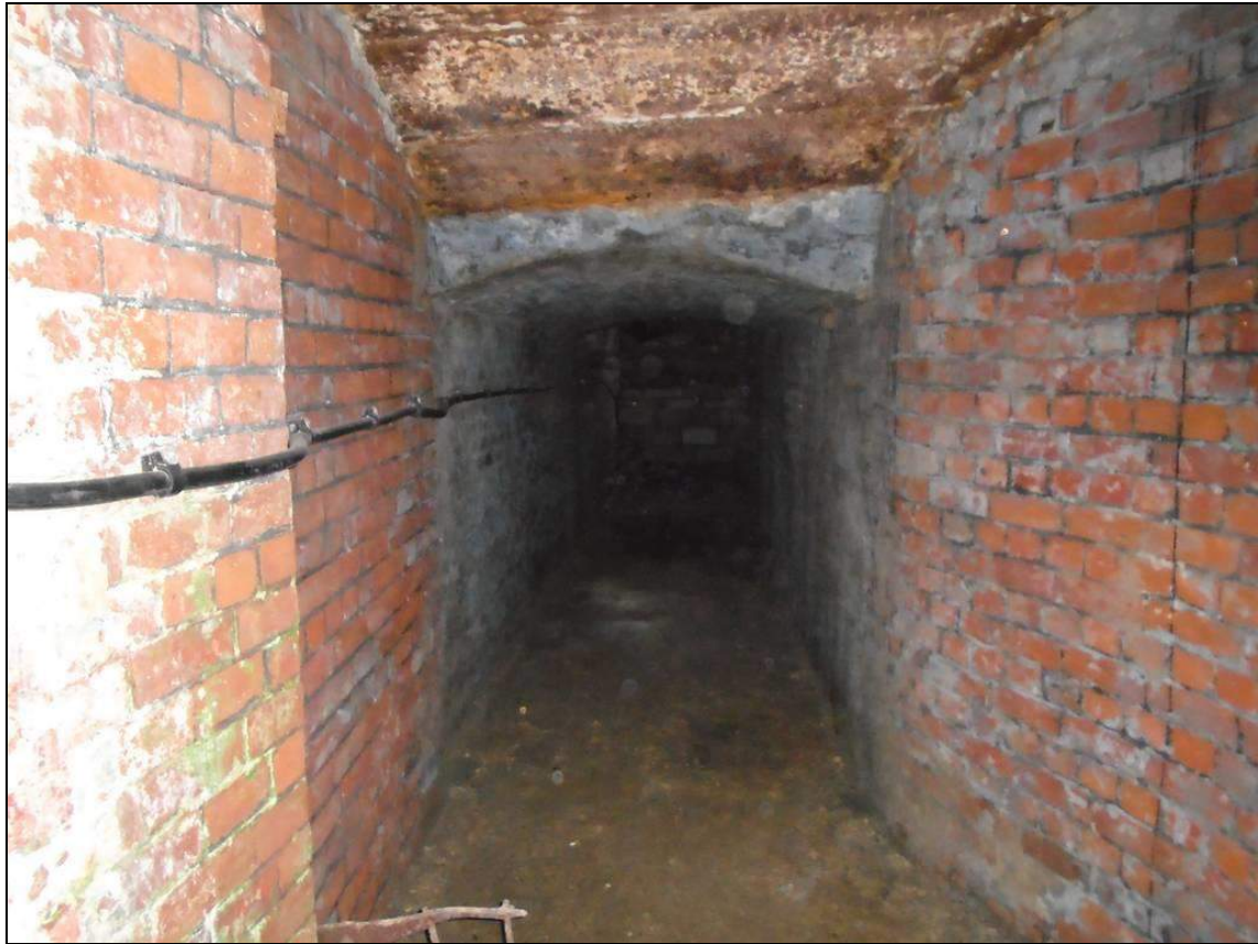
Plate 71: Entrance to the subway from New Little Mill, accessed in 2017
