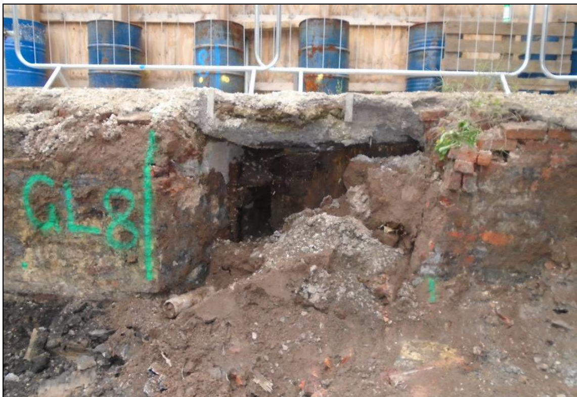
Plate 72: Entrance to the subway from the Bengal Street Block to Fireproof Mill exposed in 2016
