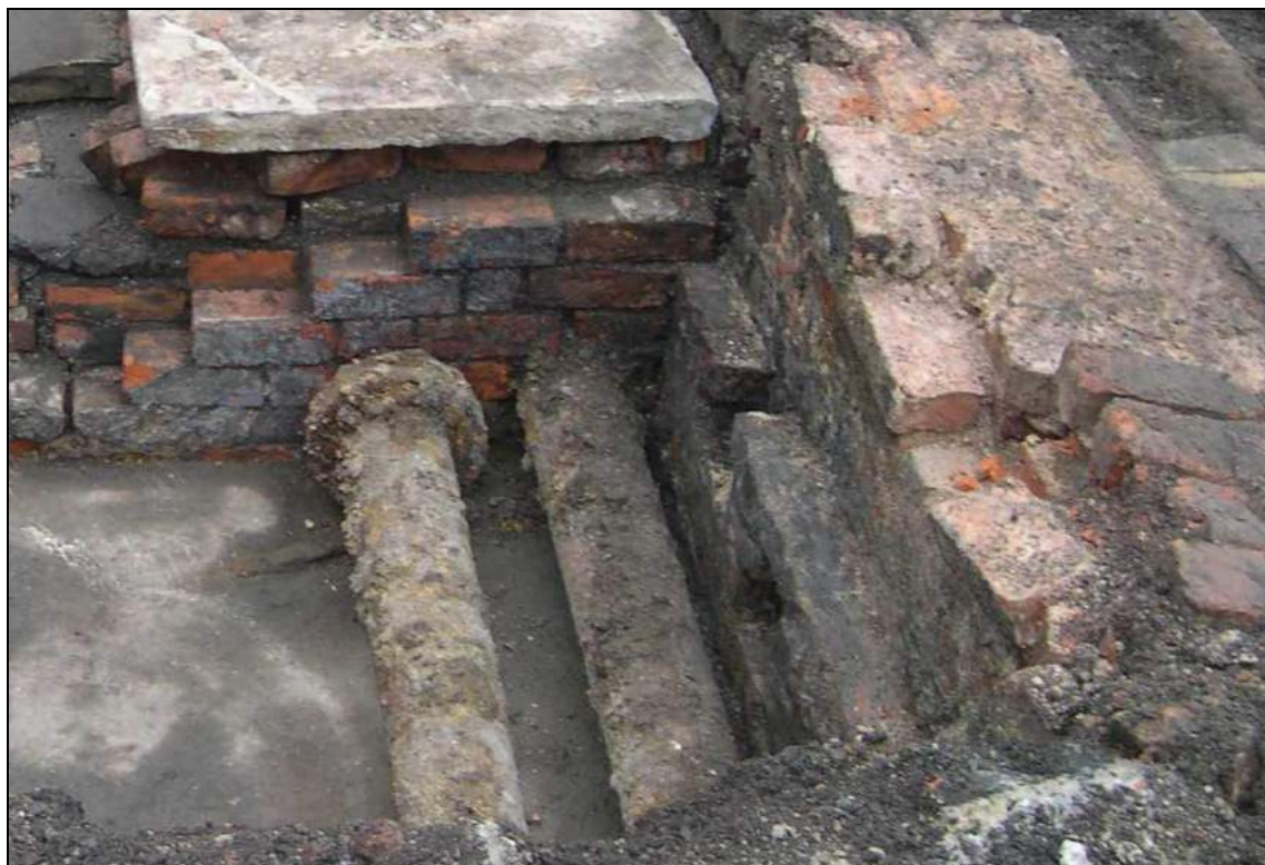
Plate 78: Mather & Platt Ltd sprinkler system pipes adjacent to the west wall of the Bengal Street Block
