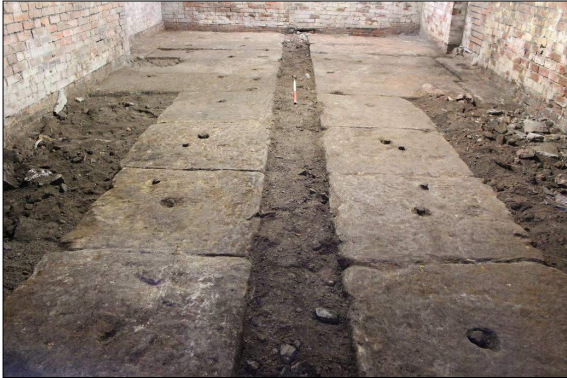
Plate 31: Stone foundation beds for the late 19 th -century engine the powered Old and Decker Mill
