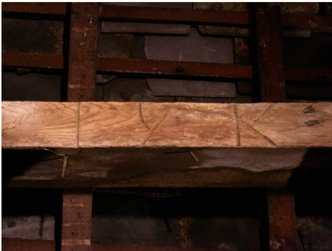
Plate 14: Example of a Baltic timber mark in Old Mill
