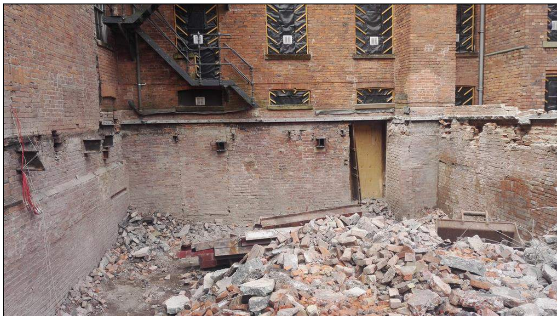
Plate 49: The site of the Blowing Room following demolition in 2016, showing the stubs of the rolled steel joists embedded in the Murray Street Block and New Mill
