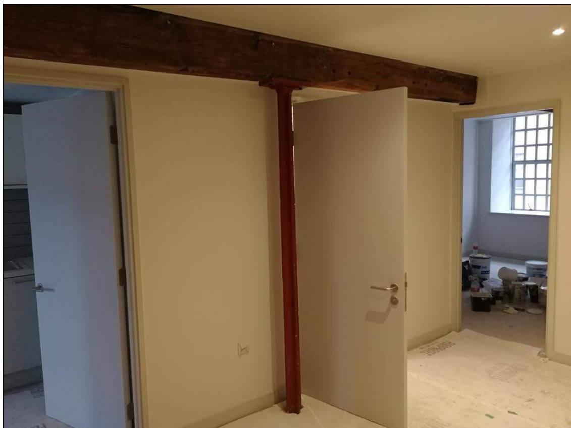
Plate 37: One of the cruciform columns on the top floor of New Mill incorporated into a new apartment
