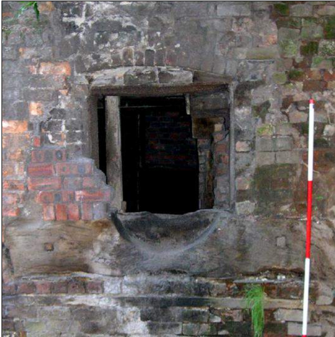
Plate 30: Timber sole plate associated with the Phase 2 power-transmission set into the stair tower
