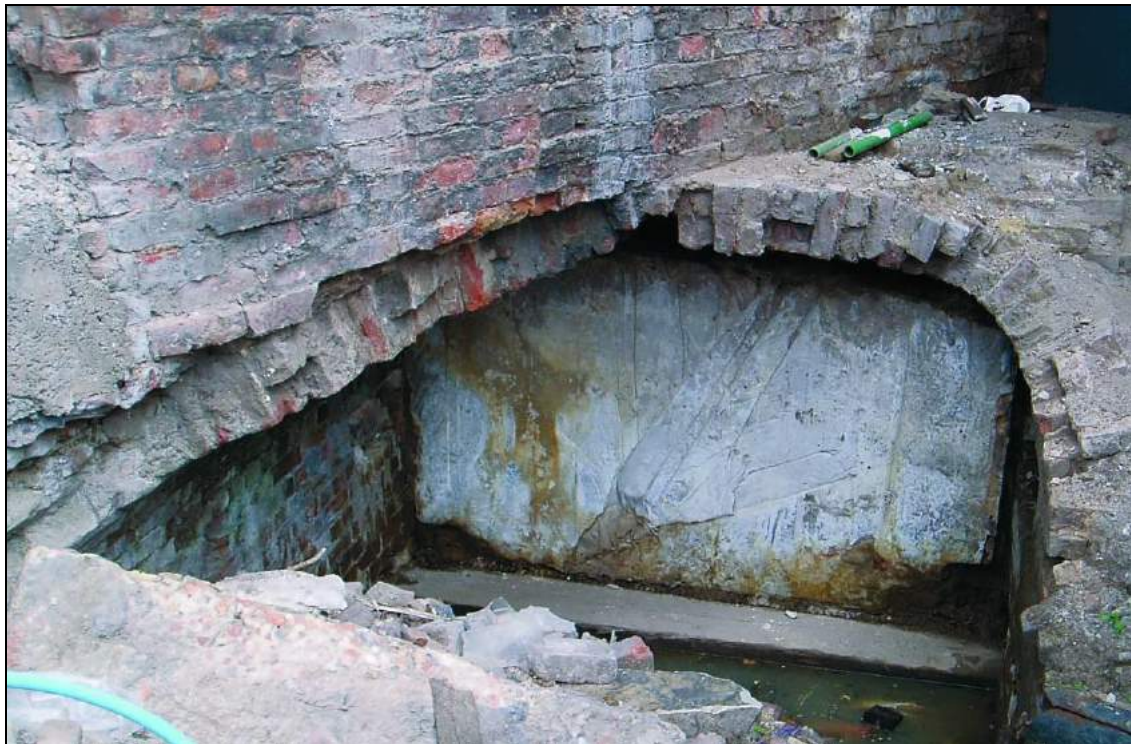
Plate 60: The crown of the canal tunnel beneath the Bengal Street Block, infilled with concrete
