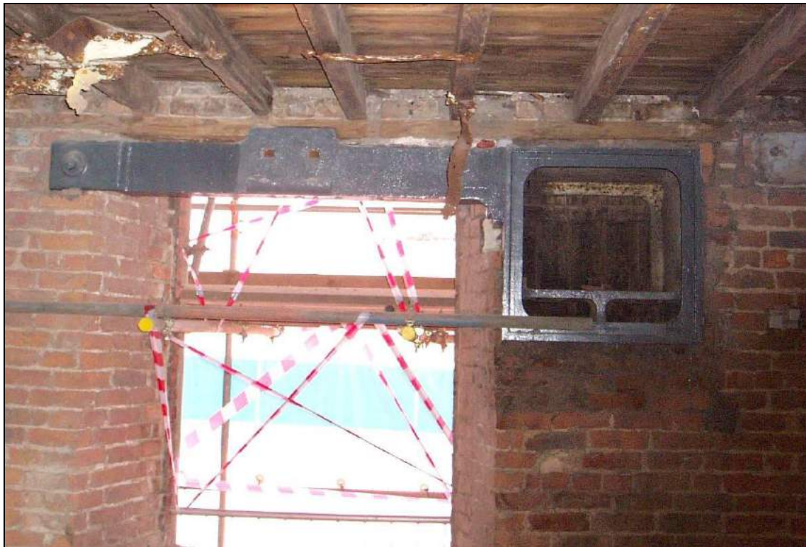
Plate 40: Bearing box for line-shafting associated with Little Mill on the third floor of New Mill
