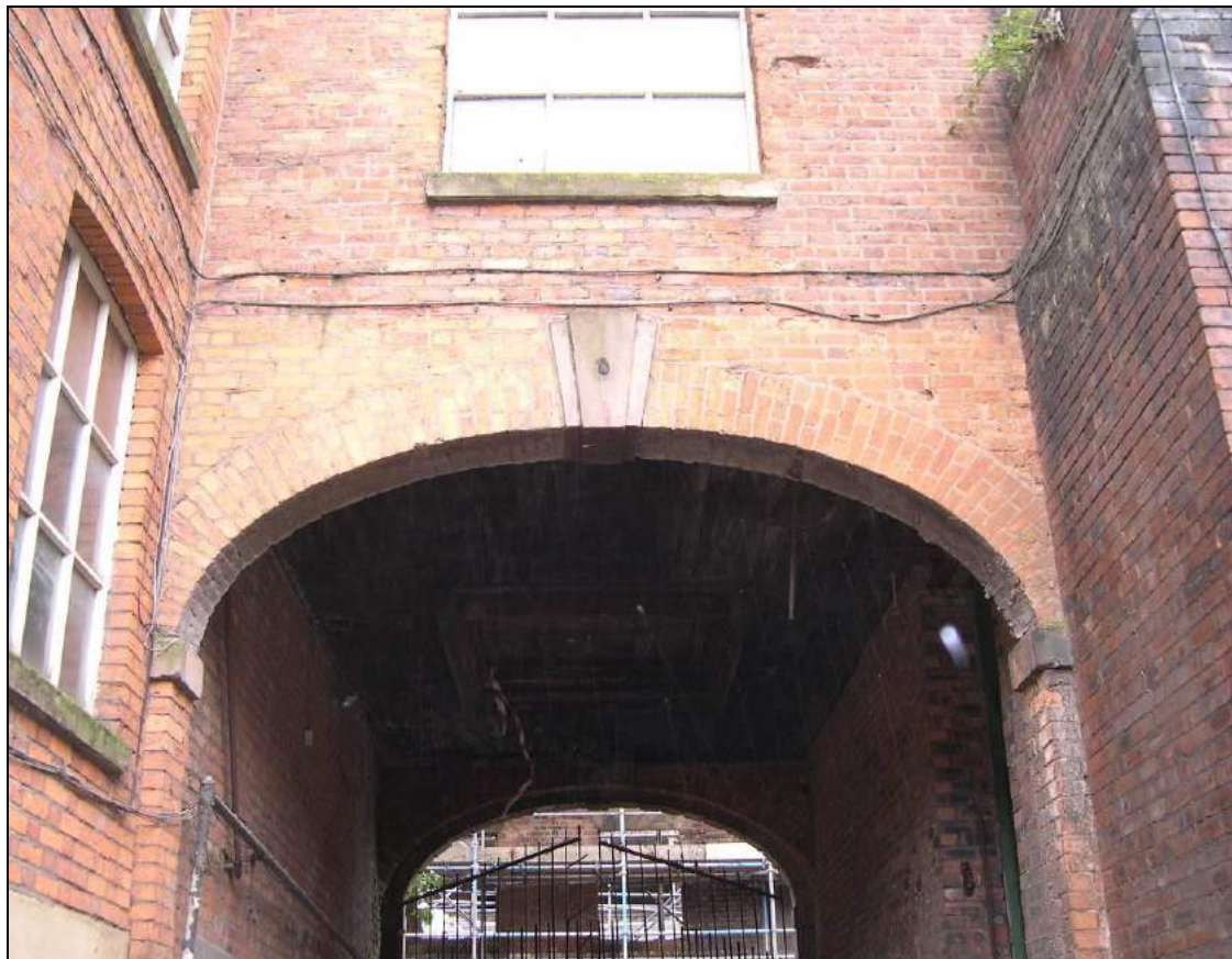
Plate 50: Rebuilt inner arch of the Murray Street Block (Link Block), Bay 10
