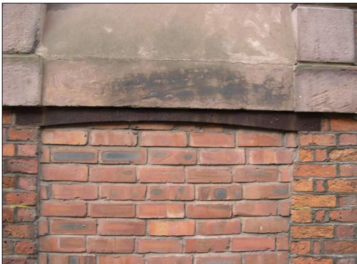
Plate 52: Inserted cast-iron lintel, west external elevation, Bay 7 of the Murray Street Block
