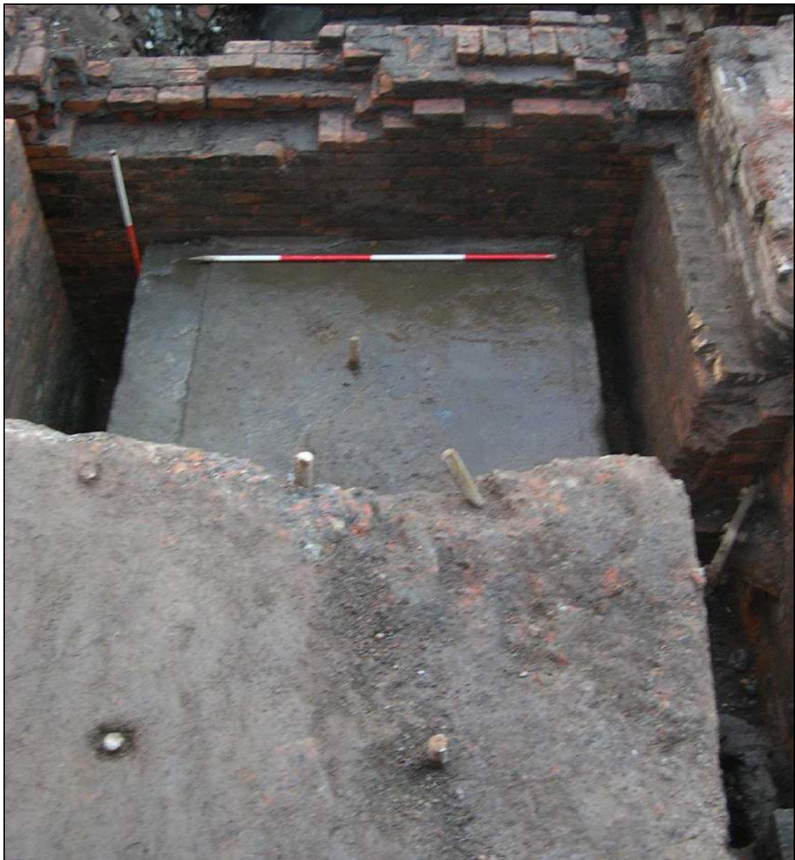
Plate 83: Foundation beds for the late 19 th -century engine
