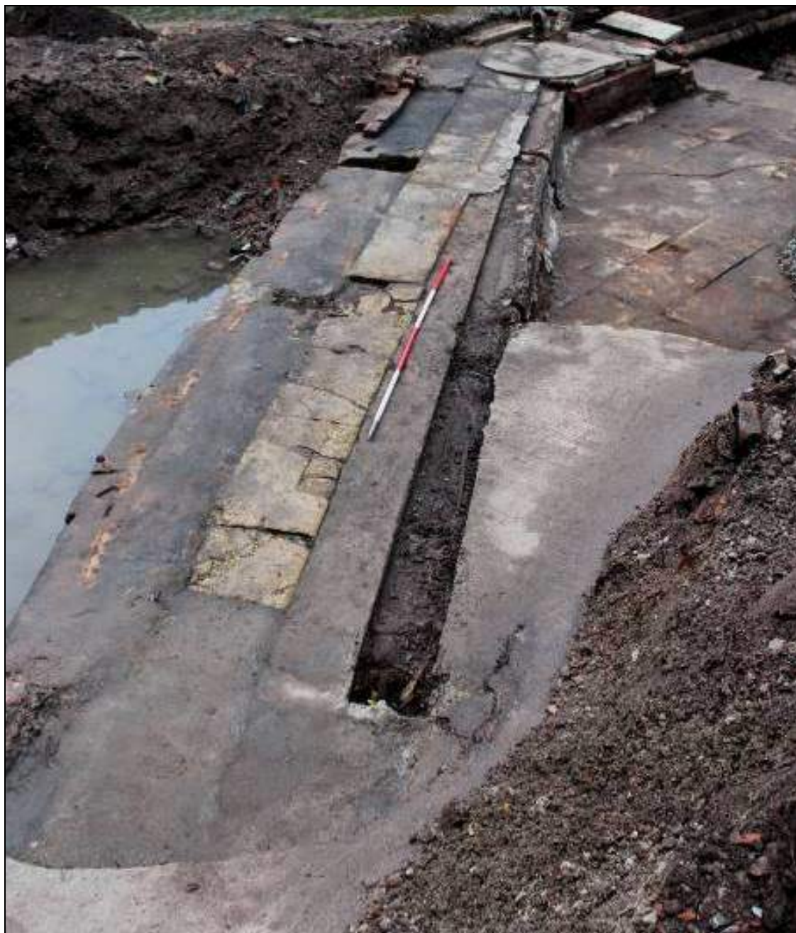
Plate 89: Concrete 'tanking' next to canal wall, looking north-west
