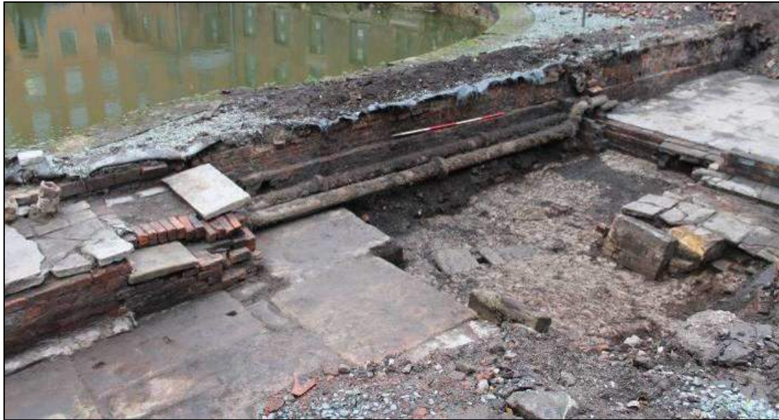
Plate 62: The western exterior wall of the Bengal Street Block excavated in December 2013, showing pipes for the sprinkler system
