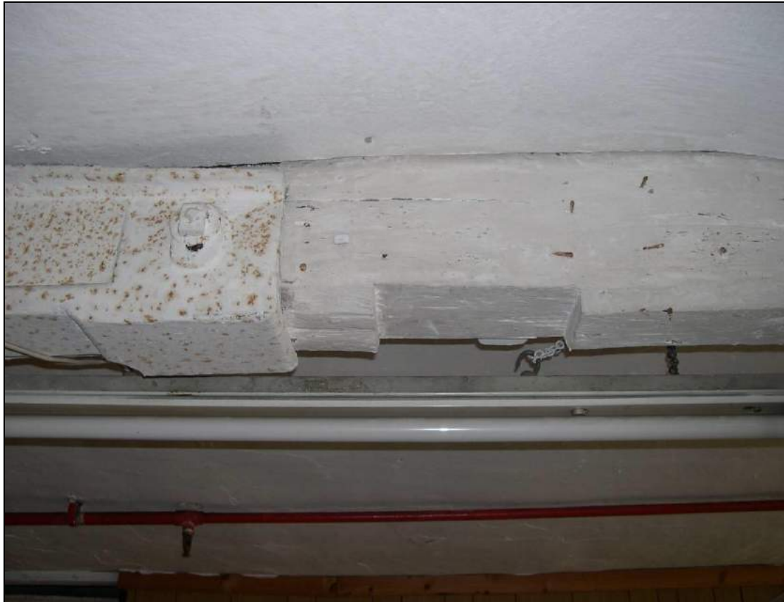
Plate 15: Rebate denoting original column position, second floor, Old Mill
