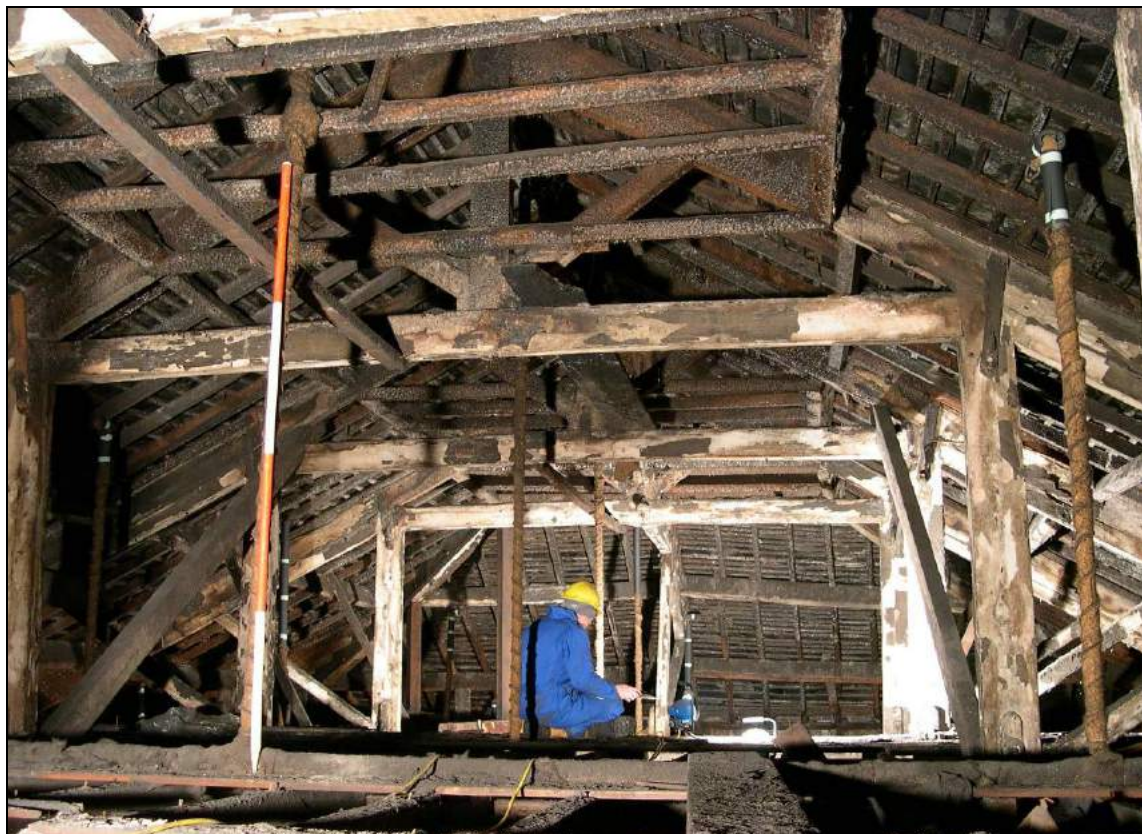
Plate 17: The roof space in Old Mill prior to the refurbishment in 2005
