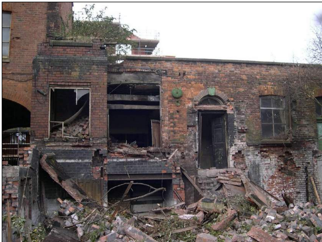
Plate 58: The dilapidated Murray Street North Block in 2005
