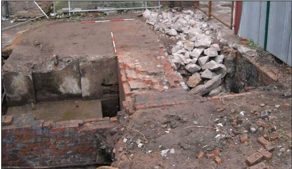
Plate 82: Initial excavation of the engine house at the northern end of the Bengal Street Block
