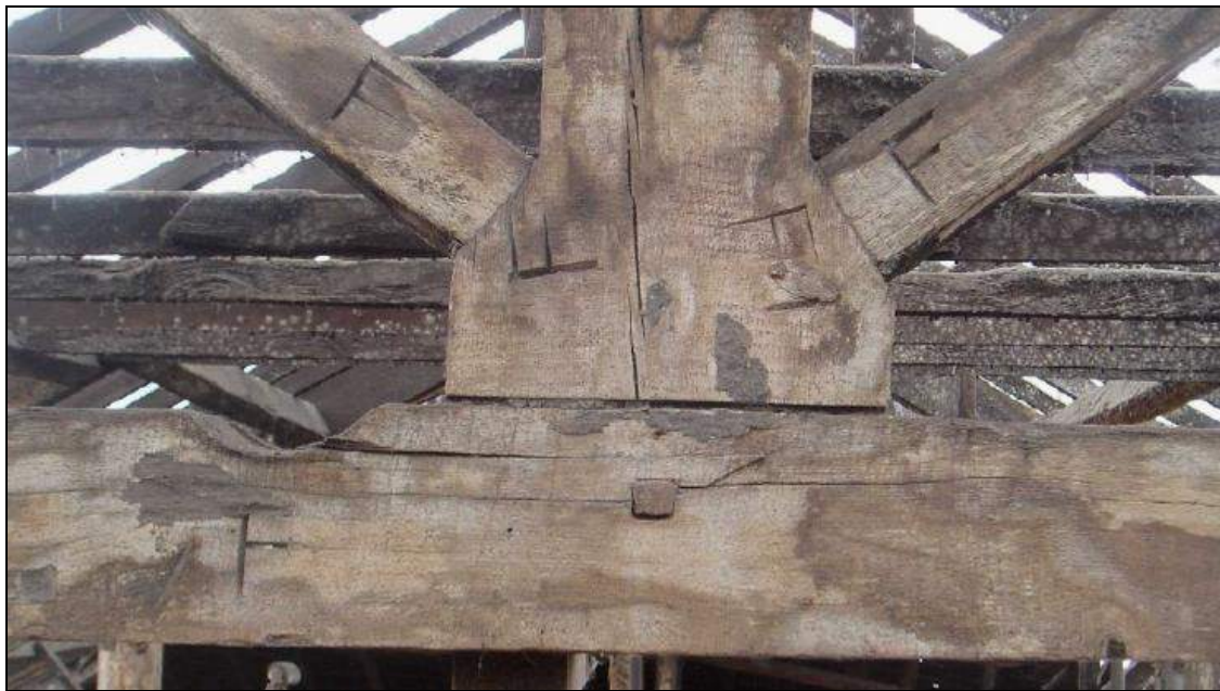
Plate 18: Carpenters' assembly marks in Old Mill roof
