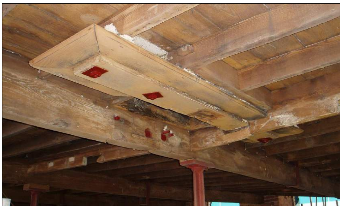
Plate 39: Framing for the vertical transmission on the top floor of New Mill
