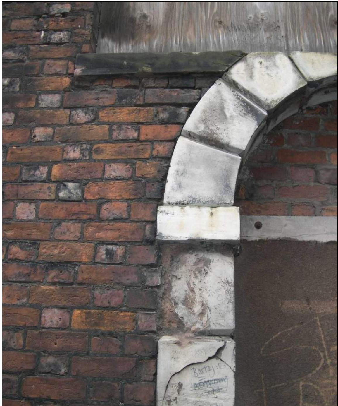
Plate 51: Cut quoin stone of the doorway in Bay 11 of the Murray Street Block
