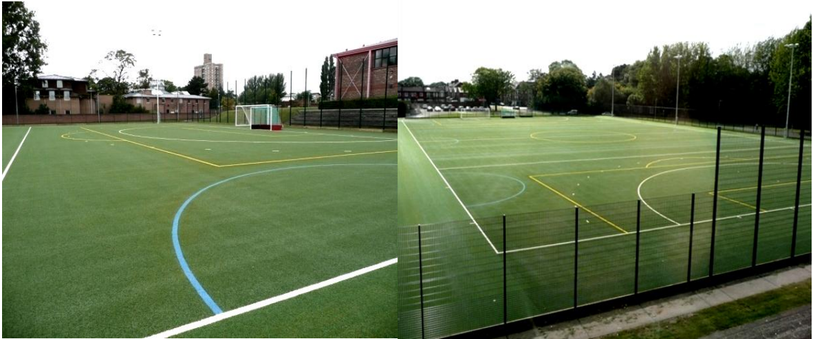
Example of sand dressed artificial turf installed
