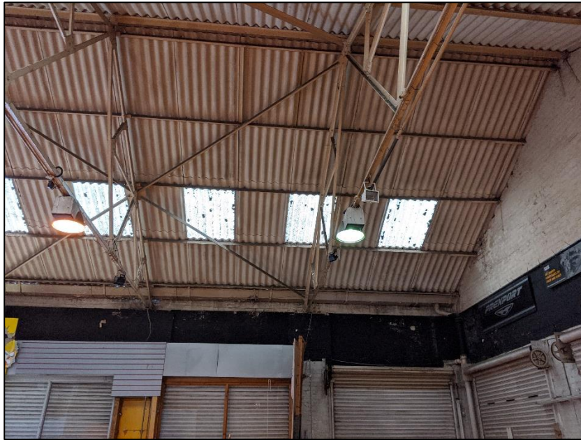
Photograph 5 showing the interior of Building 2
