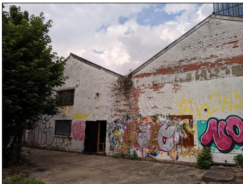
Photograph 4 showing the brickwork on the side elevations
