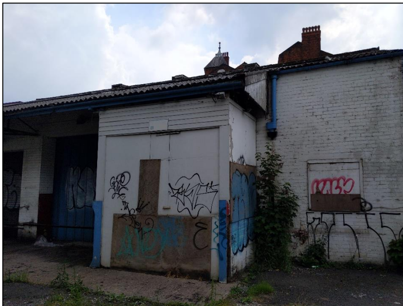
Photograph 1 showing the front elevation of the structure
